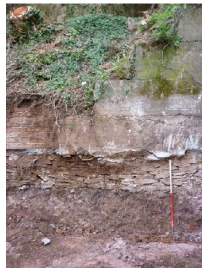
Plate 17 (right): Detail of the dry stone wall below the north-east section of the retaining wall
