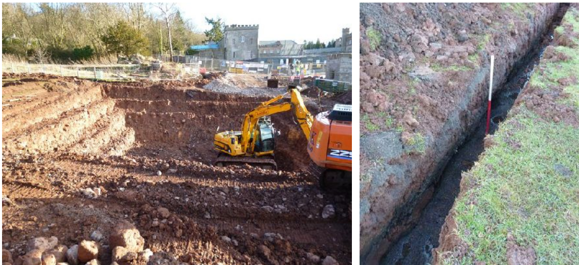
Plate 24 (left): Stepped excavation in Area B
