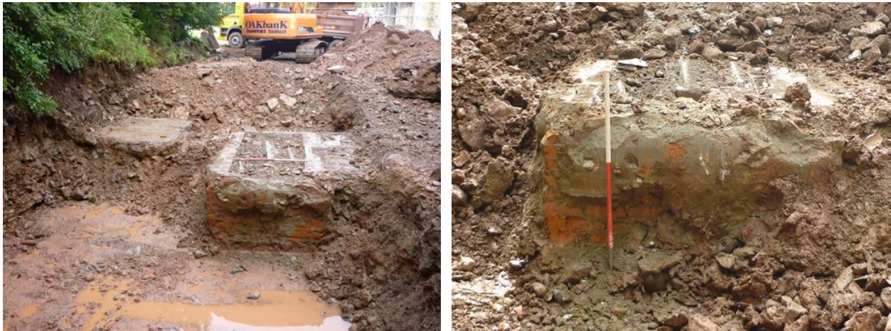
Plate 10 (left): Concrete stanchion (left) and brick-built structure (centre)
