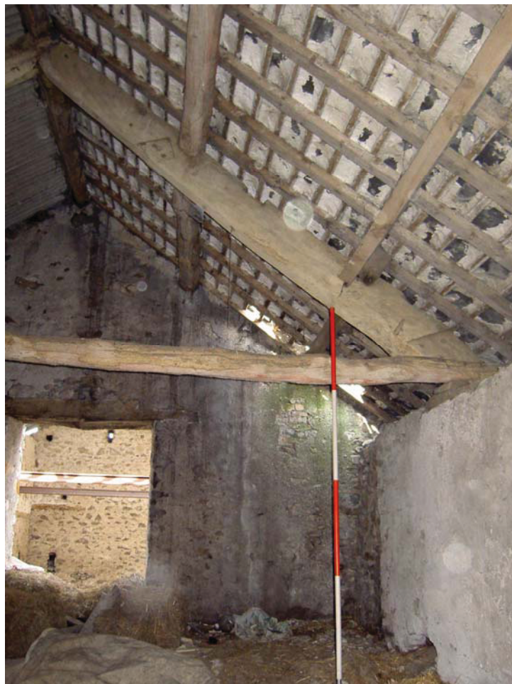
Plate 21: Detail of relict joist slots in truss in first floor Room 2
