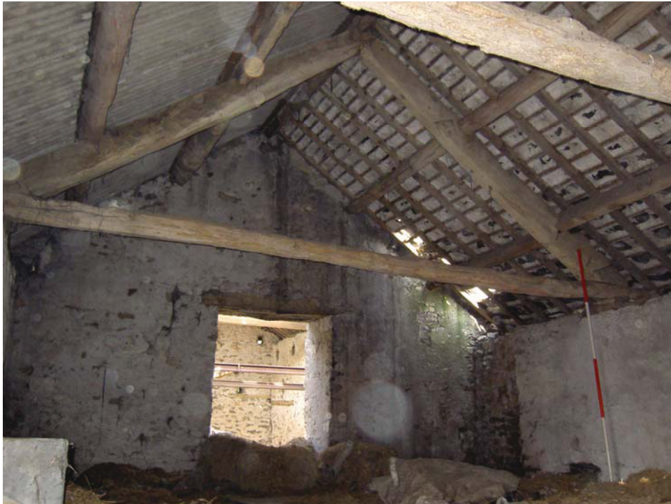
Plate 20: Truss in first floor Room 2
