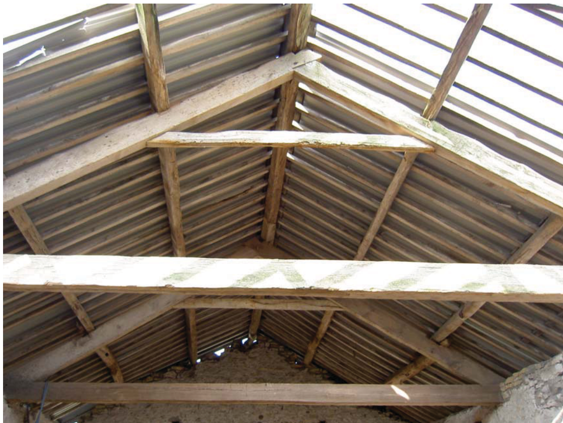
Plate 10: Truss within the threshing barn (Room 1)
