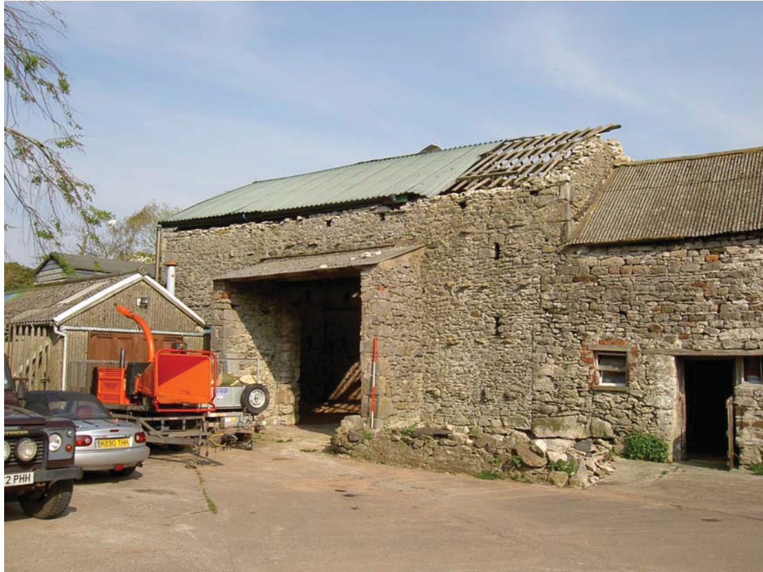
Plate 9: The north-east end of the north-west external elevation
