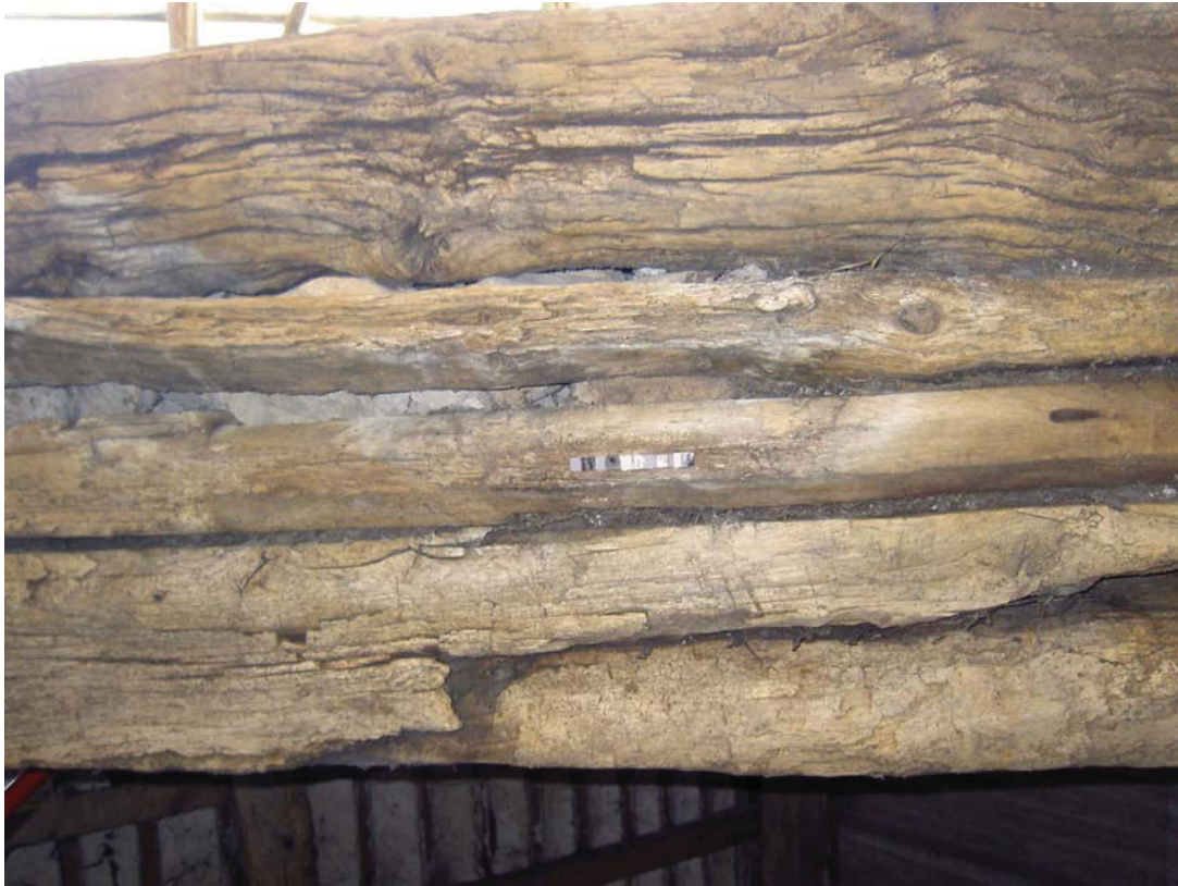
Plate 14: Re-used bedpost (?) used as a lintel in the doorway between first floor Rooms 1 and 2
