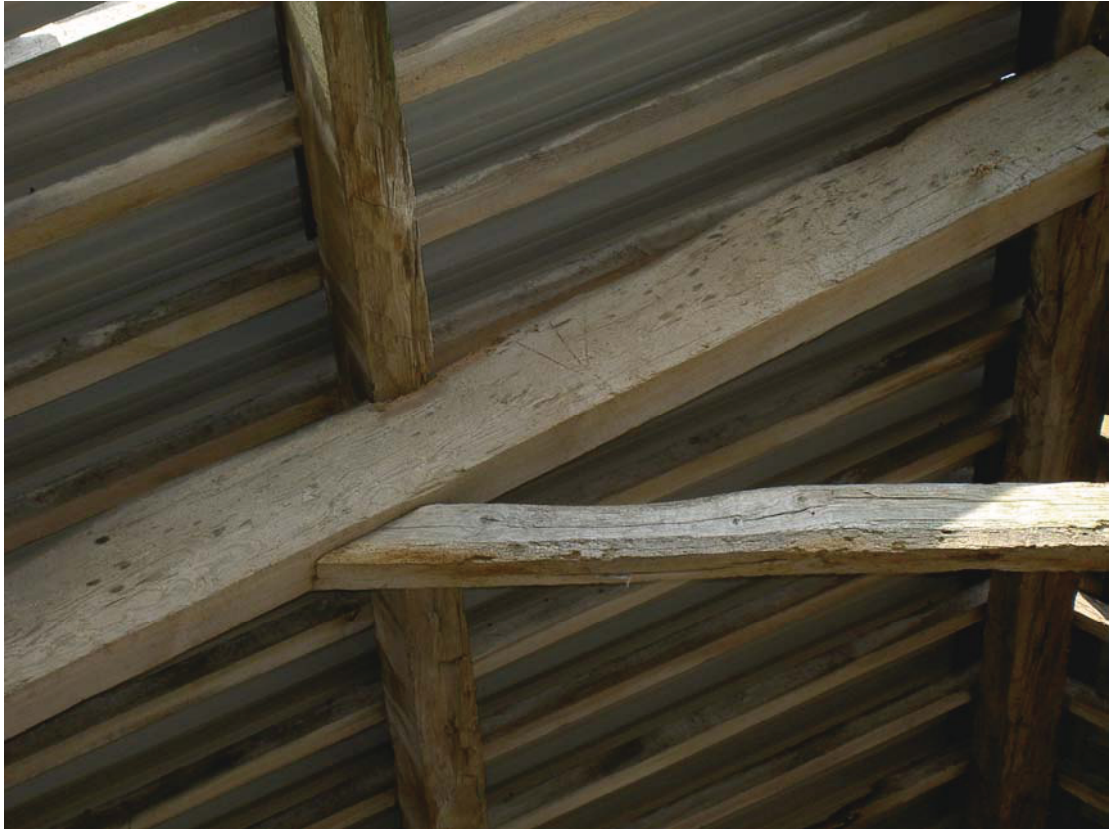
Plate 11: Probable levelling mark on truss within Room 1
