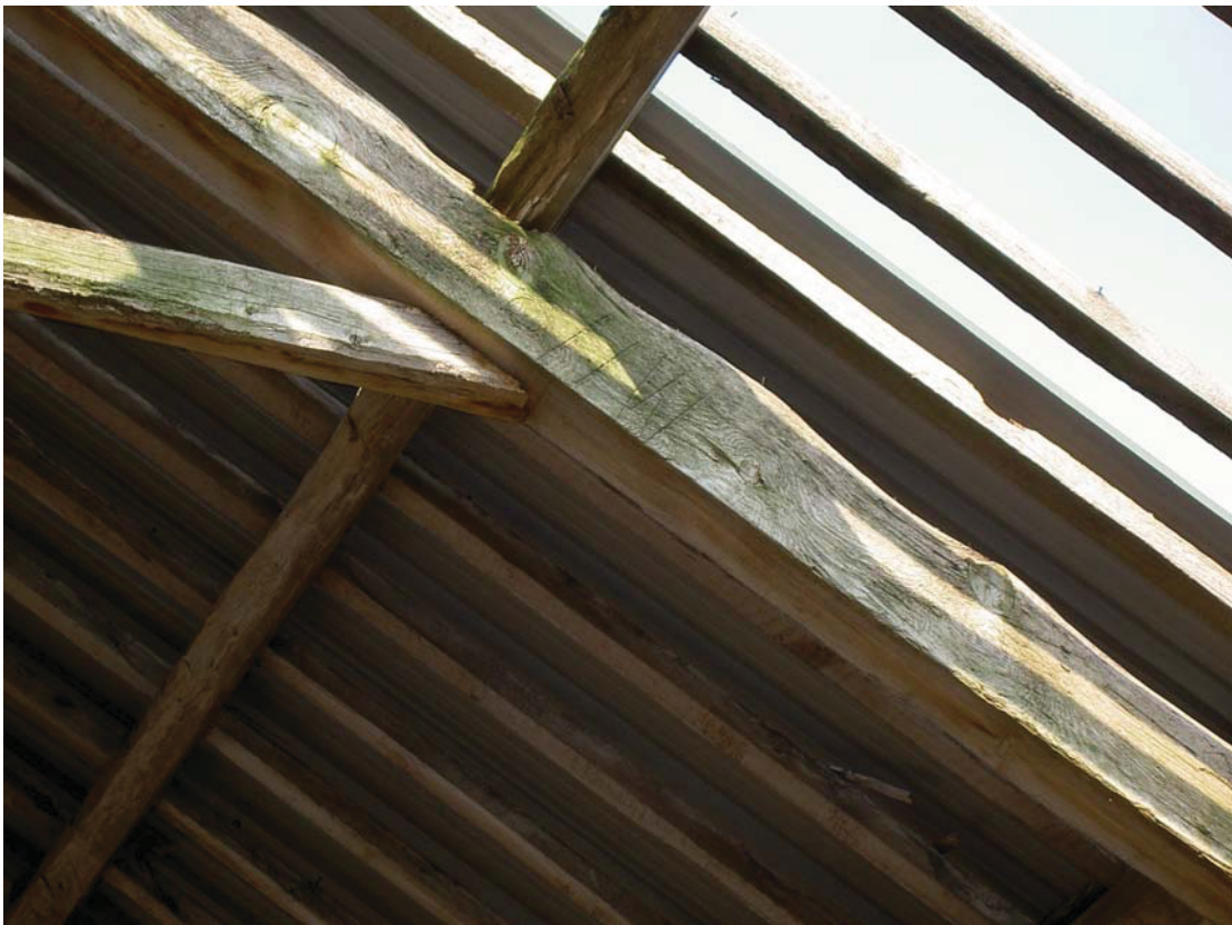
Plate 12: Levelling mark or Baltic timber mark on truss in Room 1
