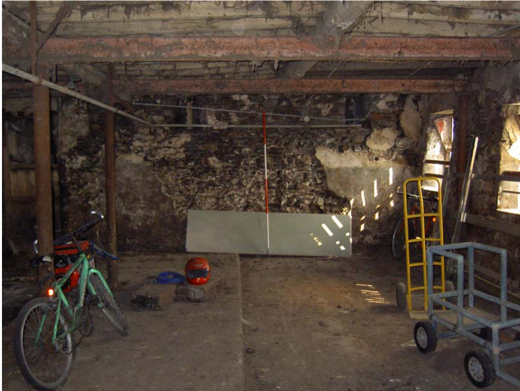
Plate 11: General view of Room 2, lower ground floor
