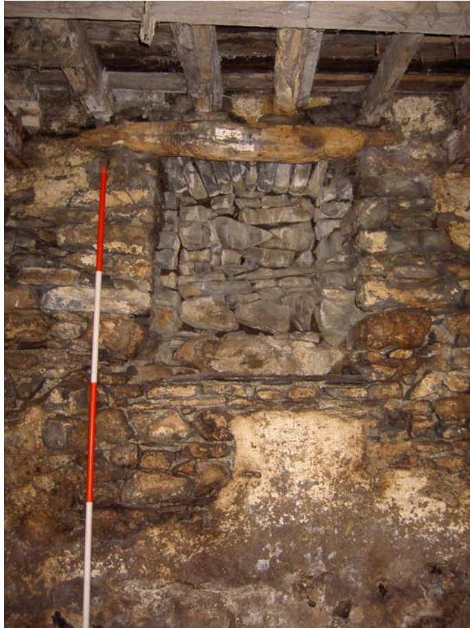
Plate 13: Blocked window, Room 2, lower ground floor
