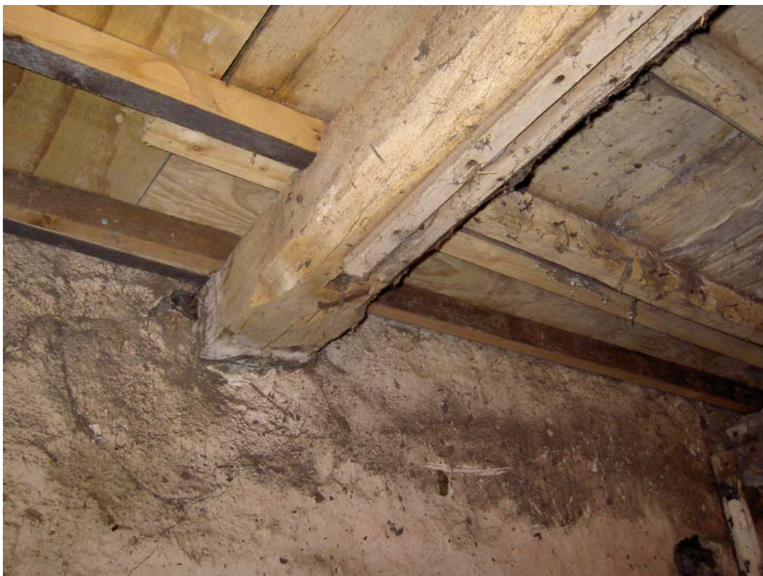
Plate 10: Detail of stop-chamfer decoration, Room 1, lower ground floor
