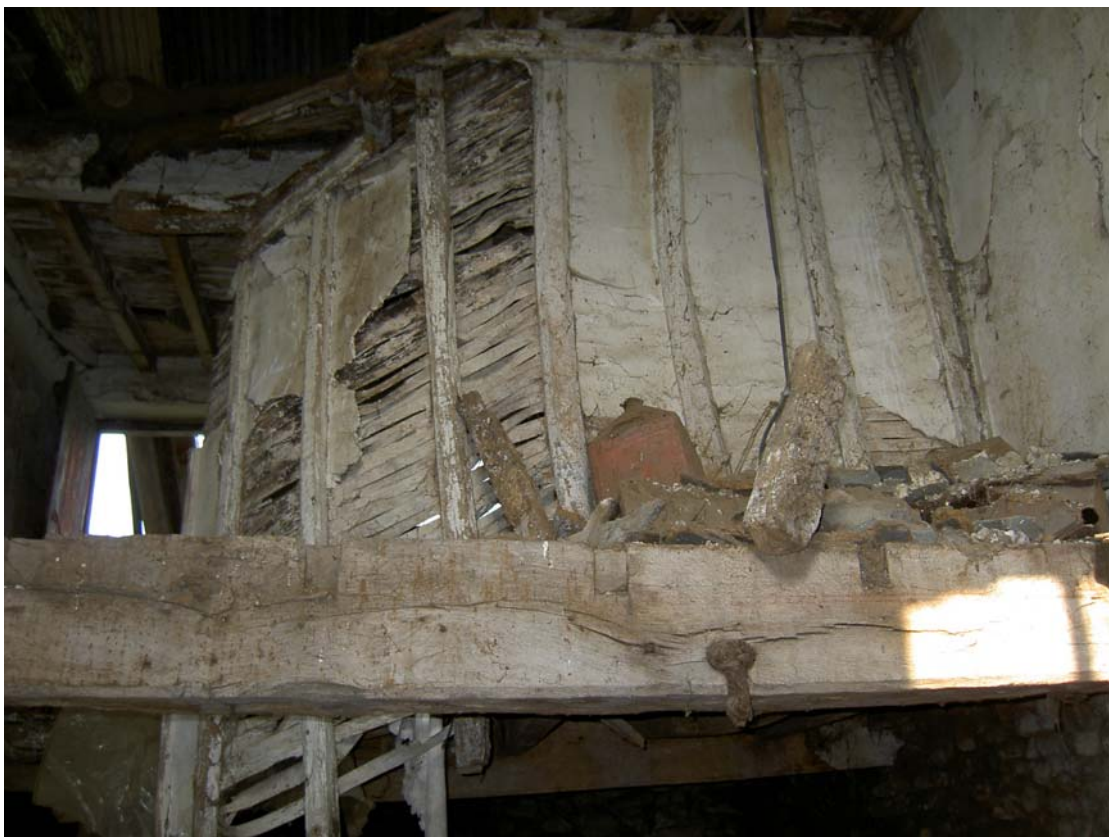
Plate 16: Remains of stud partition wall in Room 2, upper ground floor
