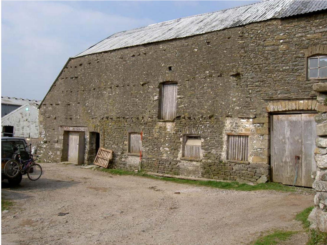
Plate 7: The centre and north-west west end of the south-west elevation
