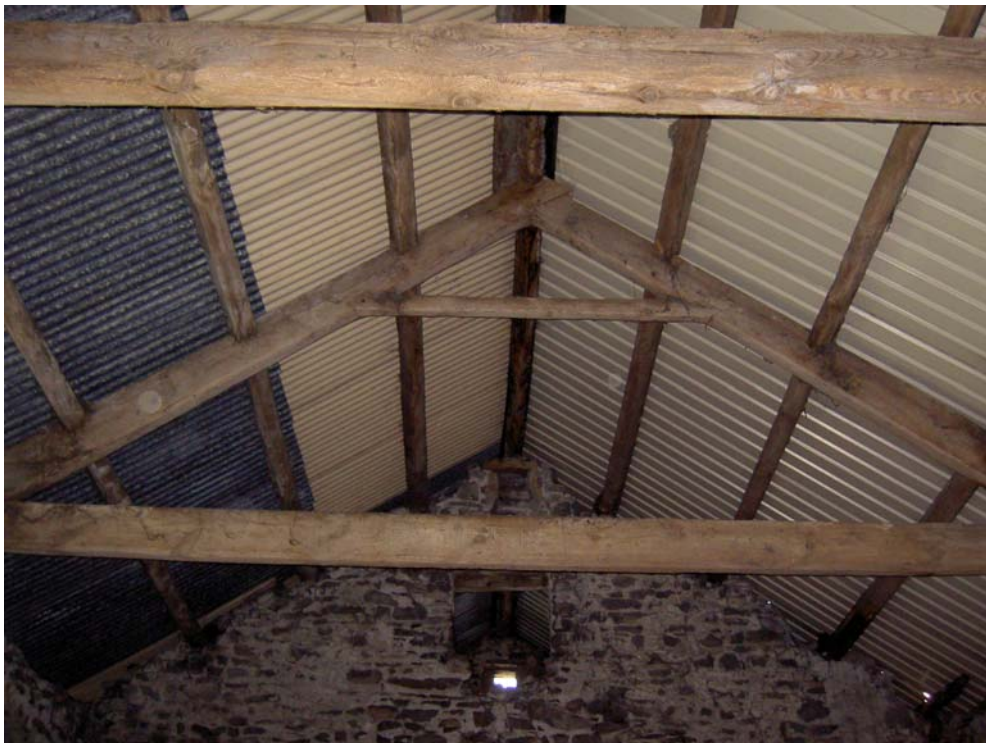
Plate 14: Detail of truss in Room 2, upper ground floor and first floor
