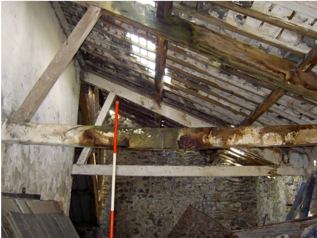
Plate 15: Half trusses in Room 3, upper ground floor
