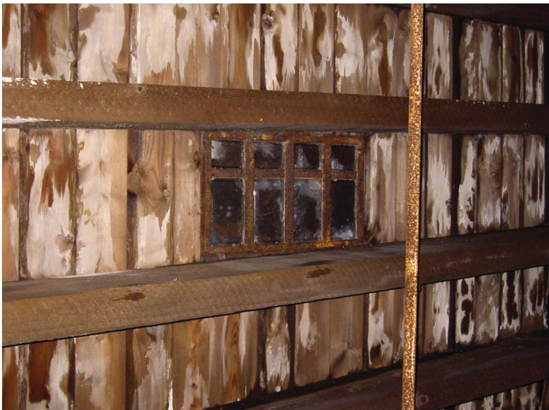
Plate 38: Iron-framed floor light in foundry Building 1
