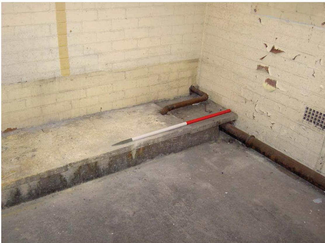
Plate 67: Concrete 'step' housing water pipe in foundry Building 5a
