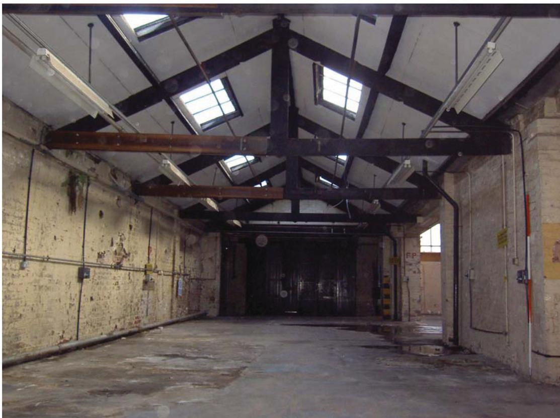
Plate 65: General view of interior of foundry Building 5 showing trusses
