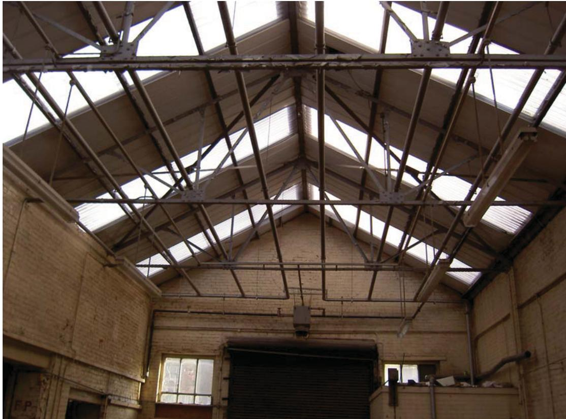
Plate 58: The steel roof structure in foundry Building 4
