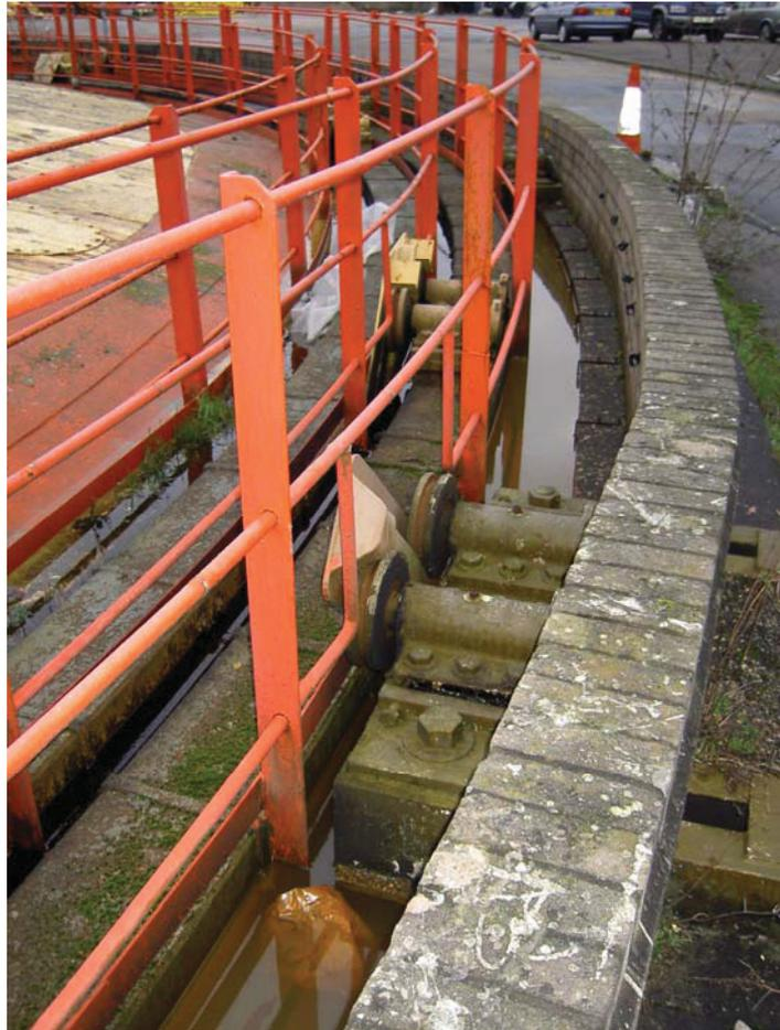
Plate 20: Detail of rolling mechanism, gasworks Building 4
