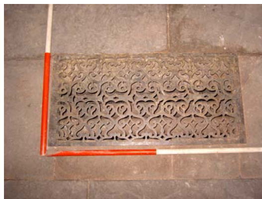
Plate 3: Iron grill in vestibule floor
