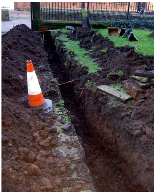
Plate 4: Area 2, looking north
