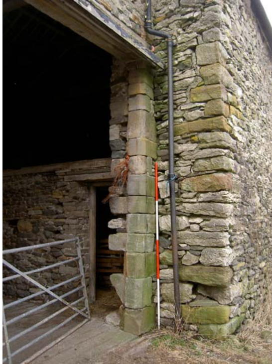
Plate 11: Detail of chamfered surround to wagon doorway, south end of east elevation
