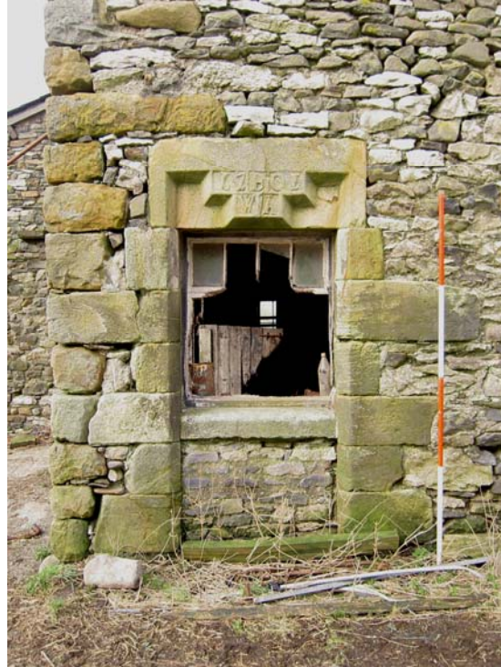
Plate 11: Detail of chamfered surround to wagon doorway, south end of east elevation
