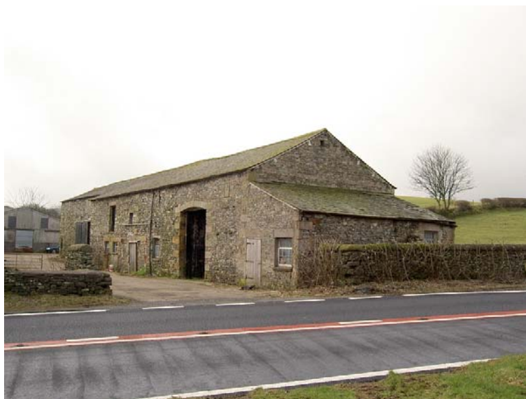
Plate 1: General view from the north-east showing the site relative to the A65
