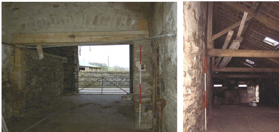
Plate 29: Wagon doorway from within small outshuts to west
