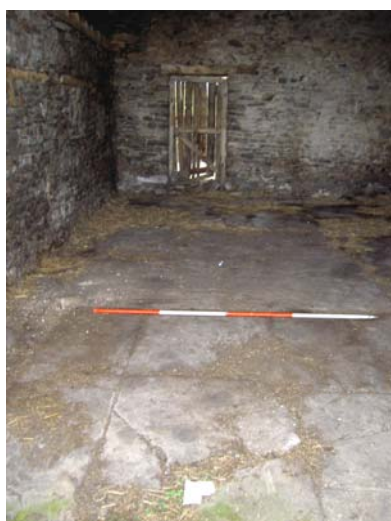
Plate 19: Stone and timber threshing floor within the north threshing barn
