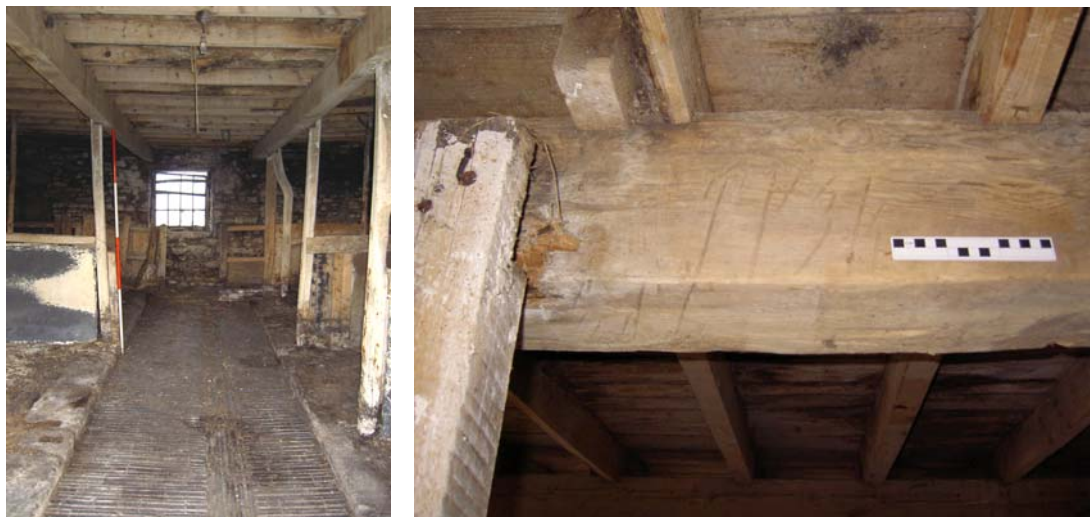
Plate 21: Stalls and dung channel within the north shippon
