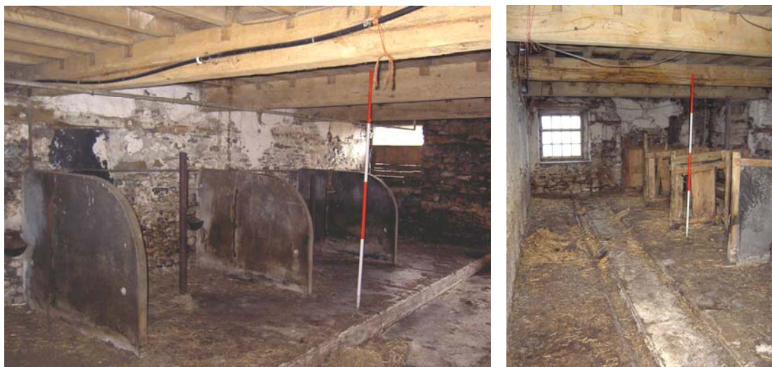
Plate 23: Concrete stall partitions in the north central shippon
