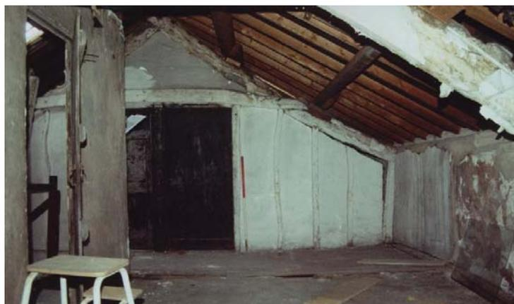
**Plate 29: Partition and ceiling scars, second floor east rooms**
