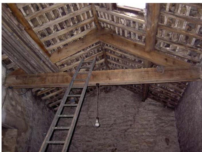
Plate 15: Tie beam truss and roof
