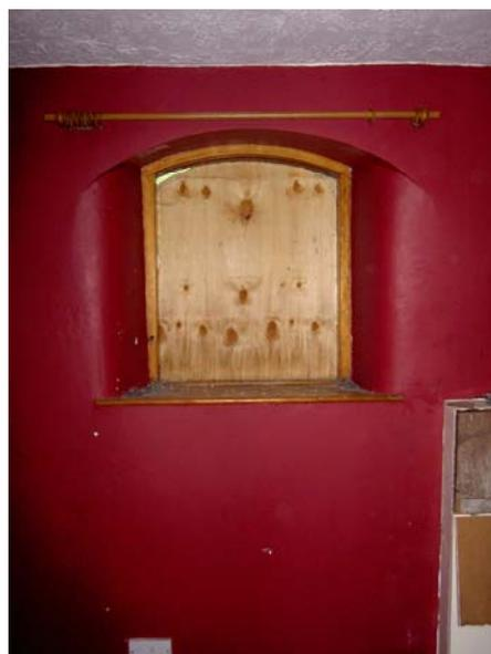
**Plate 46: (left) Converted doorway in the south-west elevation of Room G12**
