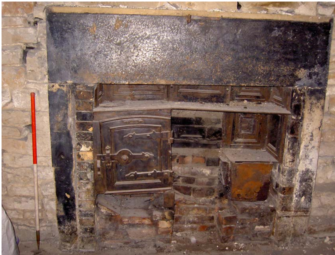
Plate 20: Basement Room 3, range
