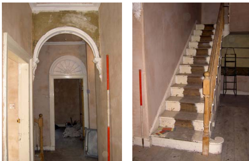
Plate 21: (left) Ground floor Room 1, decorative arch in hall with fanlight moulding beyond
