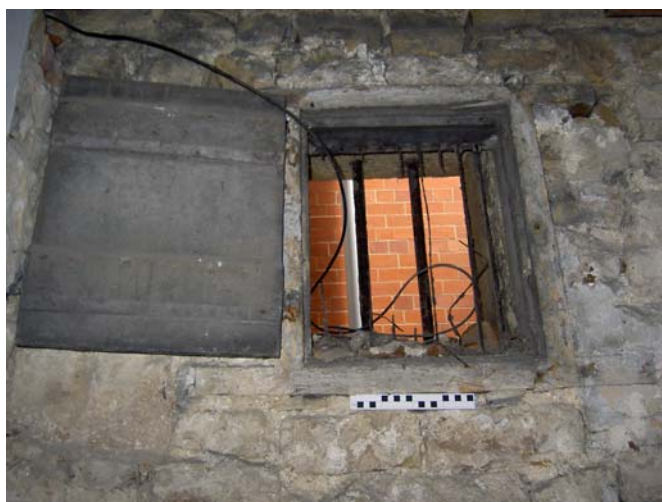
Plate 17: (left) Basement Room 2, window and shutter
