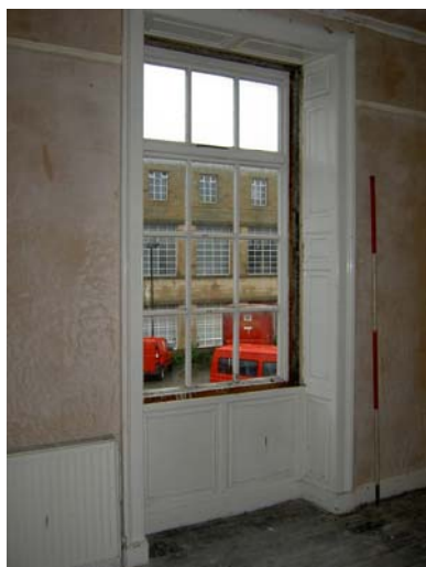
Plate 25: (left) First floor Room 1, window
