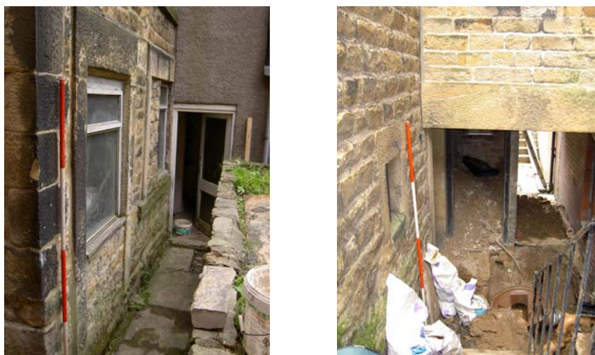
Plate 15: (left) Blocked door and window, west external elevation
