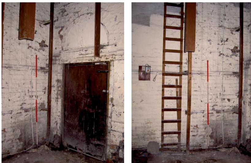
**Plate 49: (right) Ground floor, Room 3, doorway and timber tracks of elevator shaft**
