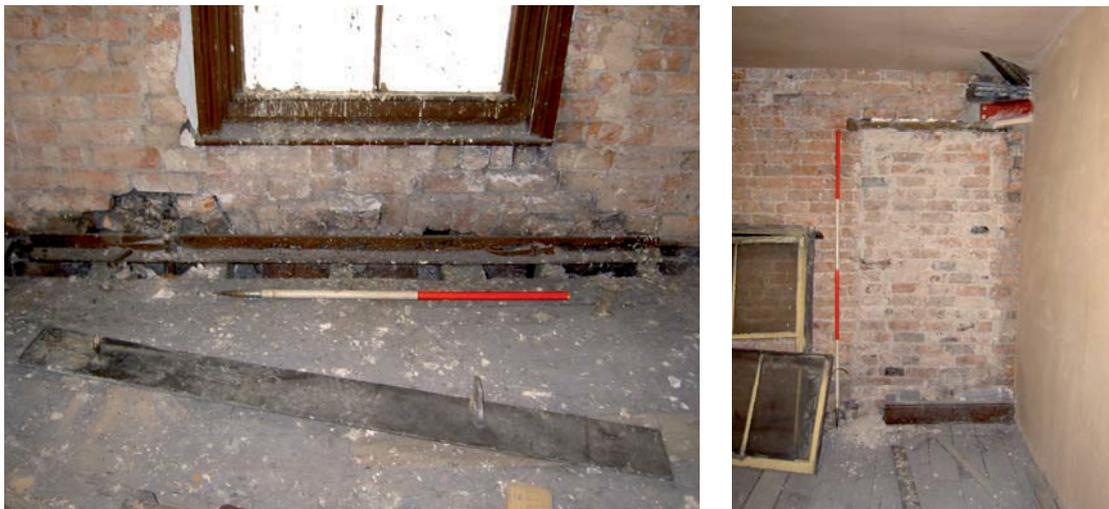
Plate 55: (left) First floor, Room 1, iron strap attached below window in north-east elevation
