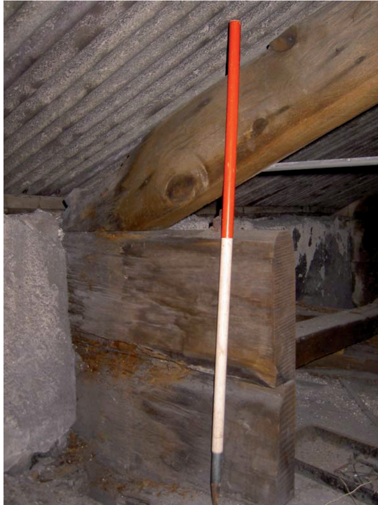
Plate 19: Spacers between tie-beam and principals
