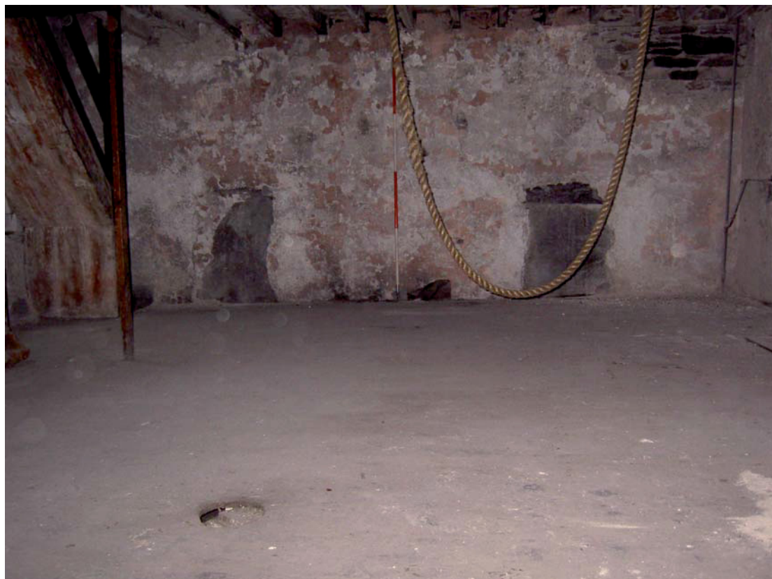
Plate 12: Blocked apertures in west wall of first floor
