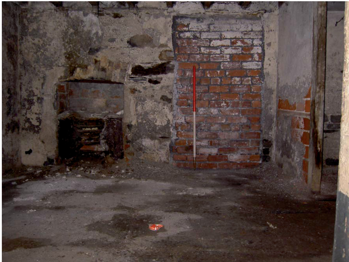
Plate 7: Fireplace, blocked door, and partition in cellar
