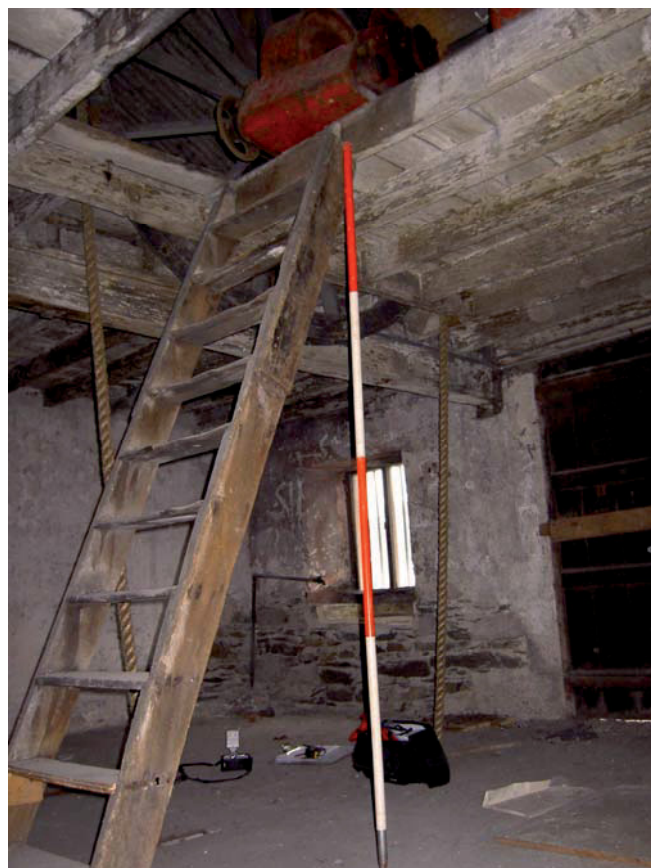
Plate 16: Loft access from second floor, looking north-west
