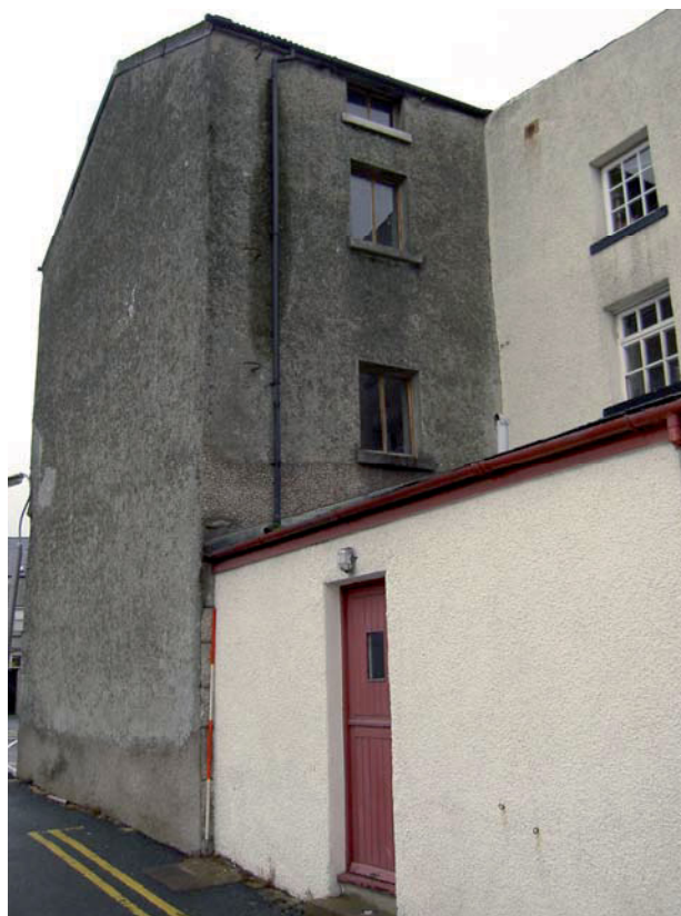
Plate 6: South elevation, showing recent ground floor addition to No.1
