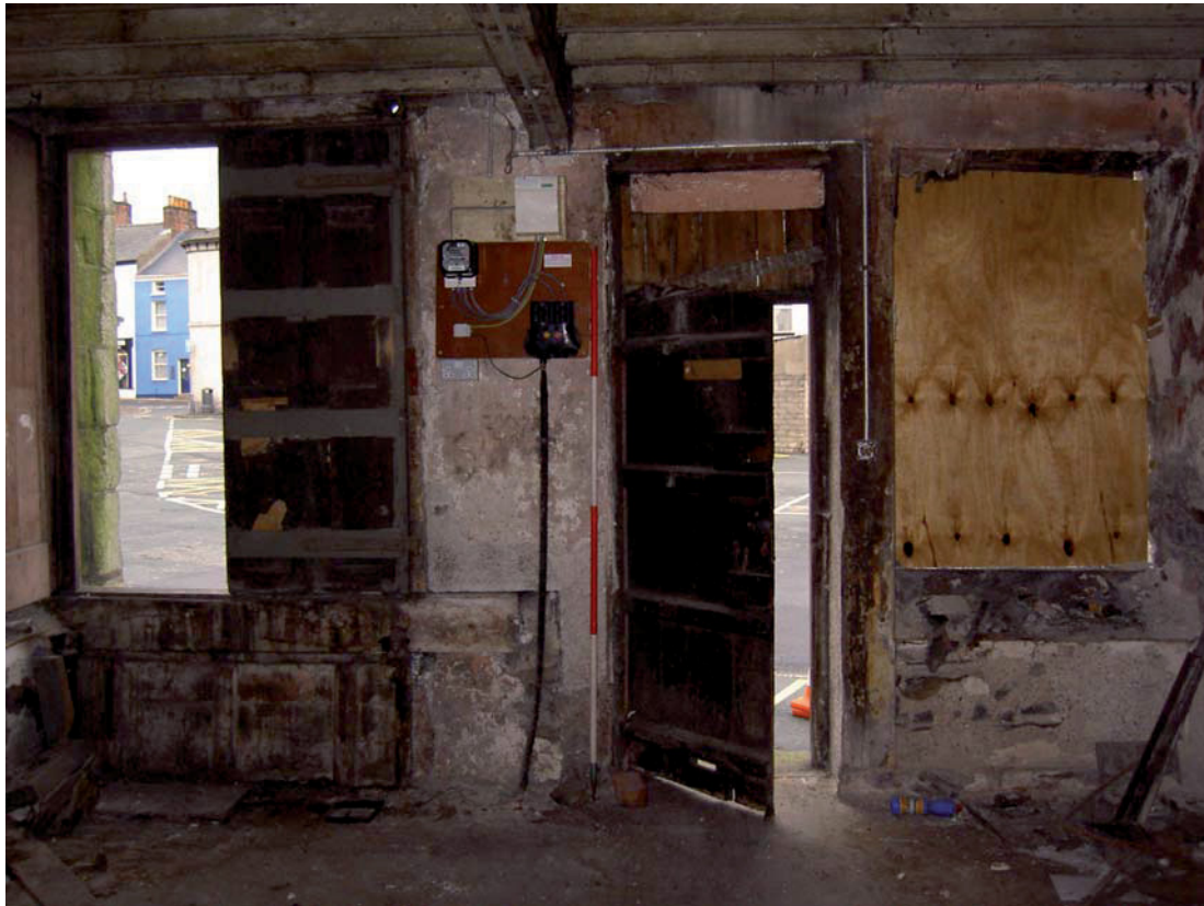
Plate 11: Interior of east side of ground floor looking north
