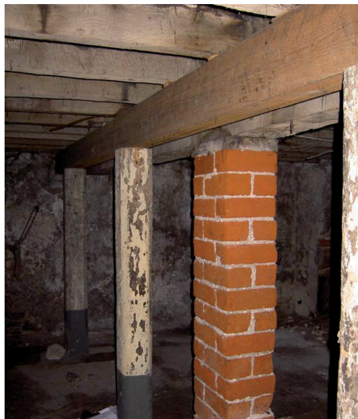
Plate 8: Inserted beam in cellar
