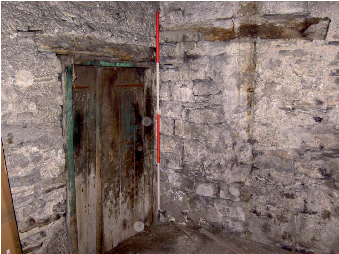
Plate 9: Ground floor west side showing entrance to cellar and blocked door in southern elevation
