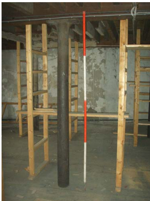
Plate 35: Detail of an iron column on the third floor
