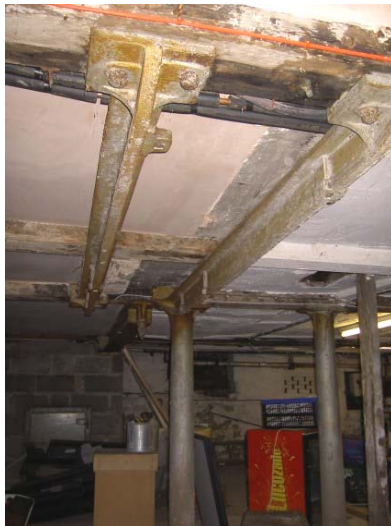
Plate 70: (left) Iron I-beams in a Y-shaped arrangement
