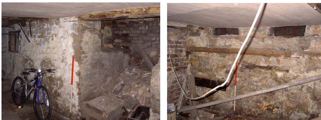
Plate 76: (left) Projecting area on the south elevation of Room 1
