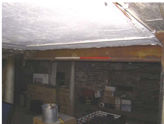
Plate 72: (left) Square iron I-beam
