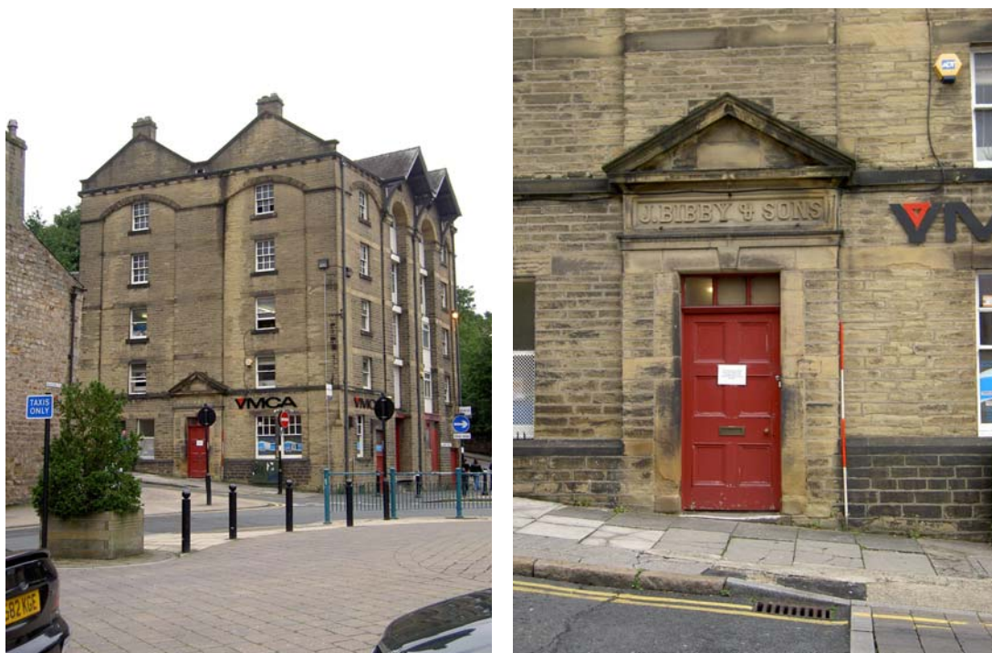
Plate 12: (left) East elevation, facing onto New Road
