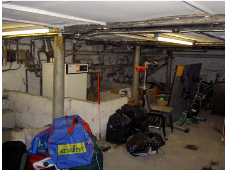
Plate 69: Low concrete block wall on east side of Room 2
