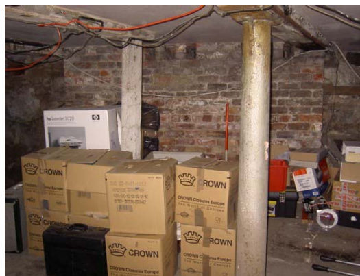
Plate 73: (right) One of the timber supports below the additional east/west beam
