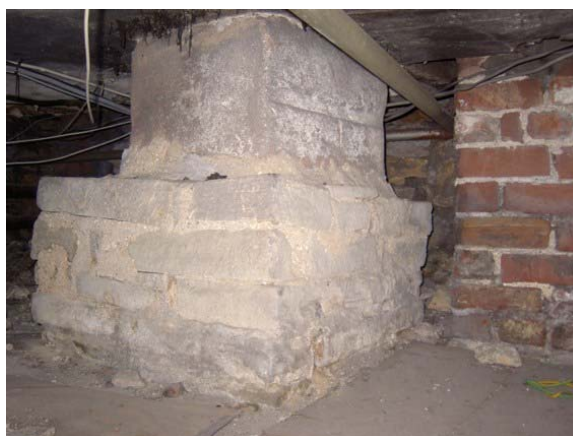
Plate 78: Stone-built column in the small crawl space (Room 3)
