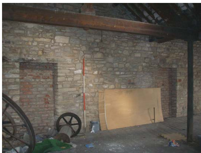
Plate 32: West elevation showing blocked 'apertures'
