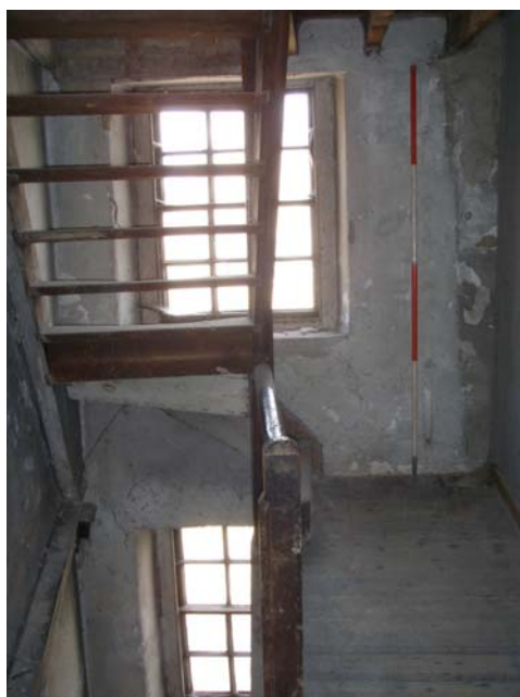
Plate 41: Stairwell on the third floor
