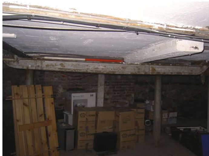
Plate 70: (left) Iron I-beams in a Y-shaped arrangement
