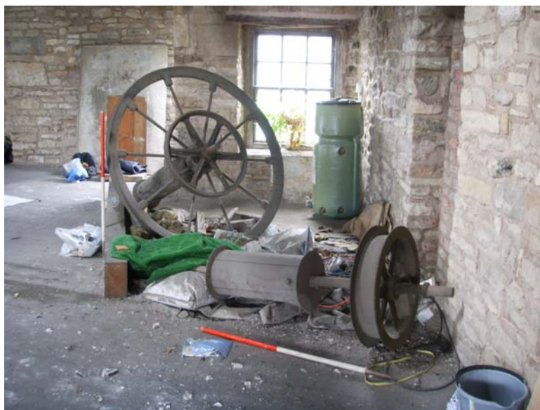
Plate 25: Loose pulley wheels from the hoist
