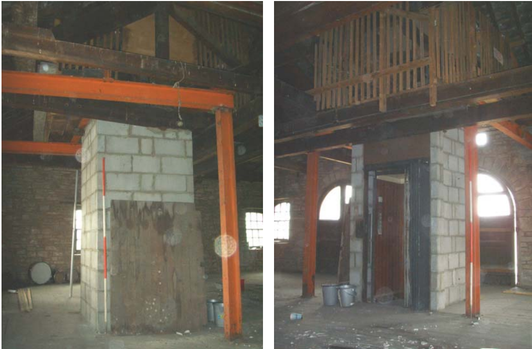
Plate 23: (left) I-beam structure built around the lift shaft
