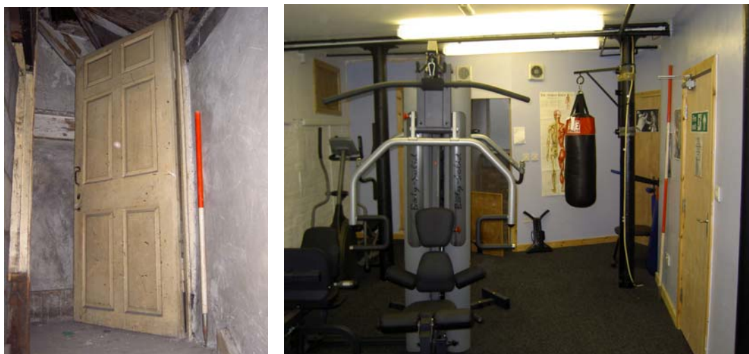
Plate 56: (left) Original six-panel bevel raised and ovolo-moulded door with a chamfered frame in Room 1
