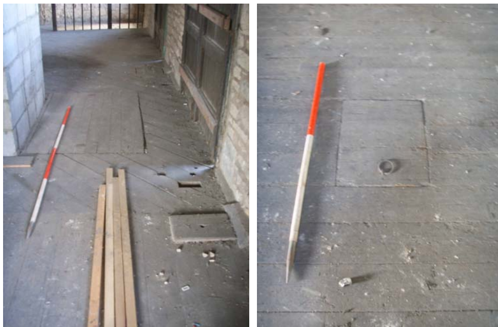
Plate 26: (left) View of the tongue and groove floorboards and large hatch on the north side of the fourth floor
