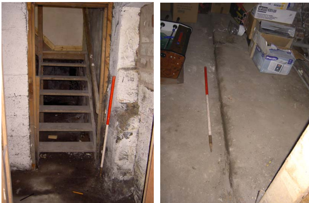
Plate 67: (left) Stairwell to the basement ( Room 1a )
