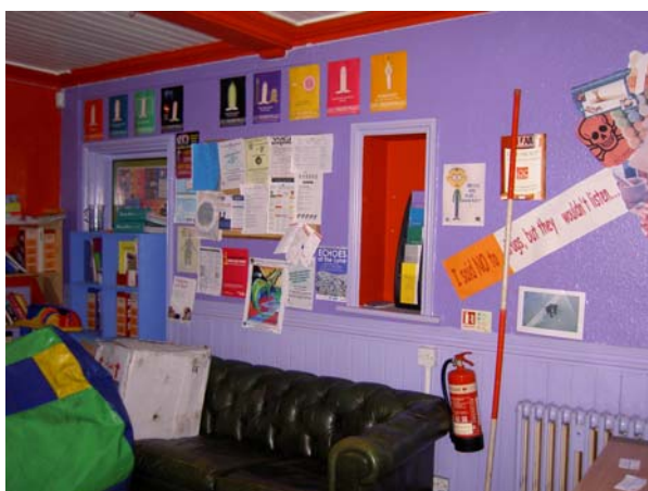
Plate 66: Room 6 , blocked doorway and window in the west elevation
