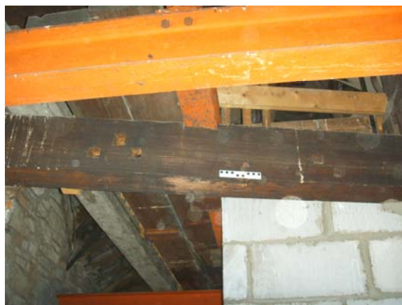
Plate 19: (left) Pair of east/west beams supporting a wheel and drum
