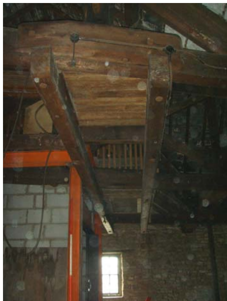
Plate 19: (left) Pair of east/west beams supporting a wheel and drum
