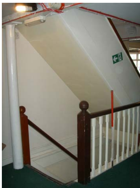
Plate 55: Staircase on the first floor
