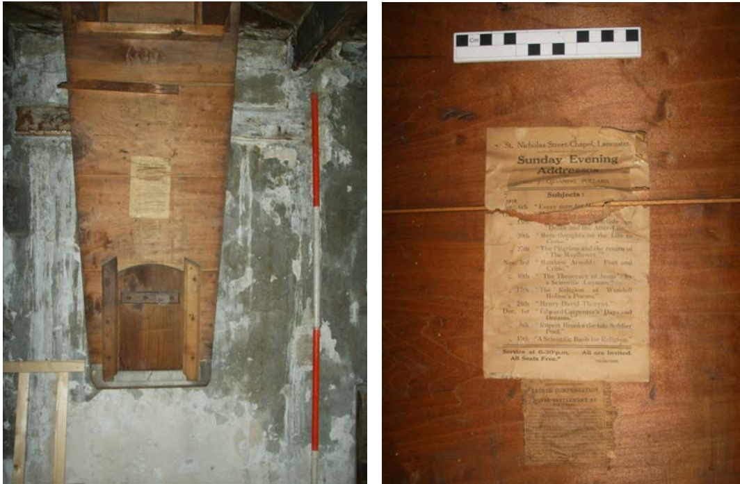
Plate 43: (left) Centrally-located timber hopper
