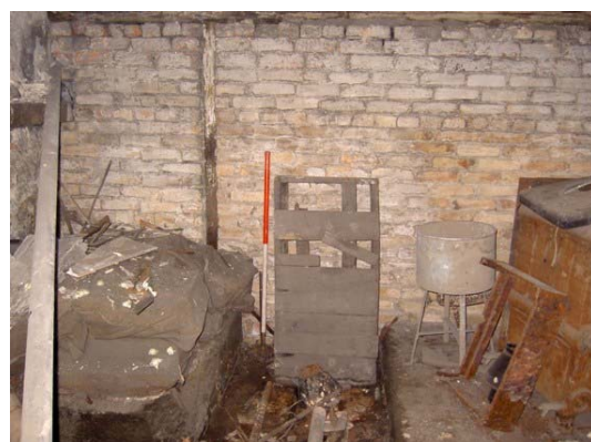
Plate 74: (left) North elevation to the west of Room 1
