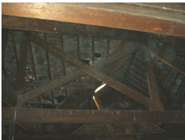
Plate 18: Crossed angled braces within the roof structure
