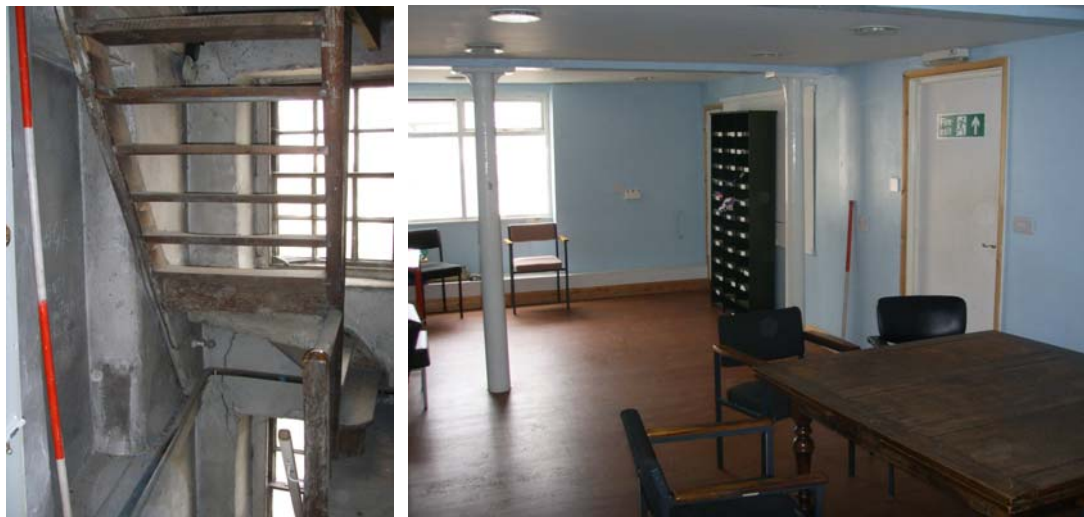
Plate 47: (left) Stairwell on the second floor
