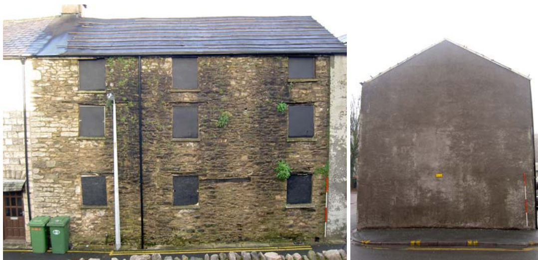
Plate 12: (left) South external elevation of cottages
