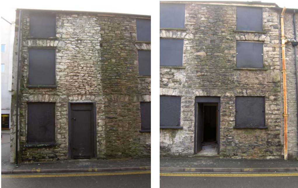
Plate 10 (left) West side of north elevation of cottages
