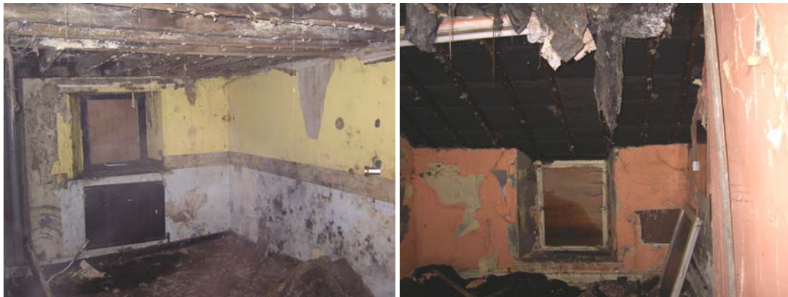
Plate 20: (left) South and west elevation of Room 13
