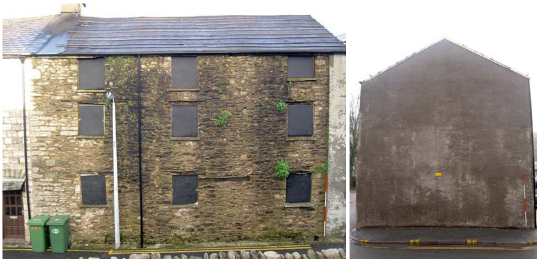
Plate 12: (left) South external elevation of cottages
