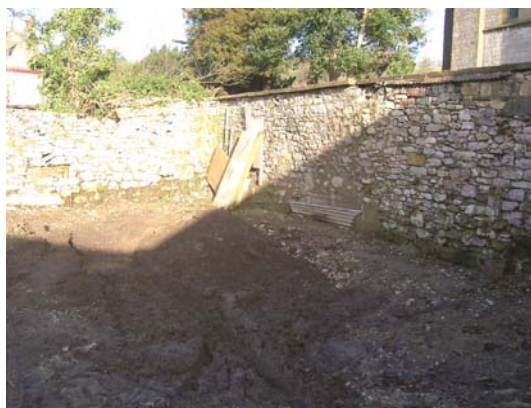
Plate 6: (left) North-east part of site from the south
