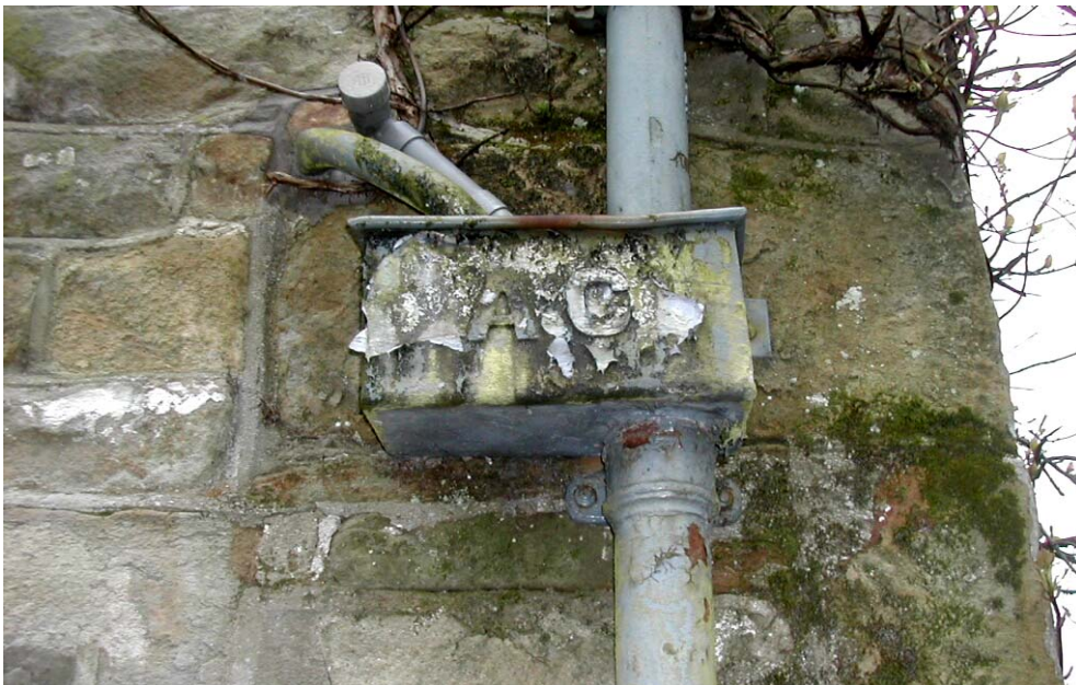
Plate 5: Hopper on west end of north elevation (courtesy of Mike Westwood)
