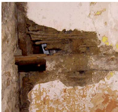
Plate 23: (left) Detail of 'mud and stud' in Room 10/9
