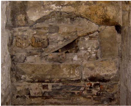
Plate 13: (left) Blocked up bread oven in kitchen
