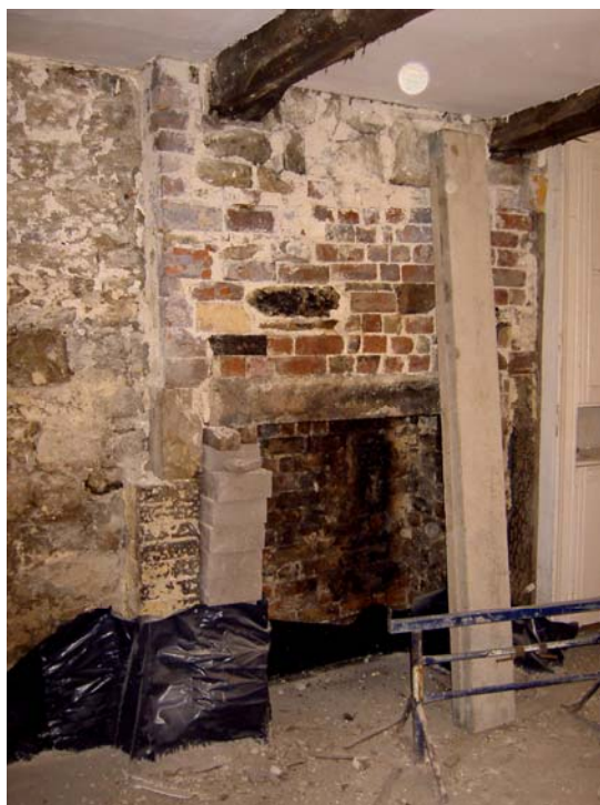
Plate 19: (left) Inserted chimney breast in the living room, ground floor
