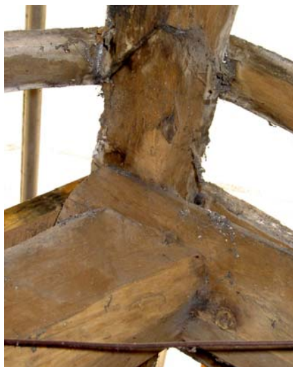
Plate 29: (left) Jointing of ridge purlin and detail of principle rafters (west truss)
