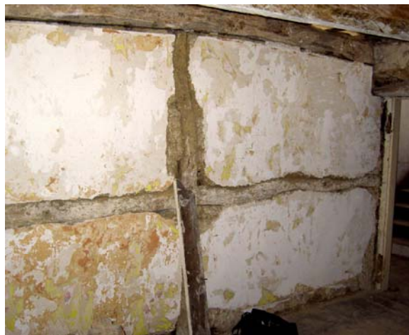
Plate 23: (left) Detail of 'mud and stud' in Room 10/9
