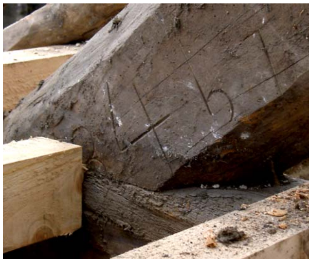
Plate 29: (left) Jointing of ridge purlin and detail of principle rafters (west truss)
