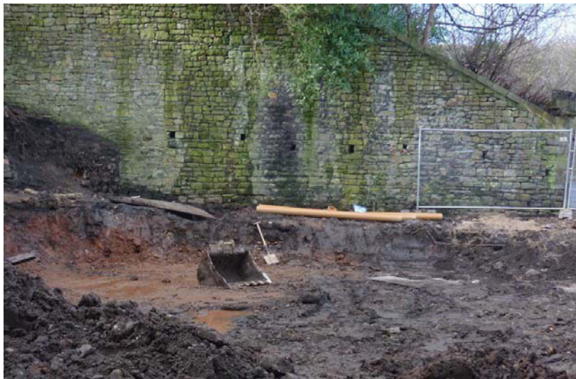
Plate 14: Open area excavated towards the north-west side of the site
