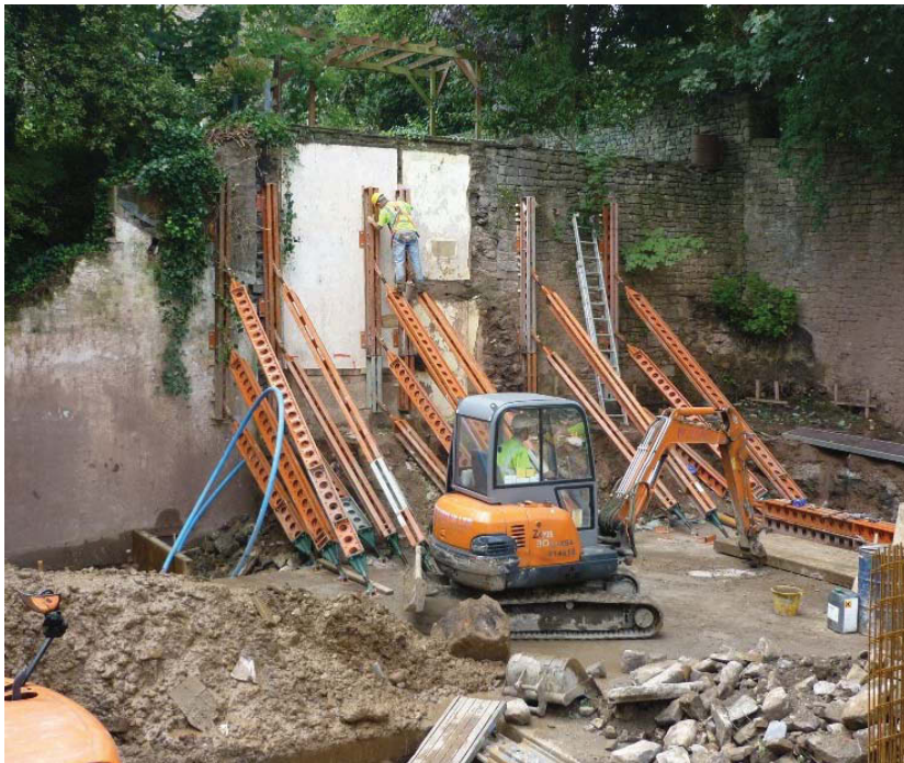
Plate 24 (left): Propping of the south-west wall
