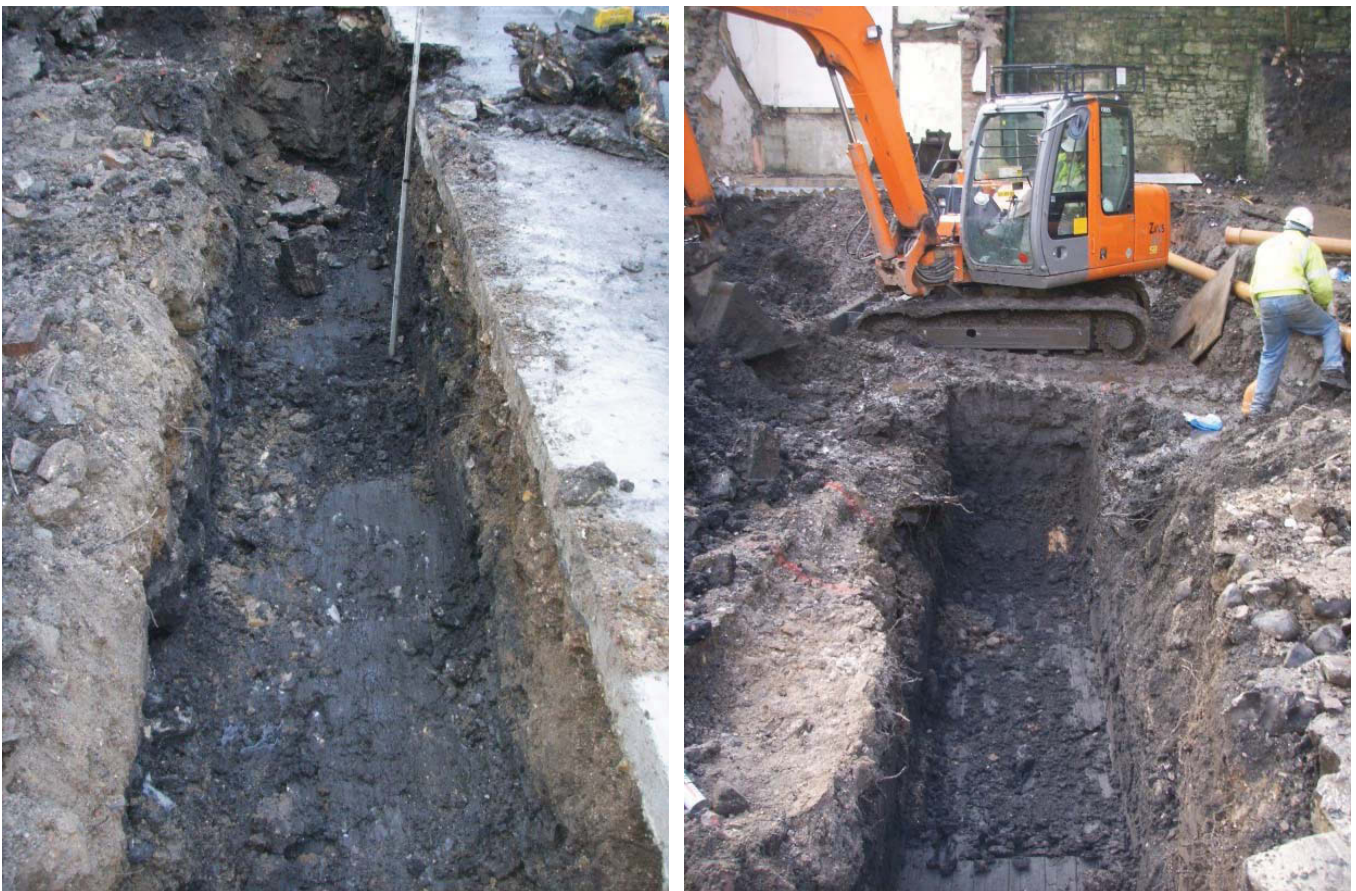
Plate 15 (left): Context 10 exposed in Trench A, looking west
