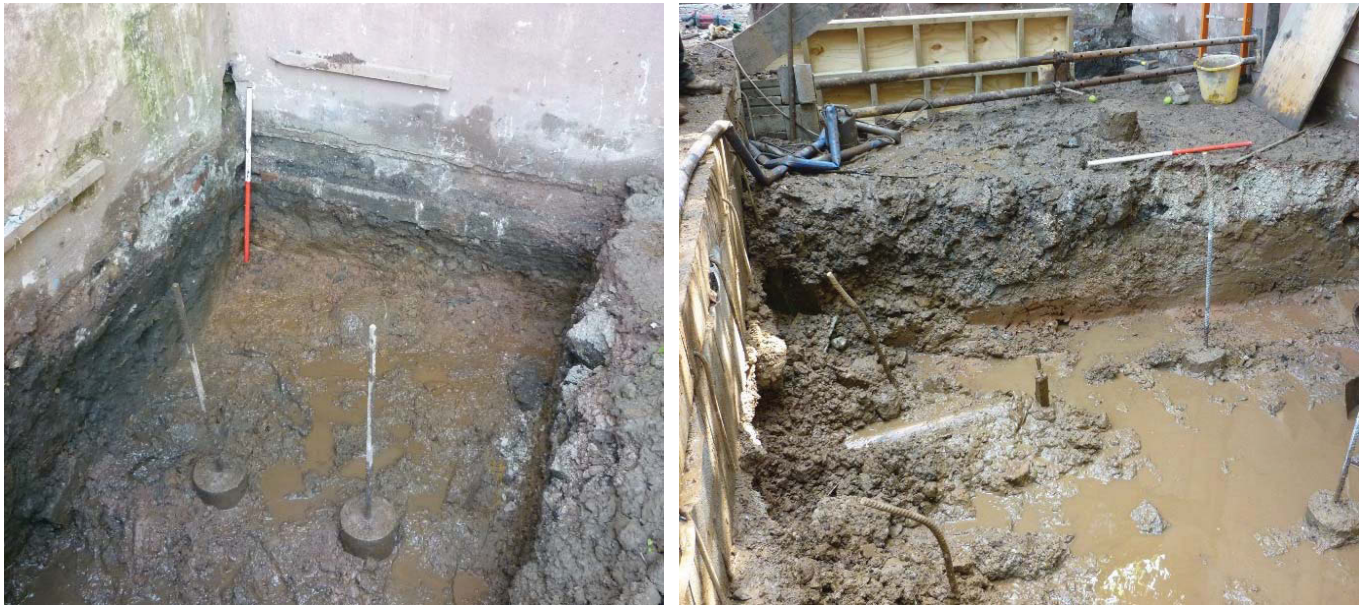
Plate 22 (left): South-east corner of the site post-excavation
