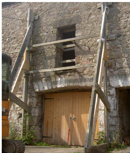
Plate 15 (left): Wagon doorway of Room 2 under an inserted winnowing door of Room 7
