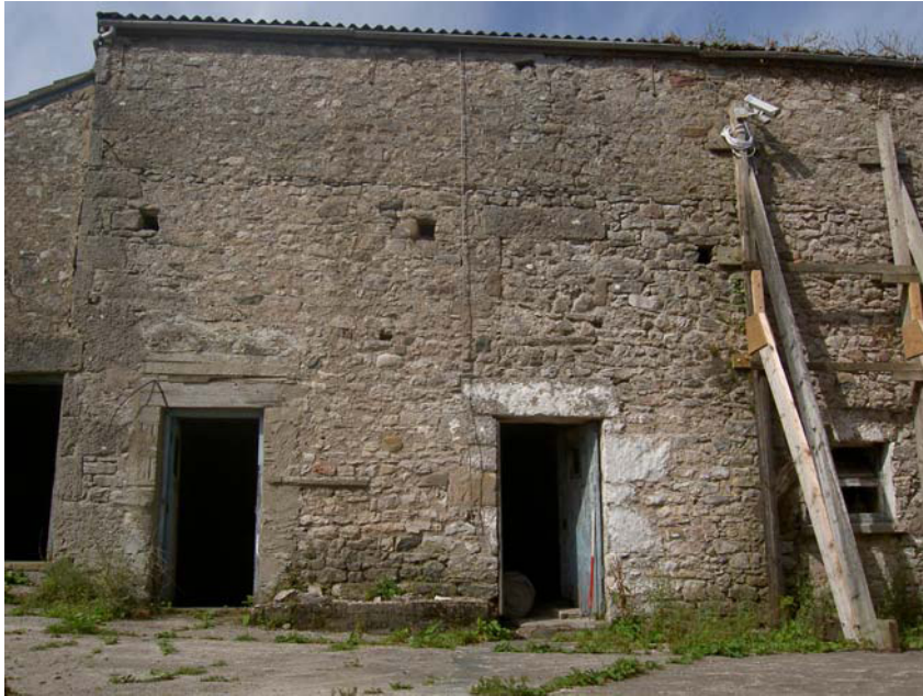
Plate 13 (left): West end of the south elevation with blocked pitching door over Room 4/4a
