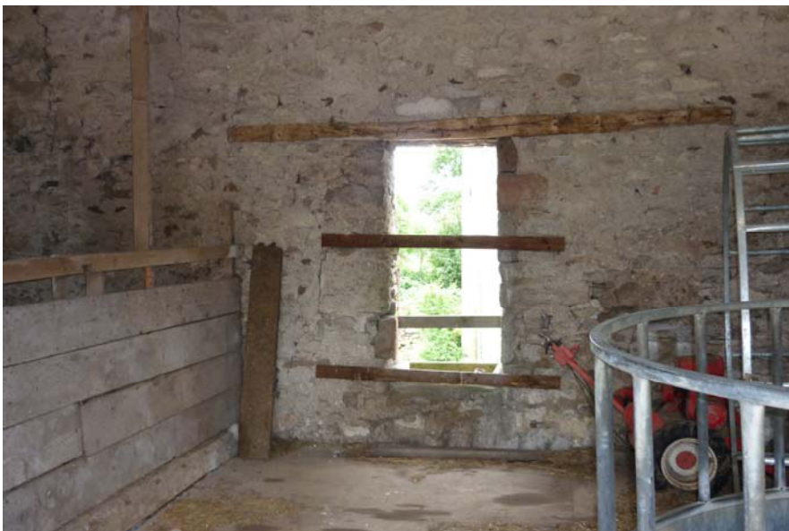
Plate 25 (left): Inserted winnowing door in south elevation of Room 7
