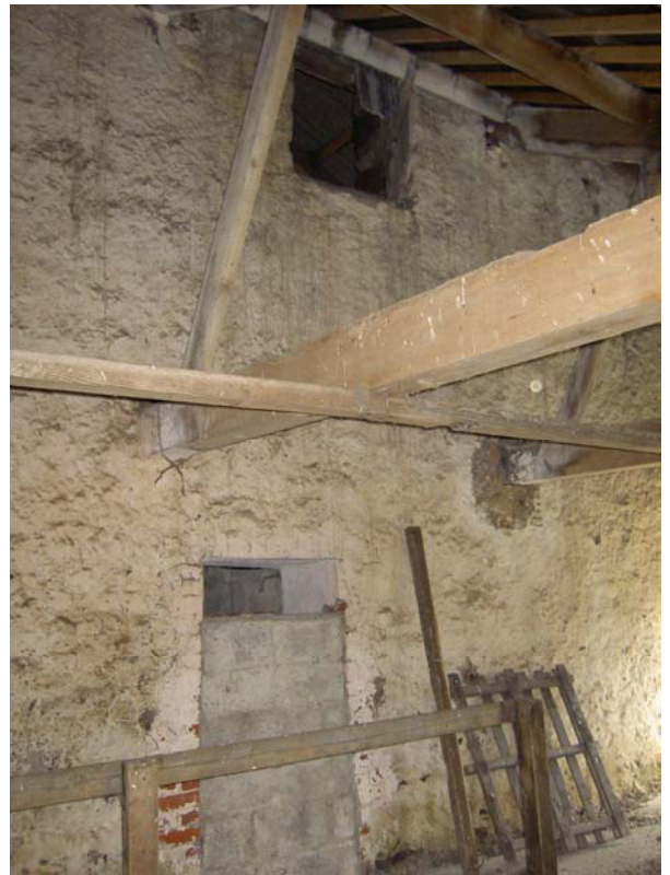
Plate 8 (left): Original access to the upper floor in the west elevation of the main barn
