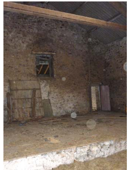
Plate 25 (left): Inserted winnowing door in south elevation of Room 7
