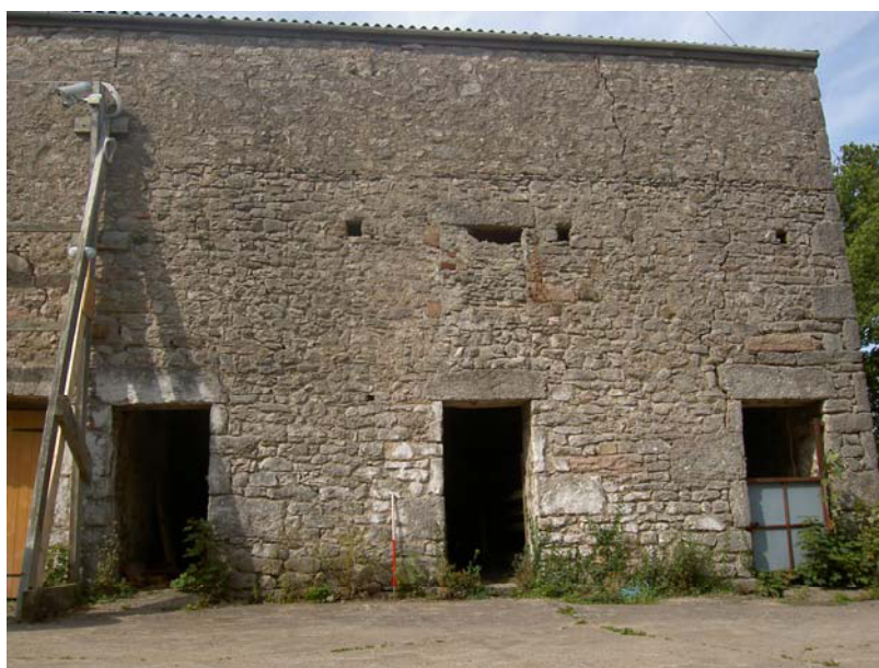
Plate 15 (left): Wagon doorway of Room 2 under an inserted winnowing door of Room 7
