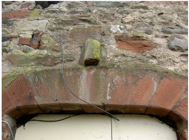
Plate 13: (left) Doorway on the south side of east elevation with re-used column fragment above
