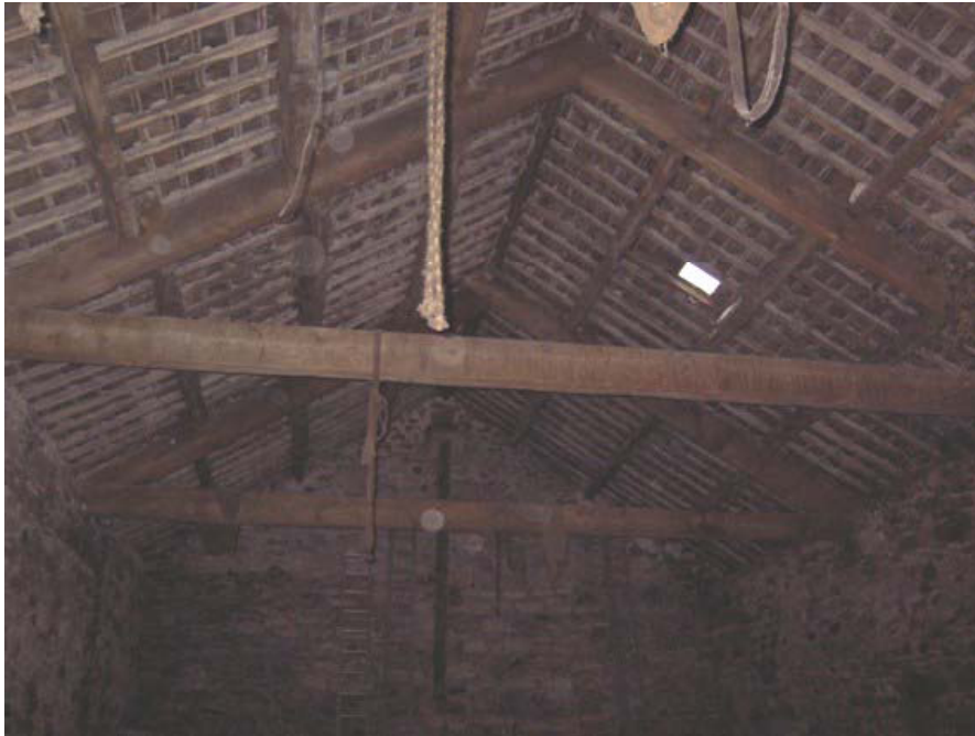
Plate 16: Trusses within the upper floor
