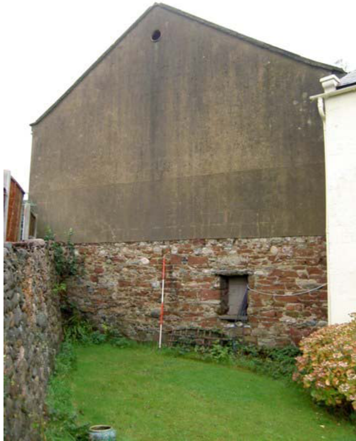
Plate 15: South elevation of barn
