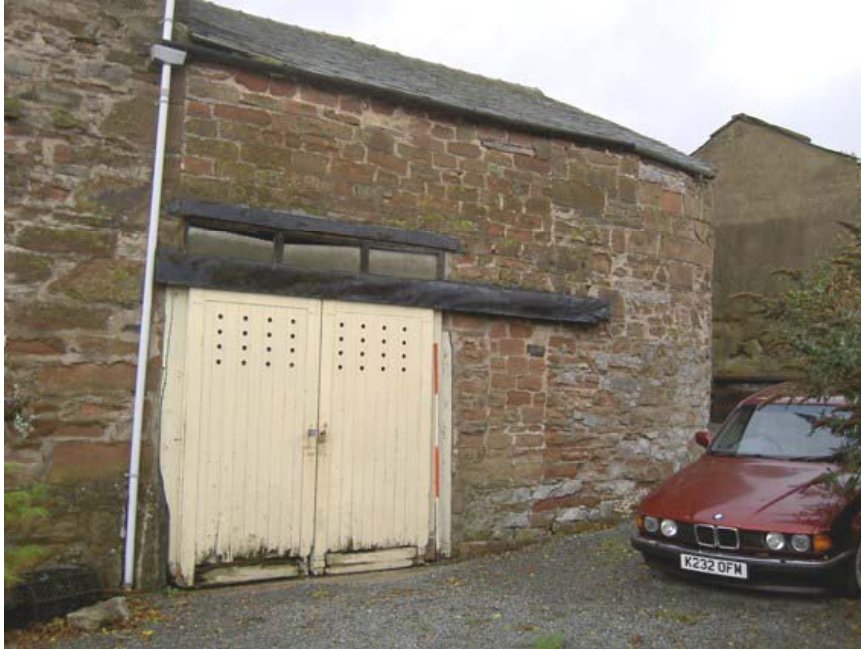
Plate 10: The east elevation of the north extension
