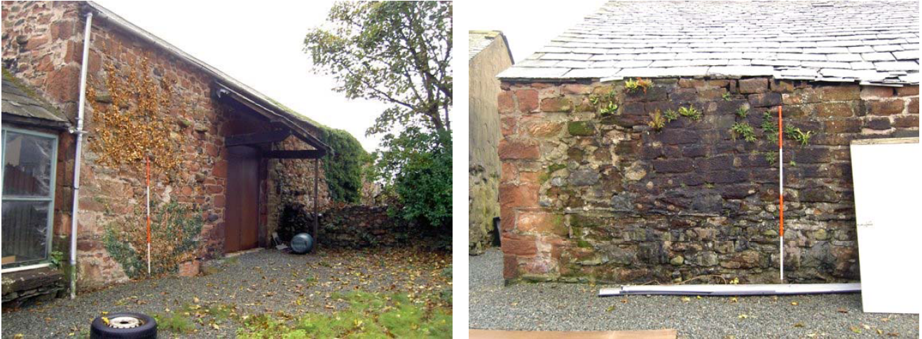
Plate 7: (left) The wagon doorway in the west elevation
