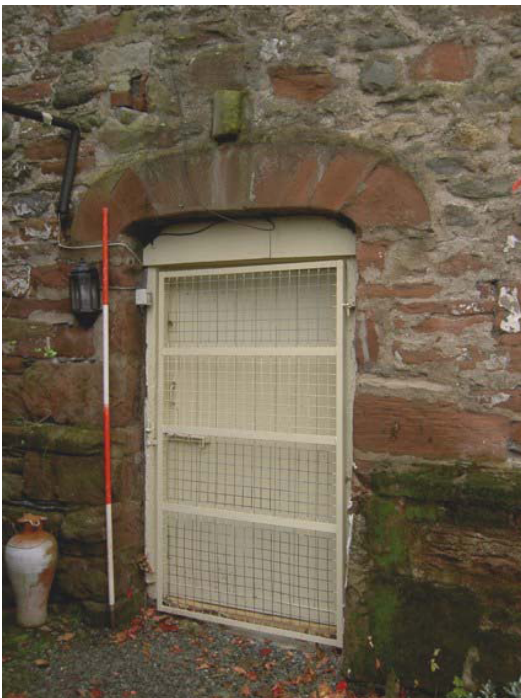
Plate 13: (left) Doorway on the south side of east elevation with re-used column fragment above
