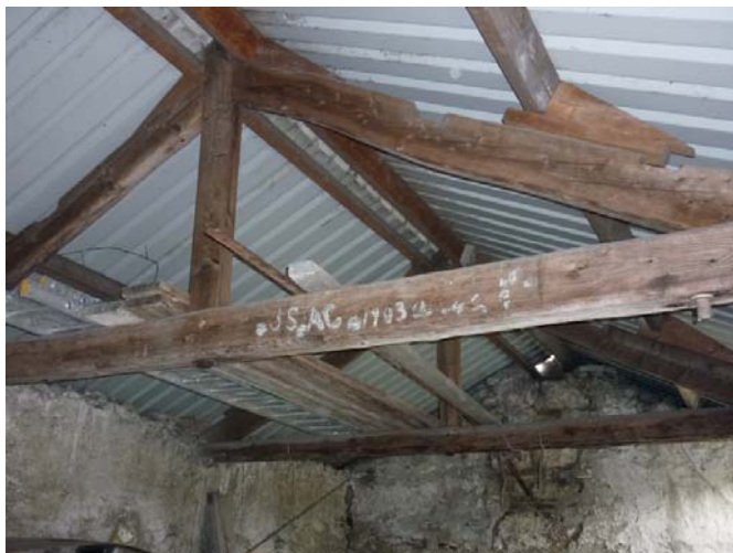
Plate 22: Internal support structure of the garage roof
