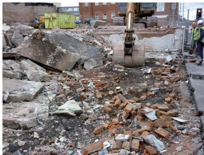
Plate 9 (left): Removal of concrete floors to the north-west of site
