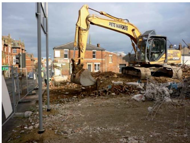
Plate 14 (left): Removal of brick-built platform midway along Corporation Street
