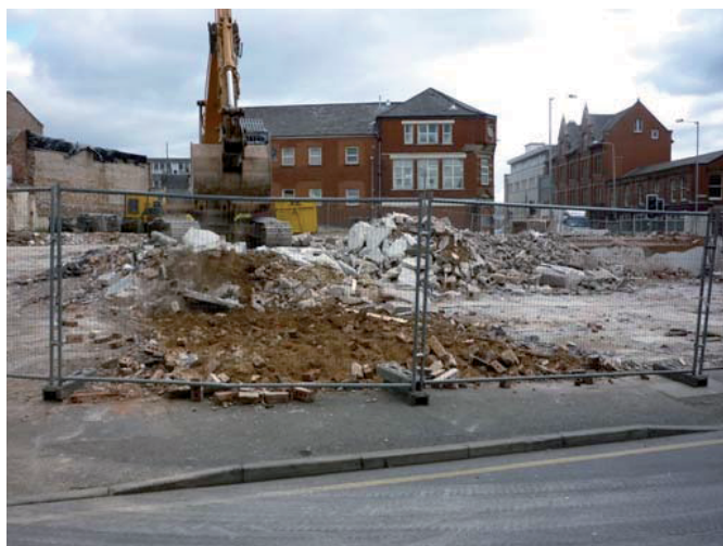
Plate 9 (left): Removal of concrete floors to the north-west of site
