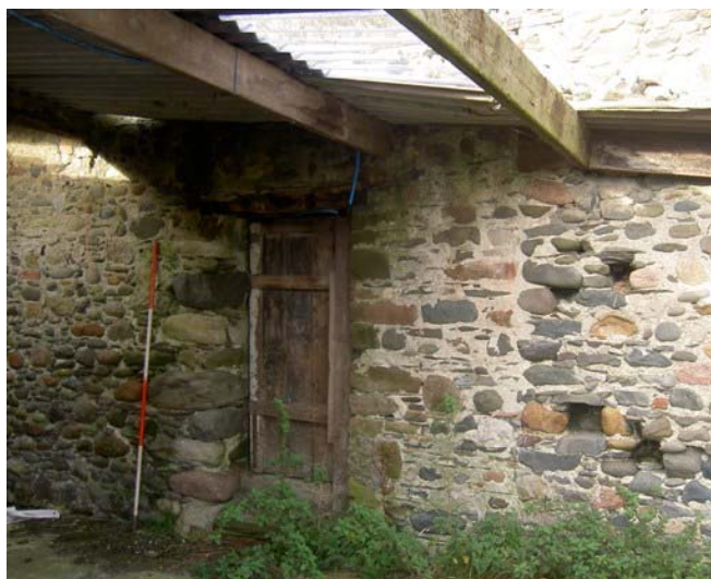
Plate 26 (left): North interior elevation of Building 3 showing the part blocked wagon doorway
