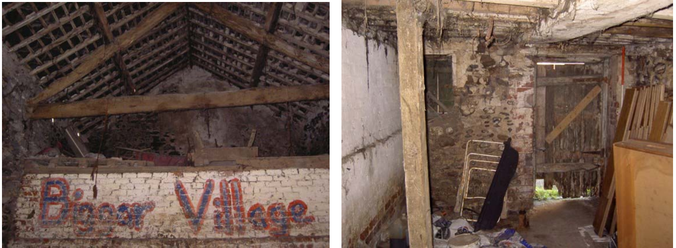
Plate 16 (left): Partition and half loft, Building 1
