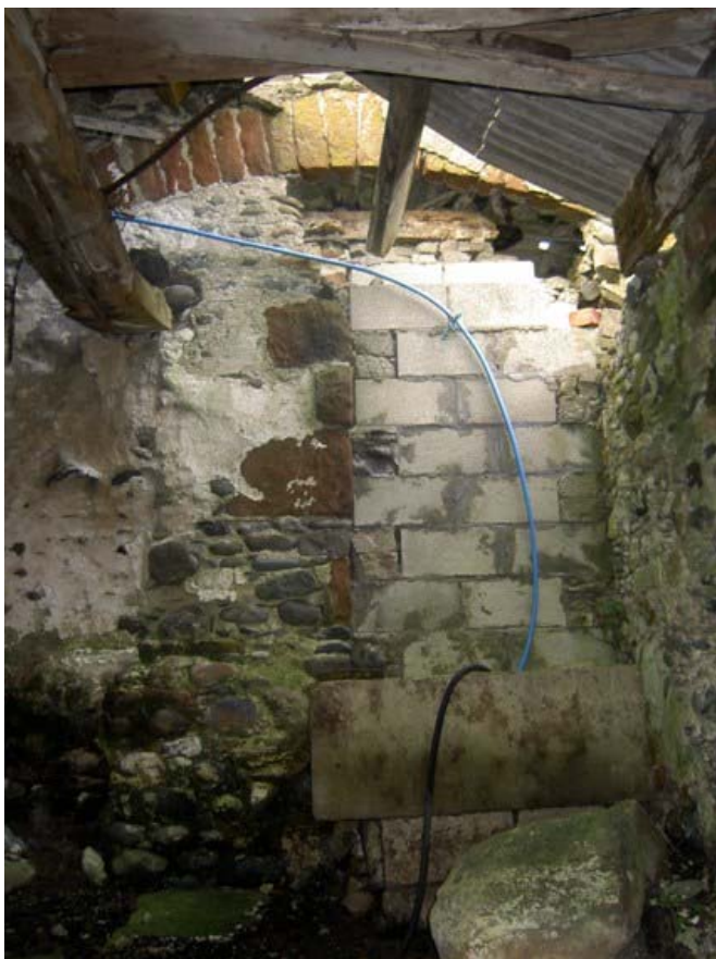
Plate 30 (left): Blocked door in the south elevation of Building 3, viewed from inside Building 4
