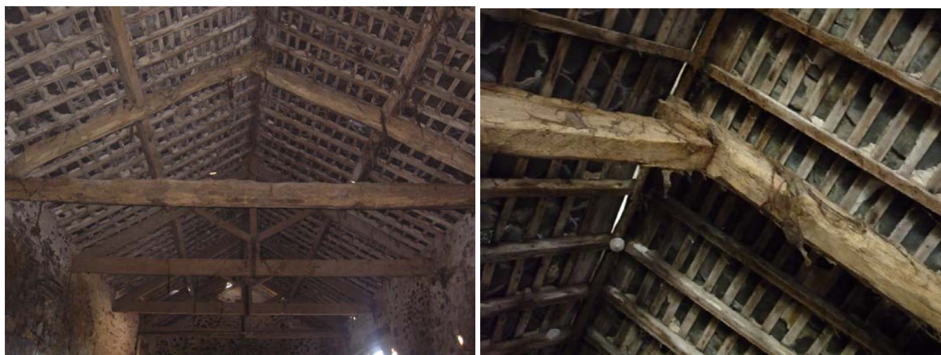
Plate 22 (left): Trusses viewed from the north, Building 1
