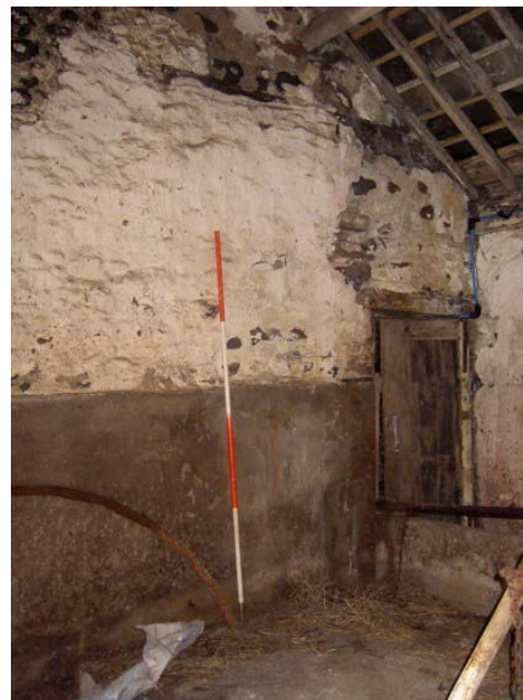
Plate 25 (right): Lintel above the blocked wagon door in south elevation of Building 2
