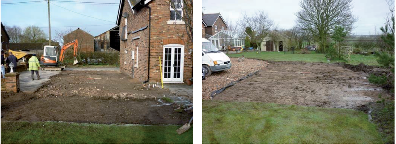
Plate 2 (left): Area A, viewed from the east ahead of the excavation
