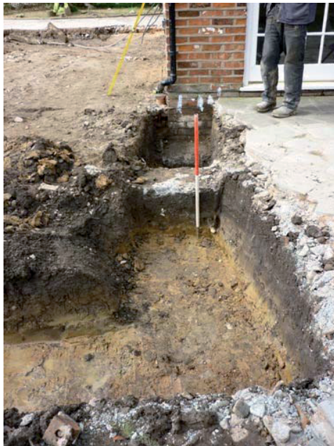
Plate 6 (left): Concrete foundations and deposits above the greyish-yellow clay natural
