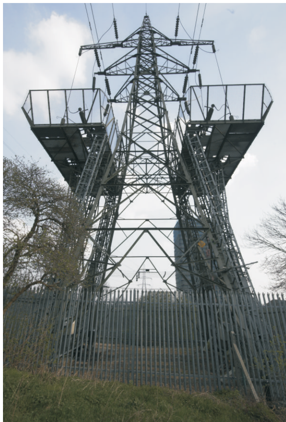
Fig 16 Pylon EDFE113, erected in 1971 with extensions to the upper cross arms. Looking south-east
