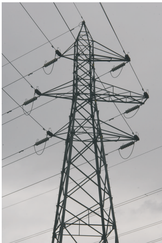
Fig 17 Deviation tower EDFE104, which incorporates shorter cross arms on the north western side. Looking north-east
