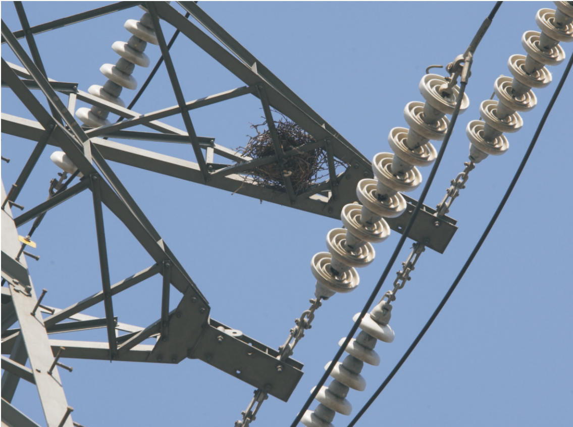
Fig 18 Ceramic insulators on suspension tower EDFE099
