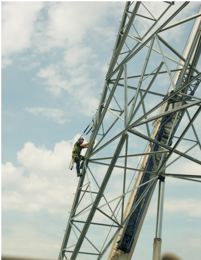
Fig 20 The ladder and harness in use during the erection of a temporary pylon in Temple Mills Lane in June 2007. Looking north
