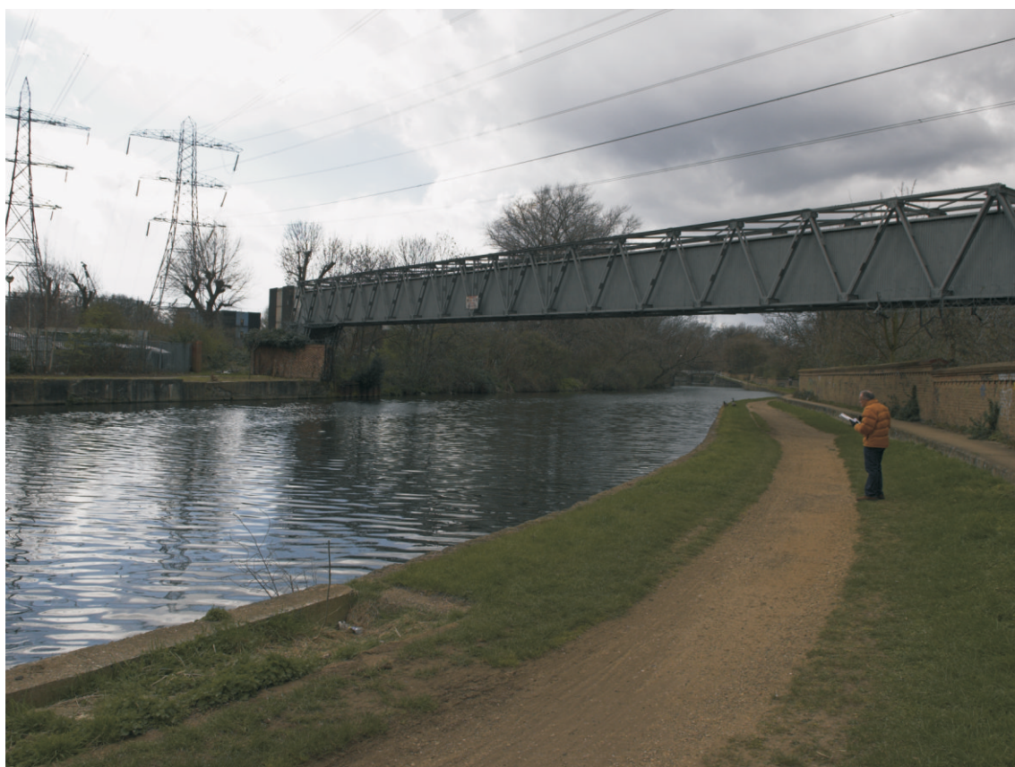
Fig 25 The 132kV power line is carried over the River Lea by a self-contained steel bridge; the line is then buried before resurfacing in the sealing end compound of EDFE095. Looking north-west
