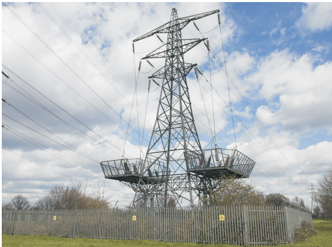
Fig 26 Terminal tower EDFE095 and its sealing end compound on Hackney Marsh. Looking north-east
