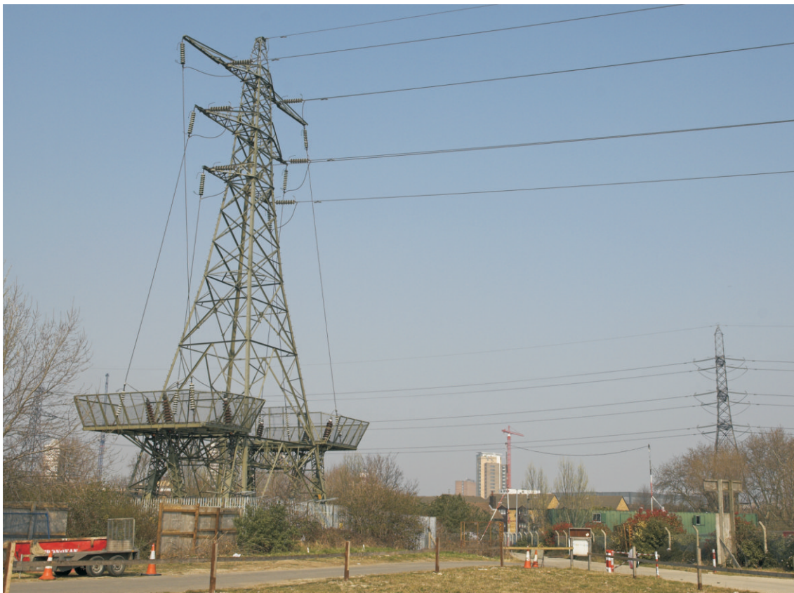
Fig 56 Terminal tower EDFE114, in the grounds of Abbey Mills Pumping Station. Looking north
