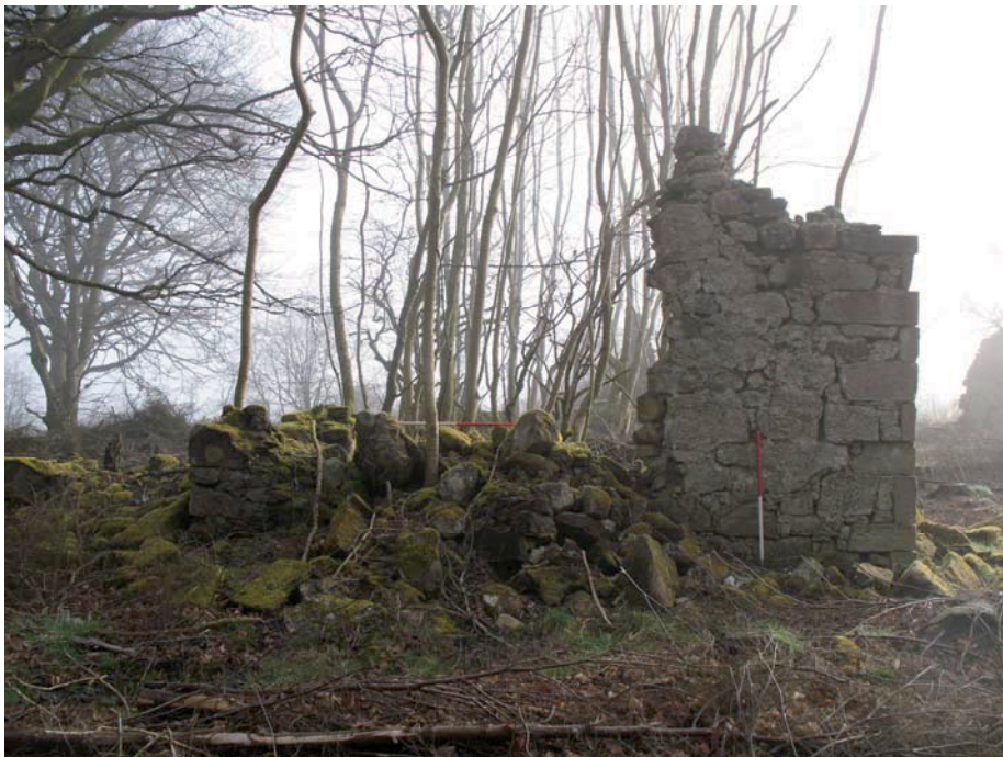
Fig. 16b: Building 202 , W-Facing Elevation
