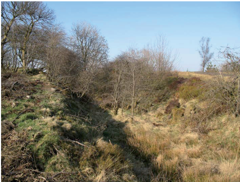
Fig. 14b: Railway Cutting 205 with Field Boundary 204 to left
