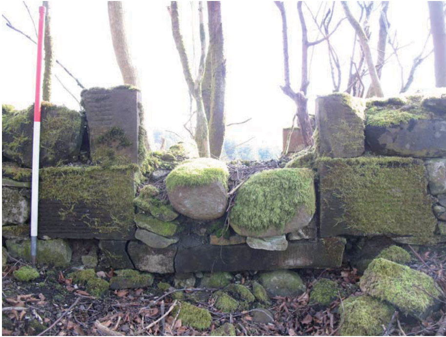
Fig. 17a: Building 202, Blocked Doorway in N-Facing Elevation, W end
