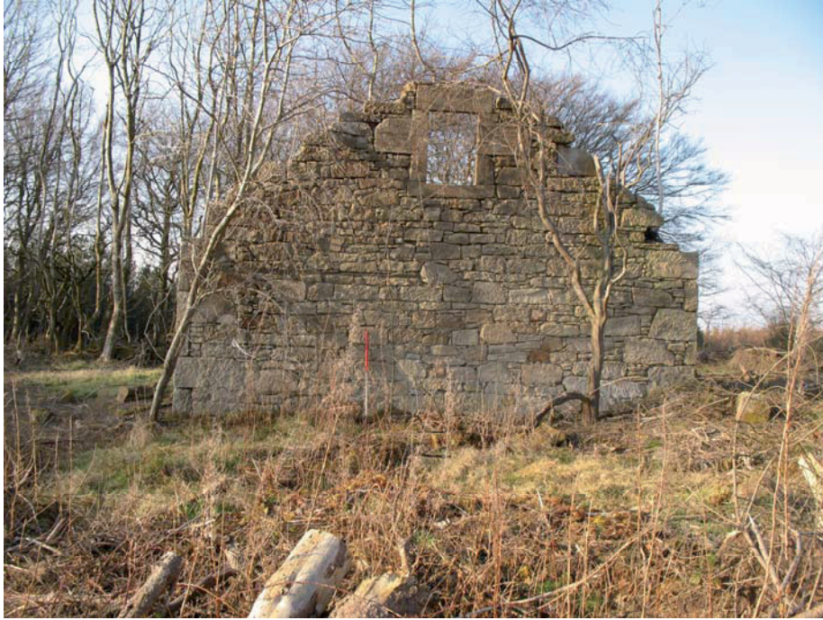
Fig. 16a: Building 201 , S-Facing Elevation
