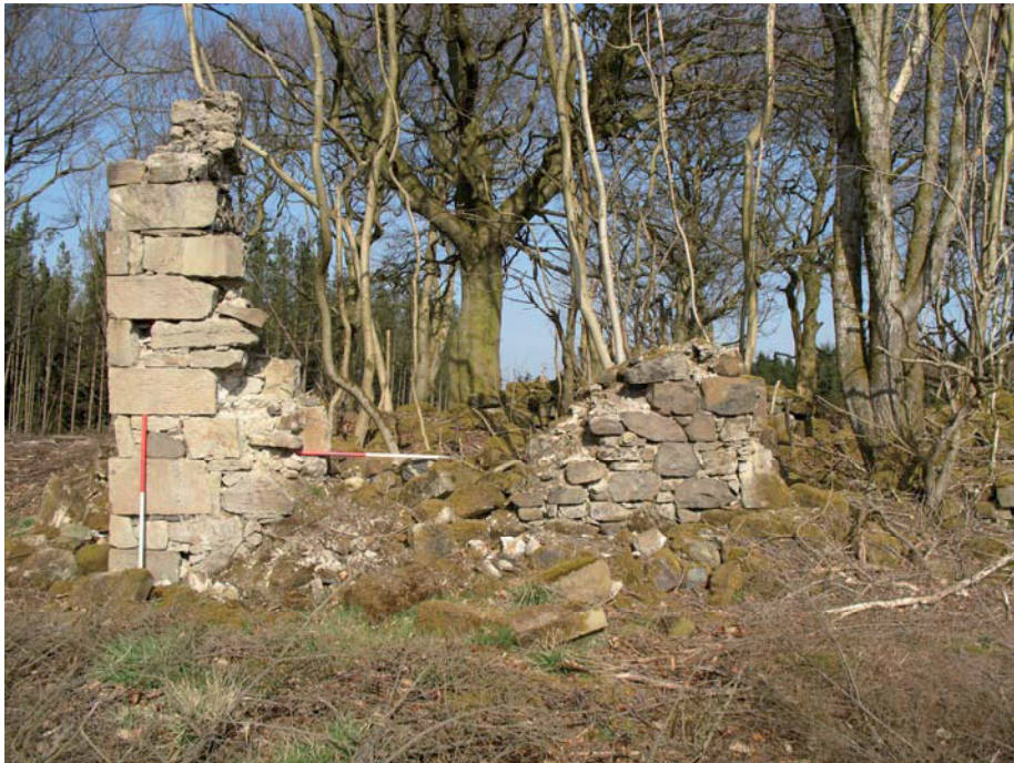
Fig. 17b: Building 202, S-Facing Elevation, W end
