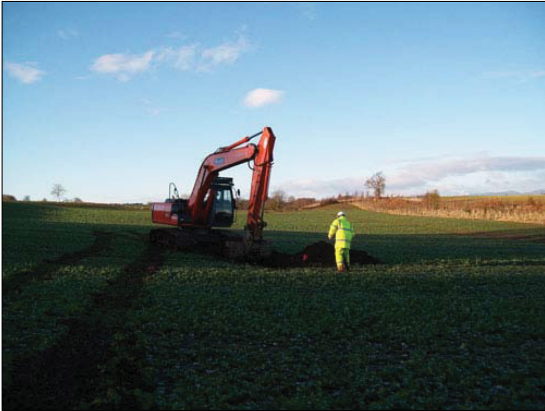
Figure 11a: Excavating in Northern Area
