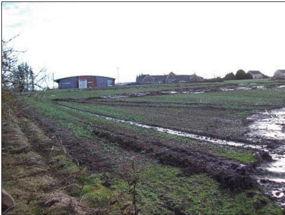
Figure 11b: Western Area backfilled
