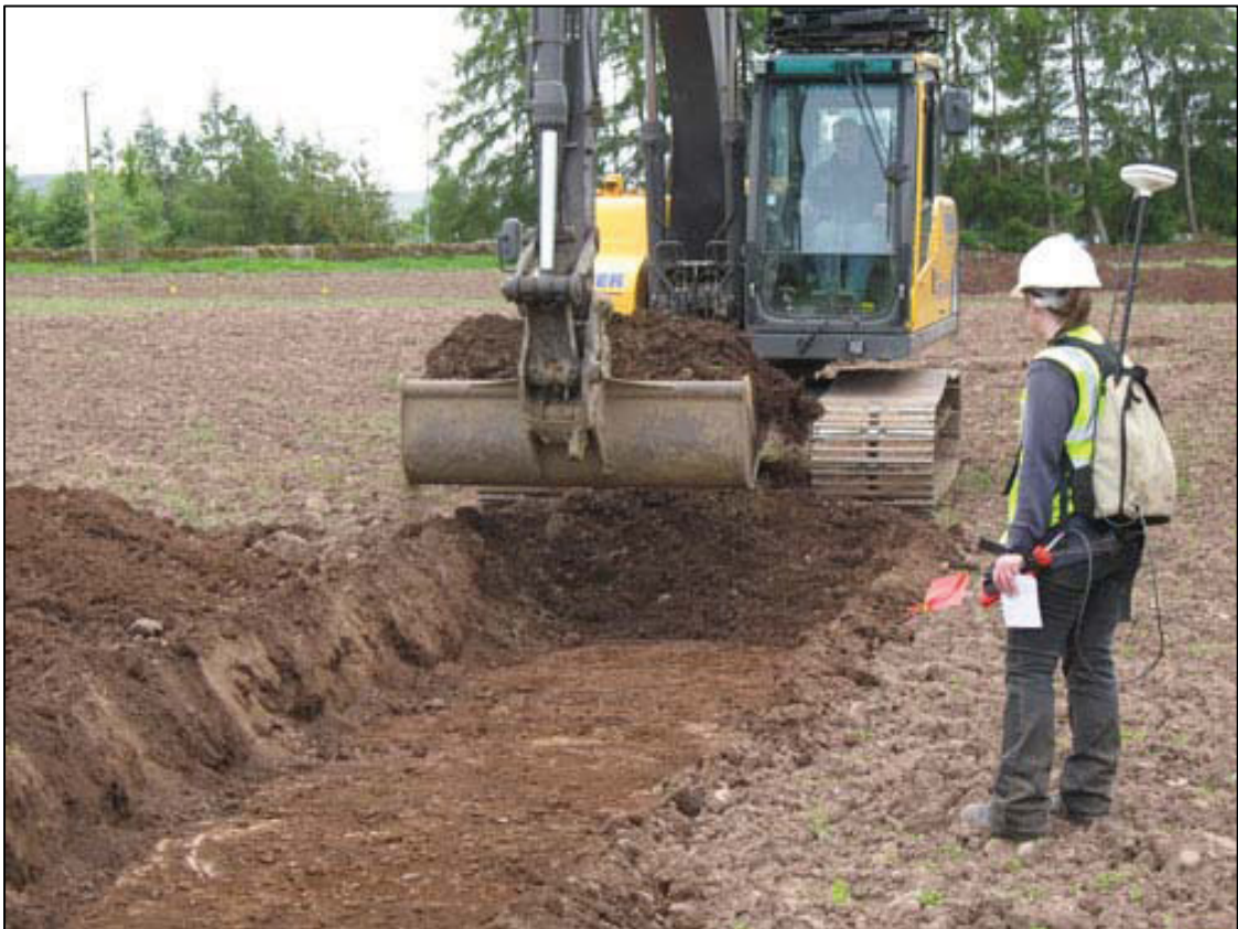
Figure 3b: Excavating trenches
