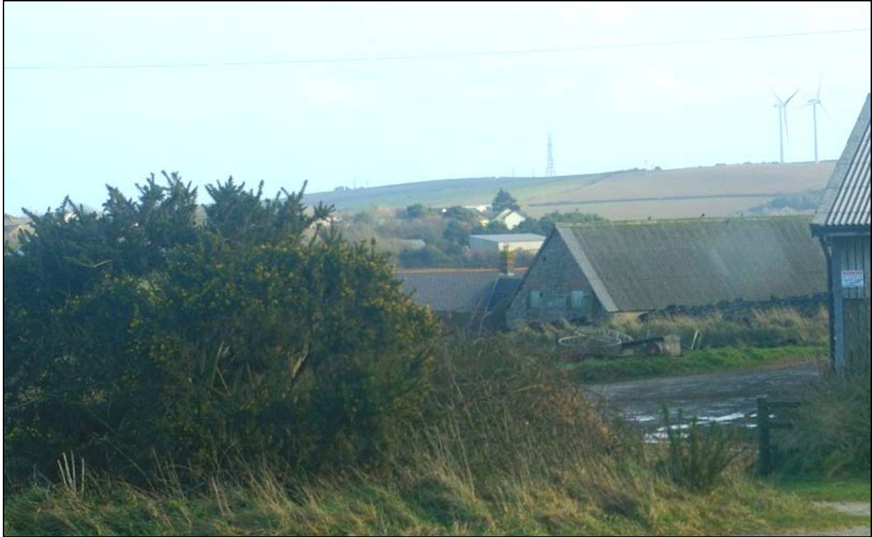
View over the roof of Cargoll barn to the south and showing the turbines at Carland Cross; from the north-west.
