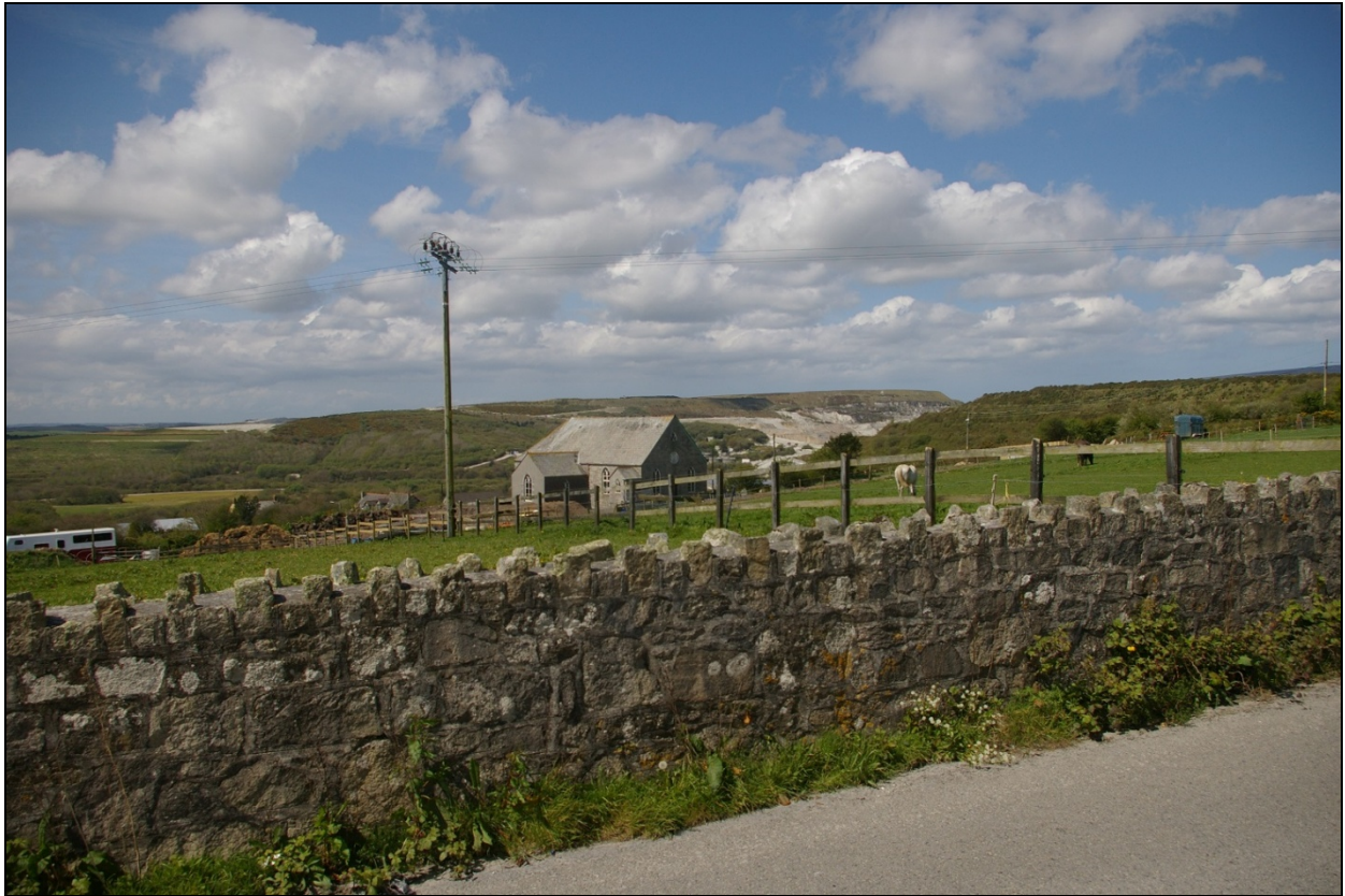
View of the 19 th century school at Trethosa, showing wide views from the general area; from the south-east.
