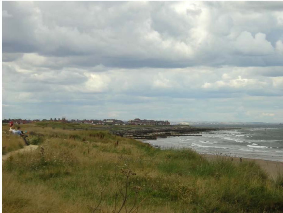
Figure 9.22. Groynes at Marske Sands
