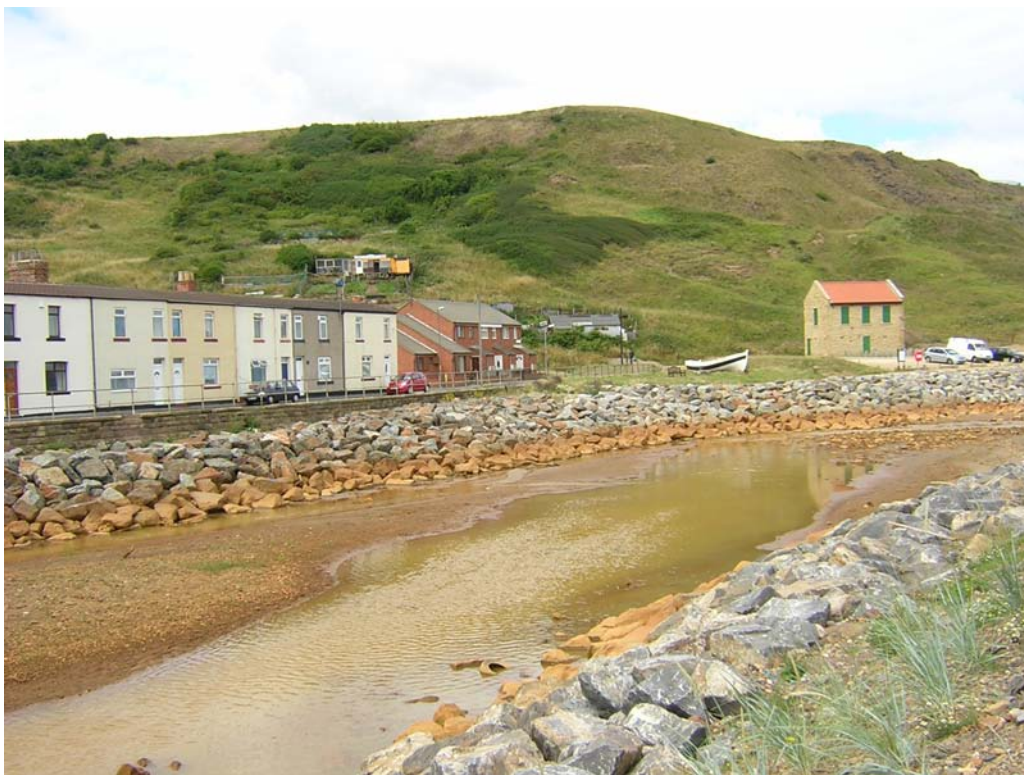
Figure 9.3. Skinningrove Beck discoloured by groundwater from the nearby ironstone mines
