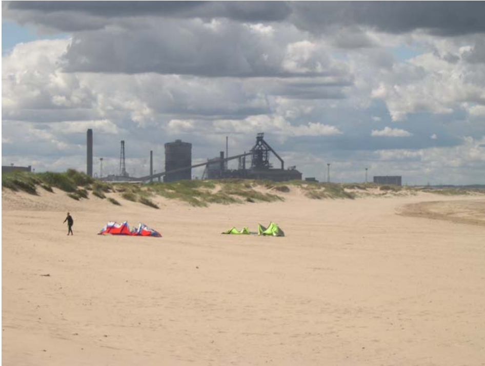
Figure 10.9. Redcar Sands with Teesside Works in the background
