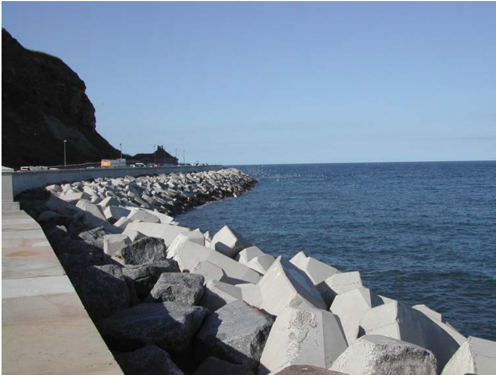
Figure 9.21. Breakwater at Scarborough
