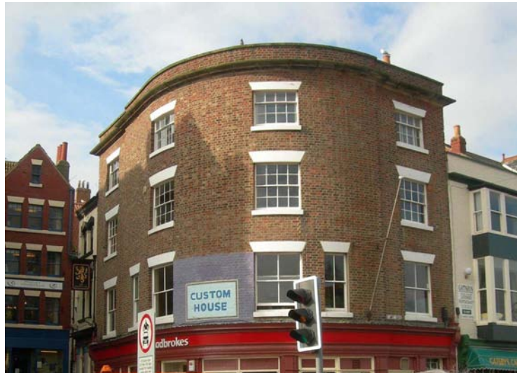
Figure 9.17. Former custom house, Scarborough
