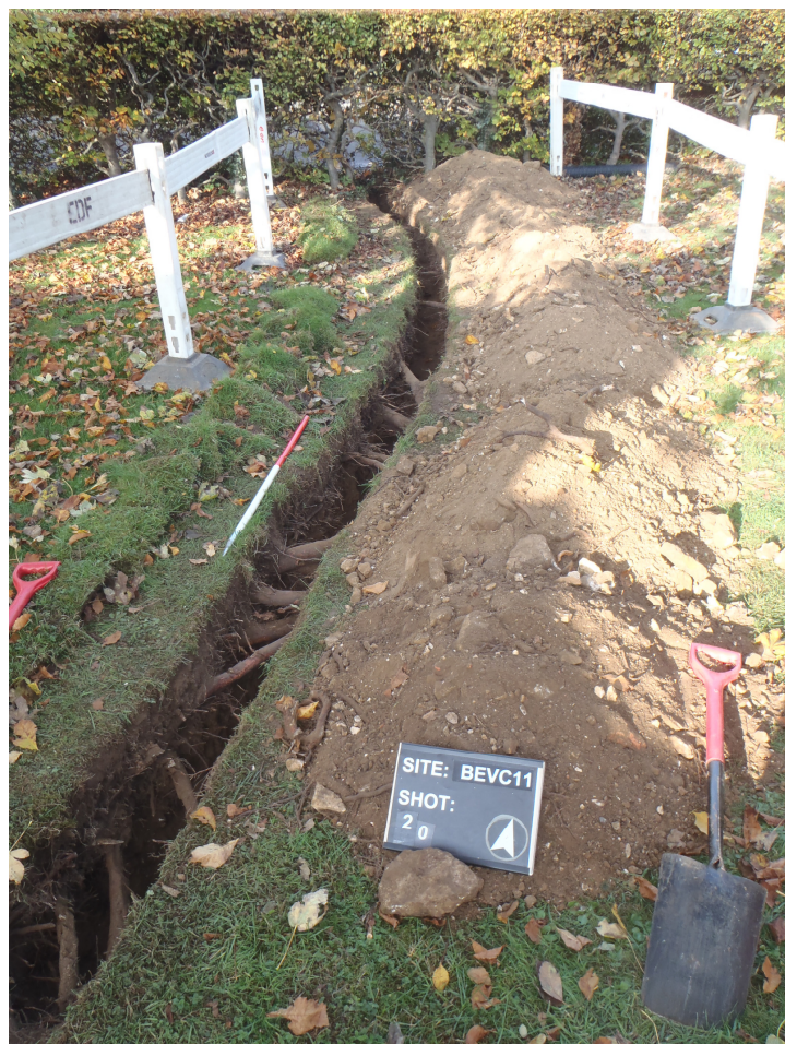
Plate 8: Hand-dug trench with several root systems
