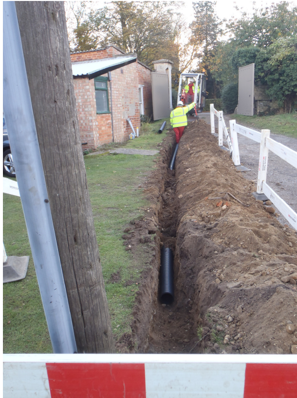
Plate 3: Location of trenching adjacent to Old School house
