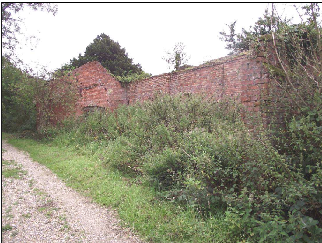
Plate 13 (Shot 33): Cart shed I, looking south, showing roof scar of former mono-pitched roof and brick buttresses
