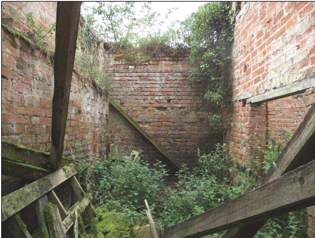
Plate 12 (Shot 26): Overgrown interior of outbuilding H, looking south-west. Note additional brick wall to left of shot with stubs of former floor joists above, and doorway into cart shed I to right of shot
