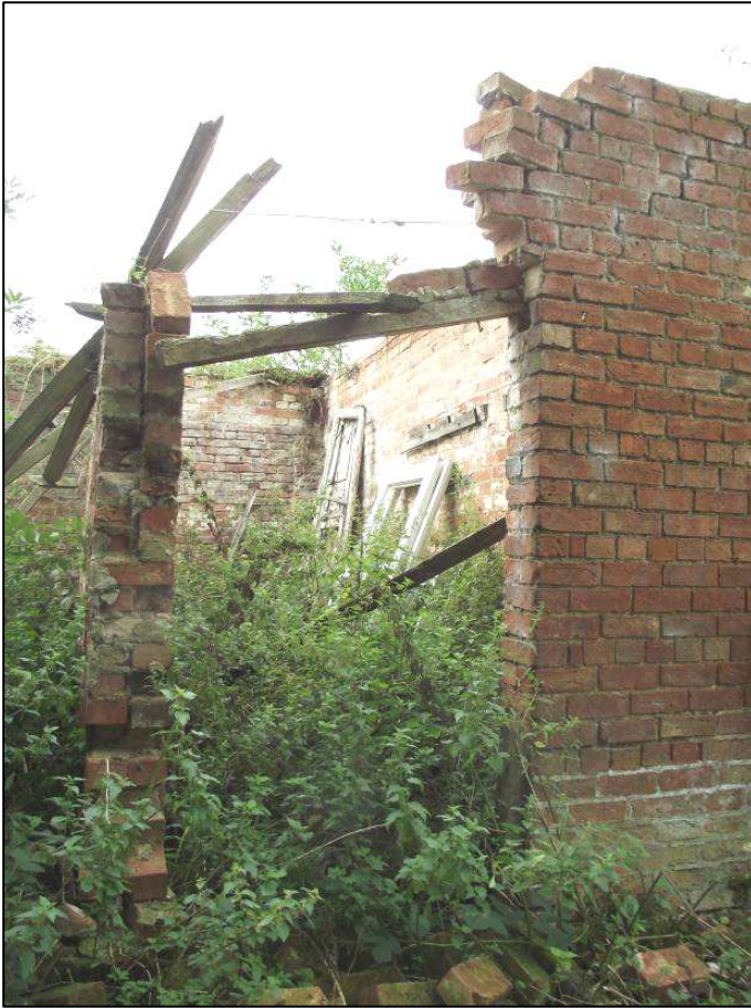
Plate 11 (Shot 25): General view of outbuilding G, looking south-west. Note the surviving brick jamb to the right of the opening indicating a probable former doorway
