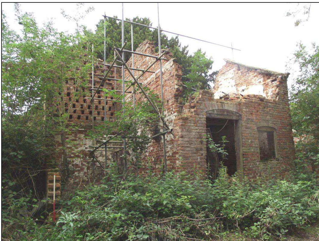
Plate 3 (Shot 9): North-west elevation of dovecote B and outbuilding C, looking south-west, showing nesting holes and perching ledges
