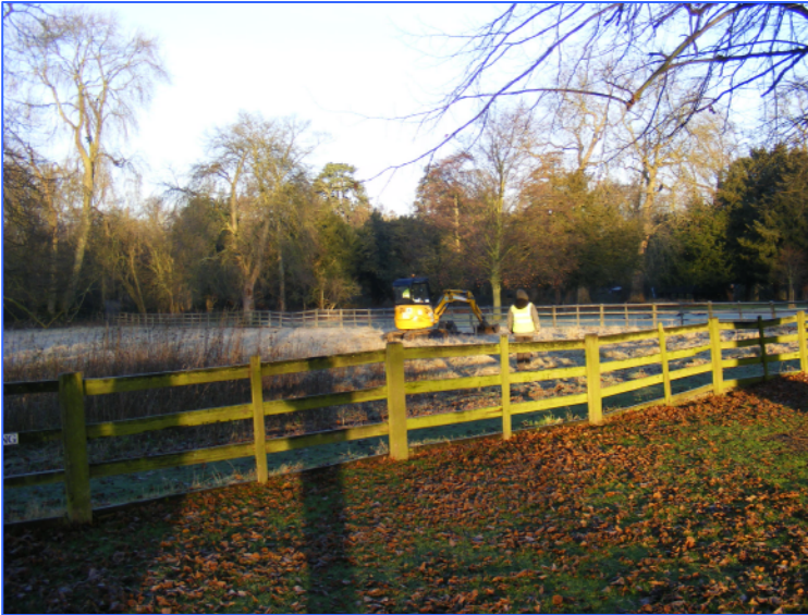
Plate 1: General working shot during excavation of Test Pit 1, looking north-west
