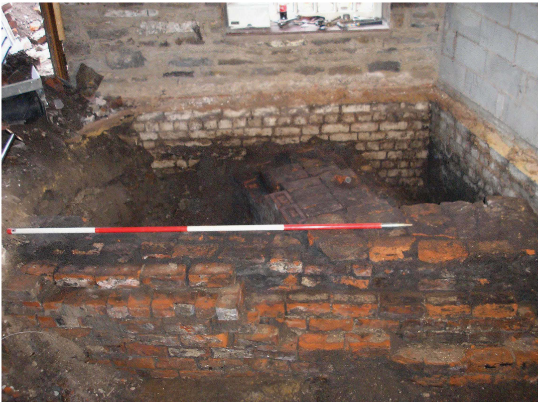
Plate 8: Western wall ( 114 ) of the boiler room
