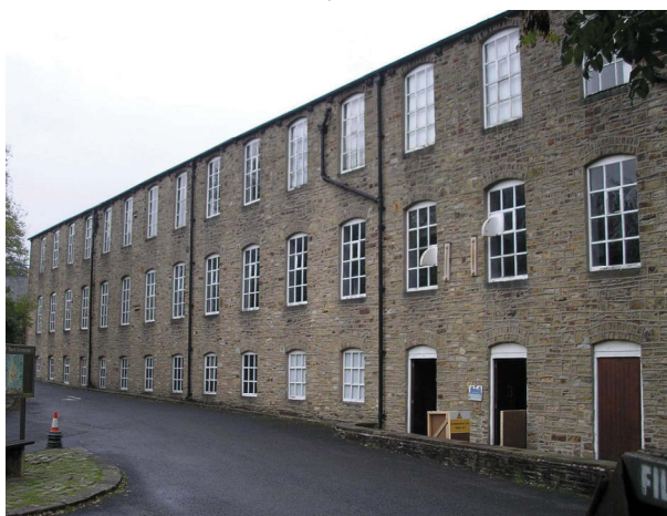
Plate 2: South-west-facing elevation of Whitaker's Mill
