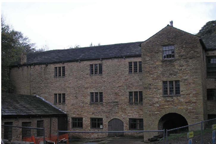
Plate 1: The south-facing elevation of Higher Mill
