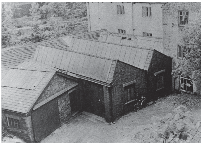
Plate 3: The boiler house (on the left) prior to demolition
