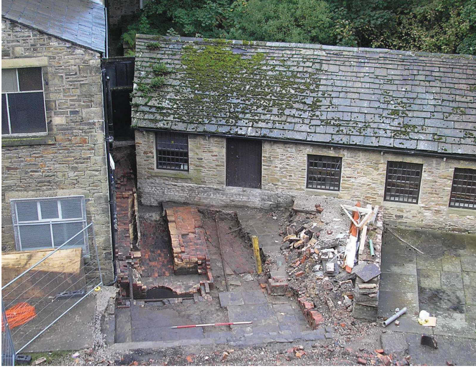
Plate 5: General view of the excavated boiler house, looking west
