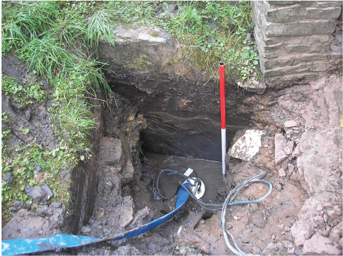
Plate 15: View of the headrace wall in Test Pit 2
