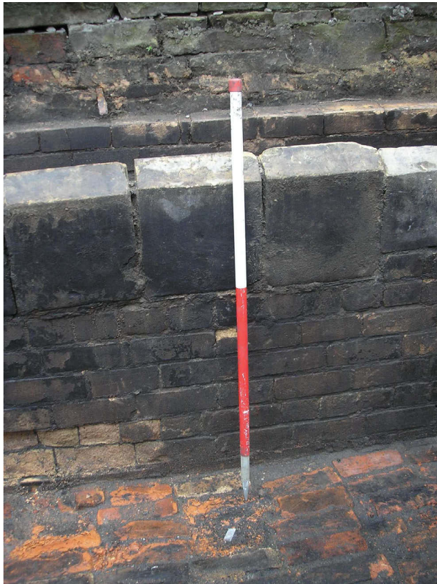
Plate 10: Refractory brick wall below boiler mounts lining the ash pit 107
