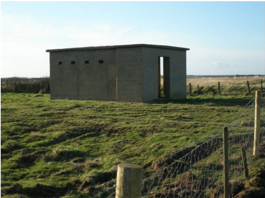
Plate 16 World War 2 structure north-east of Low Farm, Aldbrough
