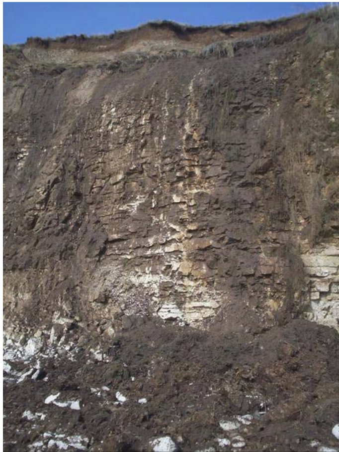
Plate 11 Sewerby cliff, showing recent collapse of till capping
