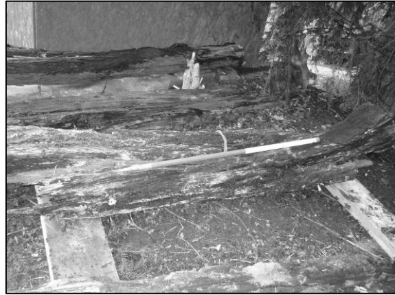
Photo 2/495: Timber 12 - general view.
