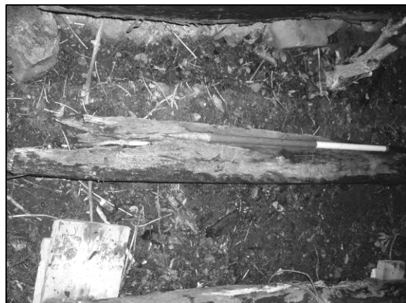
Photo 2/504: Timber 14 - general view.
