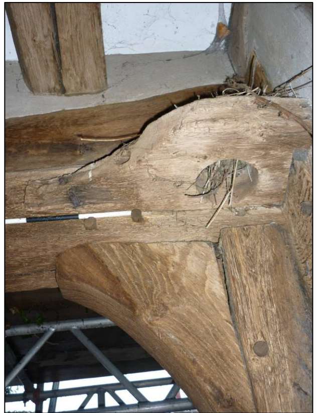
Plate 10: Harr for harr-hung gate over south-west corner of central passage.
