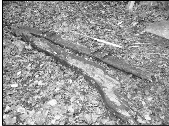
Photo 2/453: Timbers 1 & 2 - general view.
