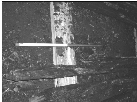
Photo 2/484: Timber 8 - general view.
