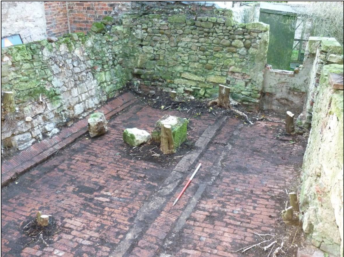
Plate 12: West cell of gatehouse after clearance, looking south-west.
