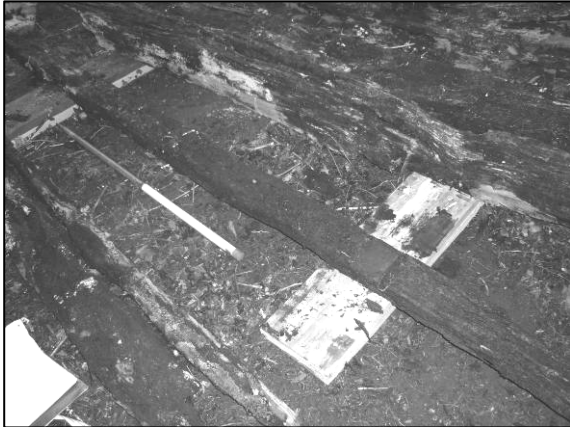
Photo 2/482: Timber 7 - general view.
