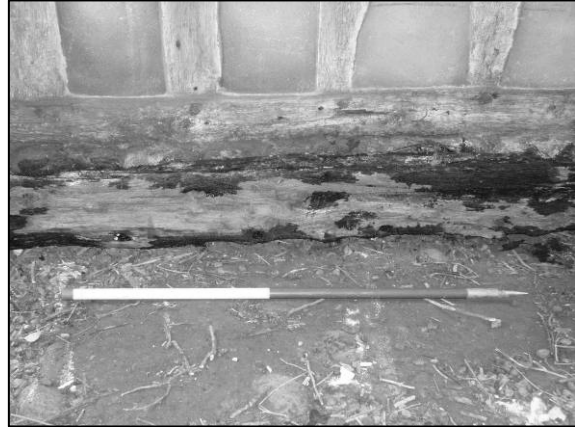
Photo 2/457: Timber 3 - detail of mortices.
