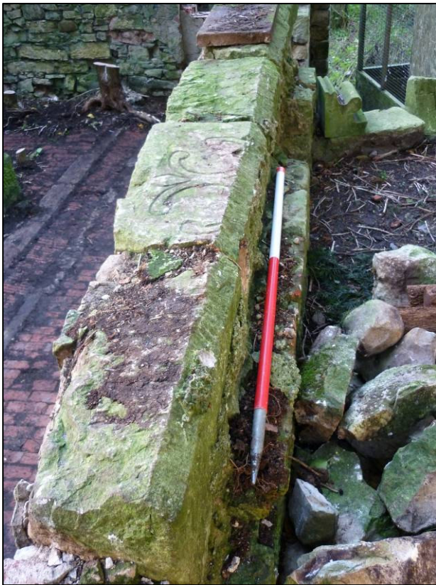
Plate 9: Reused grave slab on chamfered north wall of west cell of gatehouse, looking south-west.
