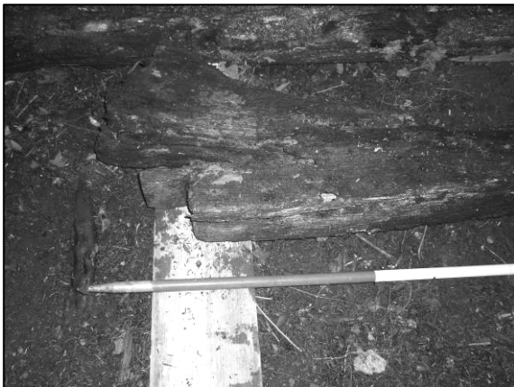
Photo 2/498: Timber 12 - detail of joint.
