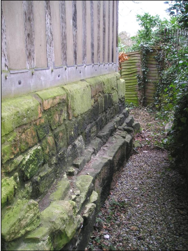
Plate 7: Chamfered plinth, east end of gatehouse, looking north.
