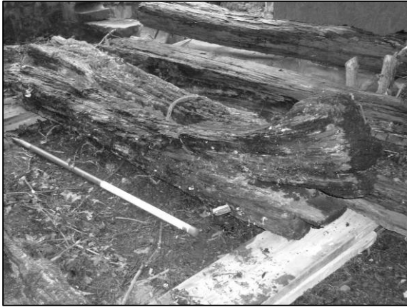
Photo 2/494: Timber 12 - general view.
