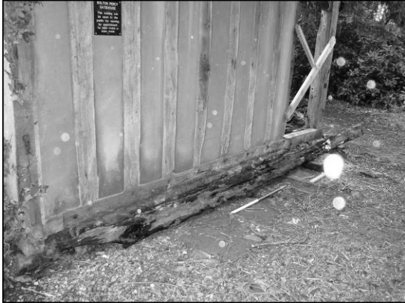
Photo 2/456: Timber 3 - general view.
