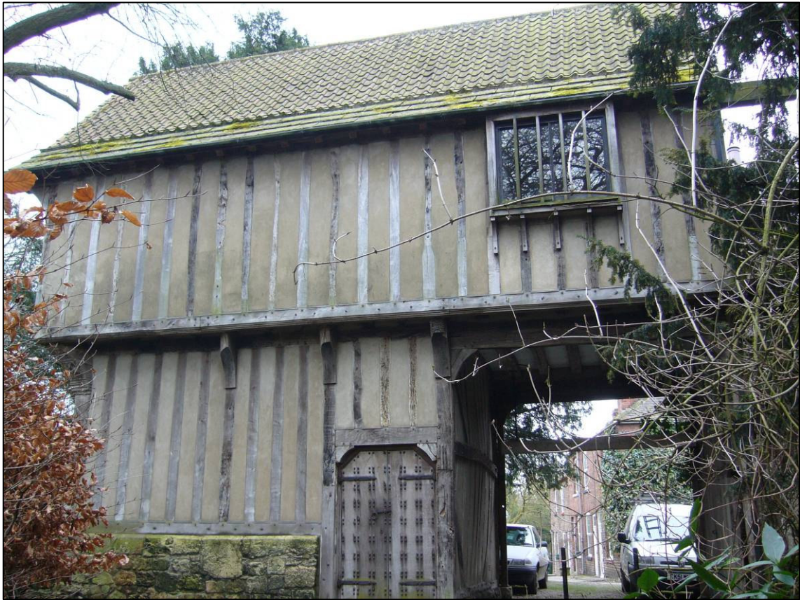
Plate 5: North elevation of gatehouse prior to repairs, looking south-east.
