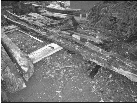
Photo 2/490: Timber 11 - general view.
