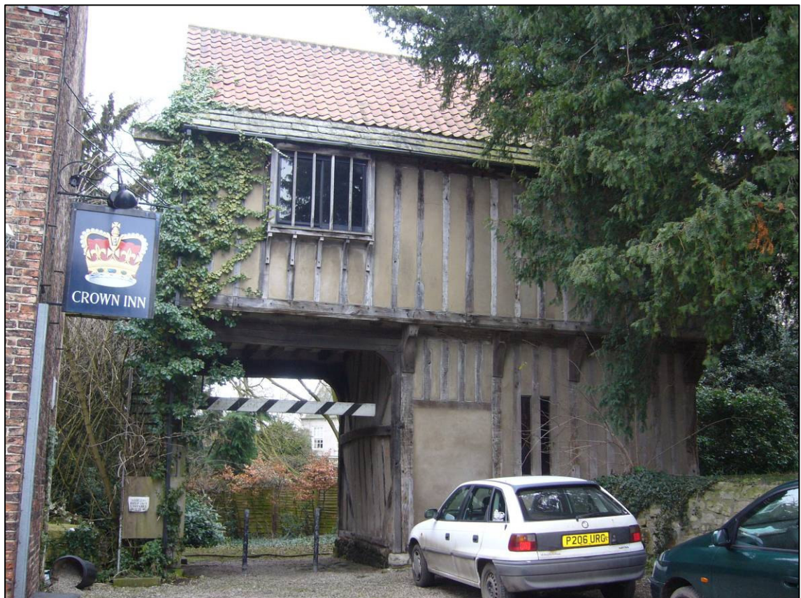
Plate 6: South elevation of gatehouse prior to repairs, looking north-west.
