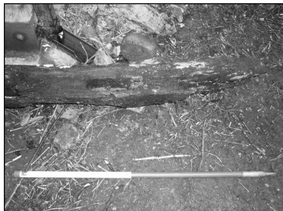
Photo 2/464: Timber 3 - detail of mortices.
