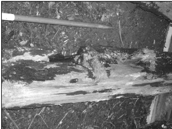
Photo 2/492: Timber 9 - detail of mortice and peg hole.
