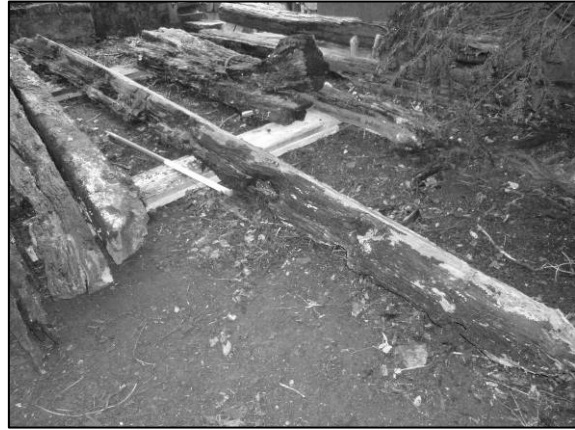
Photo 2/491: Timber 11 - general view.
