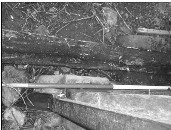
Photo 2/459: Timber 3 - detail of mortices.
