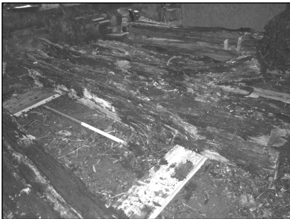
Photo 2/483: Timber 8 - general view.
