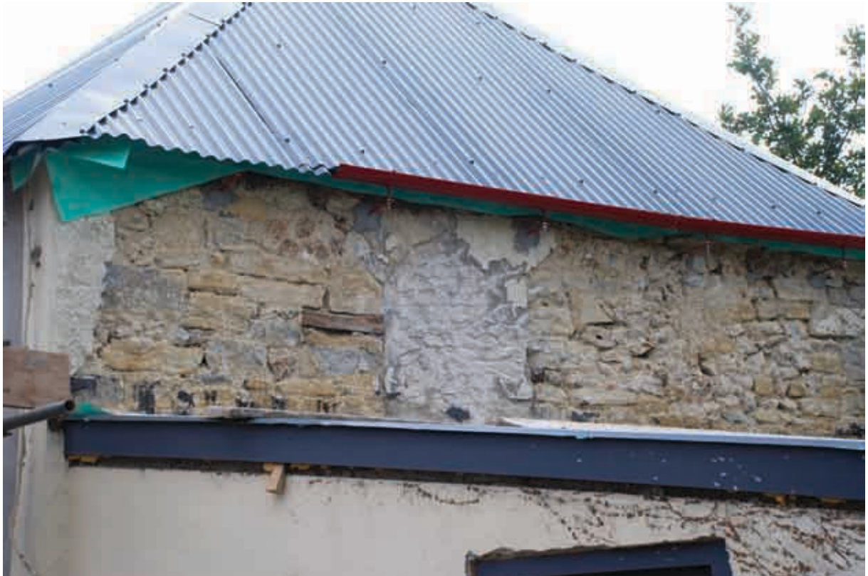
Plate 6 The blocked gallery doorway visible above the lean-to roof, looking south.
