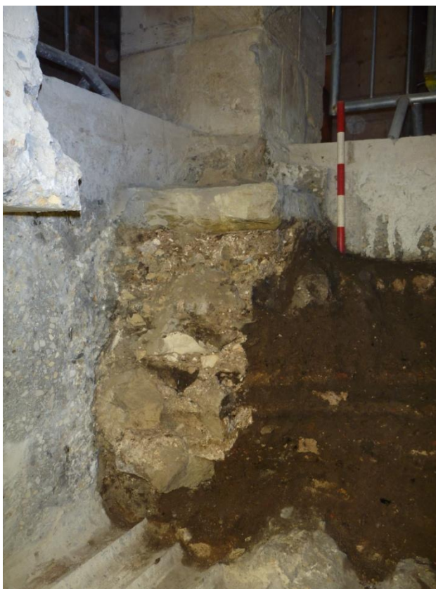
Plate 24 Northern C19th crypt pier foundation 6002, looking ENE
