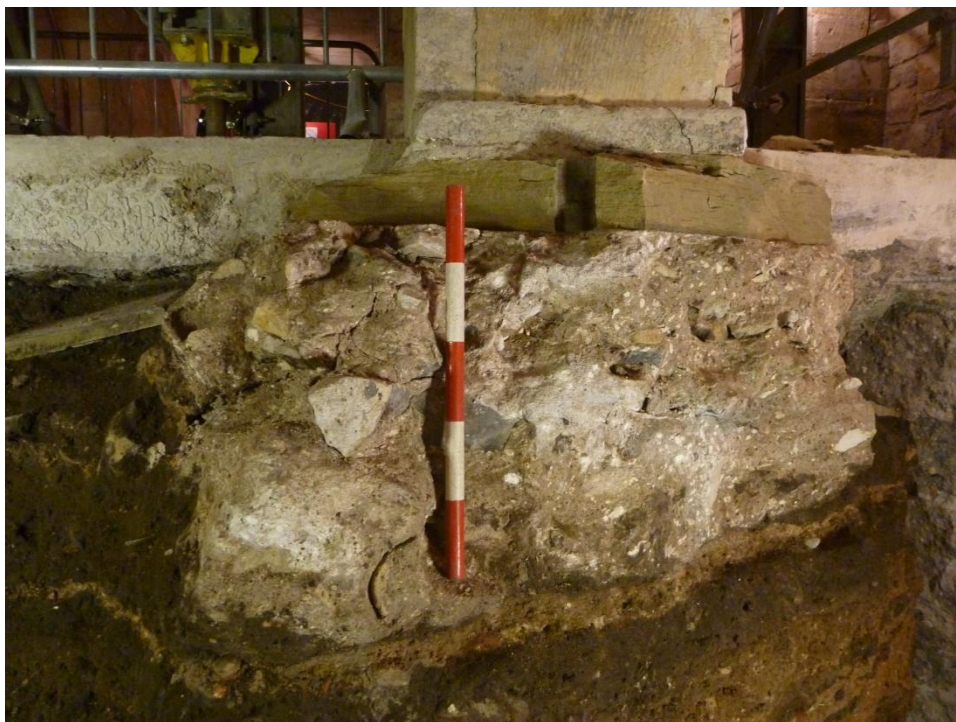
Plate 23 Phase 7 Southern C19th crypt pier foundation 6001, looking east
