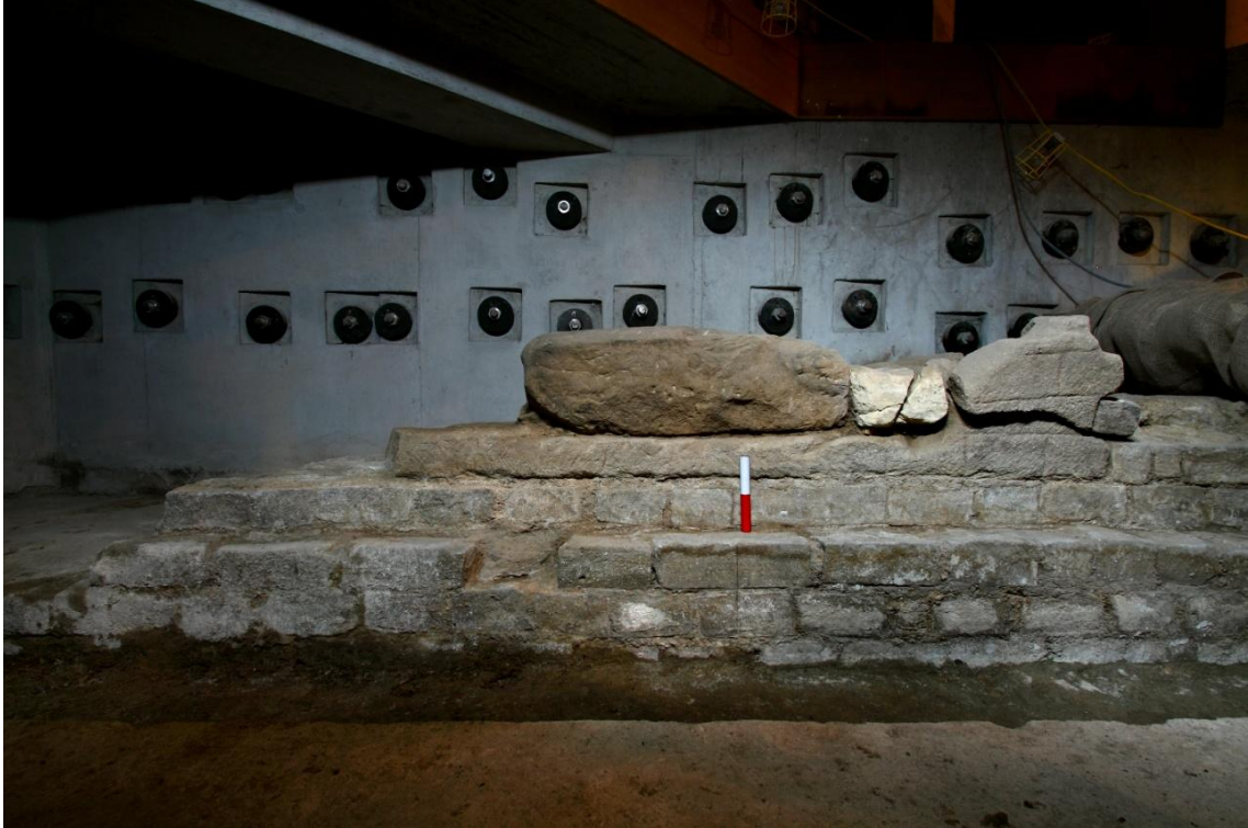
Plate 27 Basilica wall in 2012, east facing elevation. Note fracture of block WC29, numbered 6053 (base) and 6040 (top section) in 2012, in comparison with Plate 26
