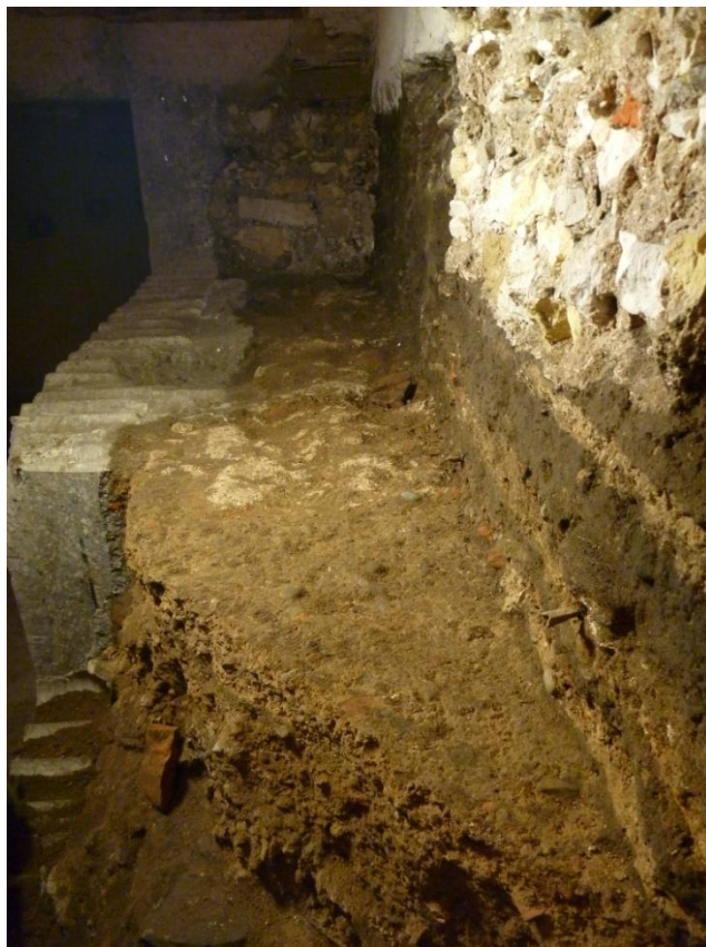
Plate 20 Demolition spread 6013, looking north
