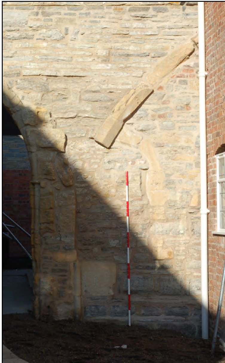
Plate 20: Line of vault arch within south flanking range
