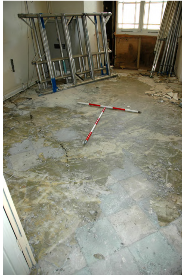
Plate 64: 18 th century lias and limestone floors, covered and varnished in the 20 th century
