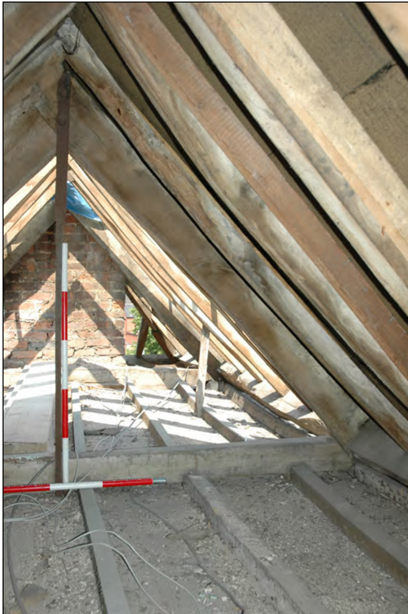
Plate 28: White washed rafters in roof space
