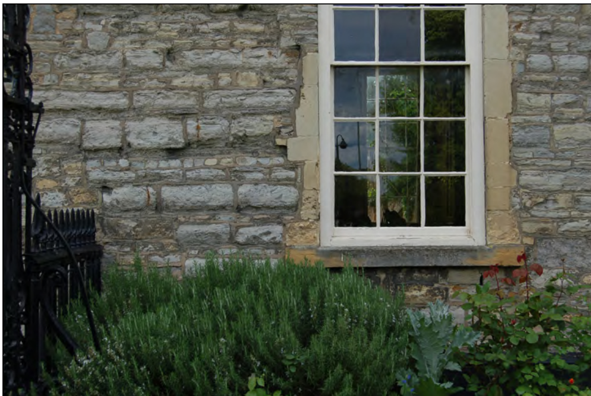
Plate 3: Wide and narrow coursing on front elevation of Abbey Gate
