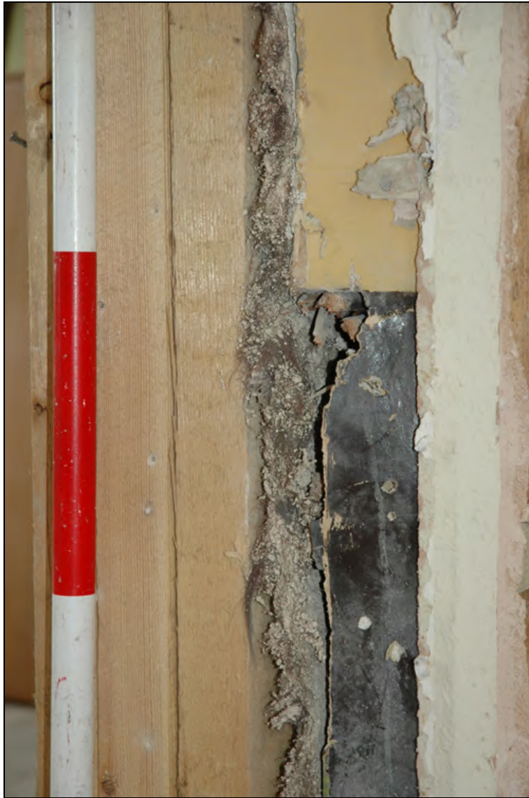
Plate 29: Example of lime plaster partition (modern timber on left)
