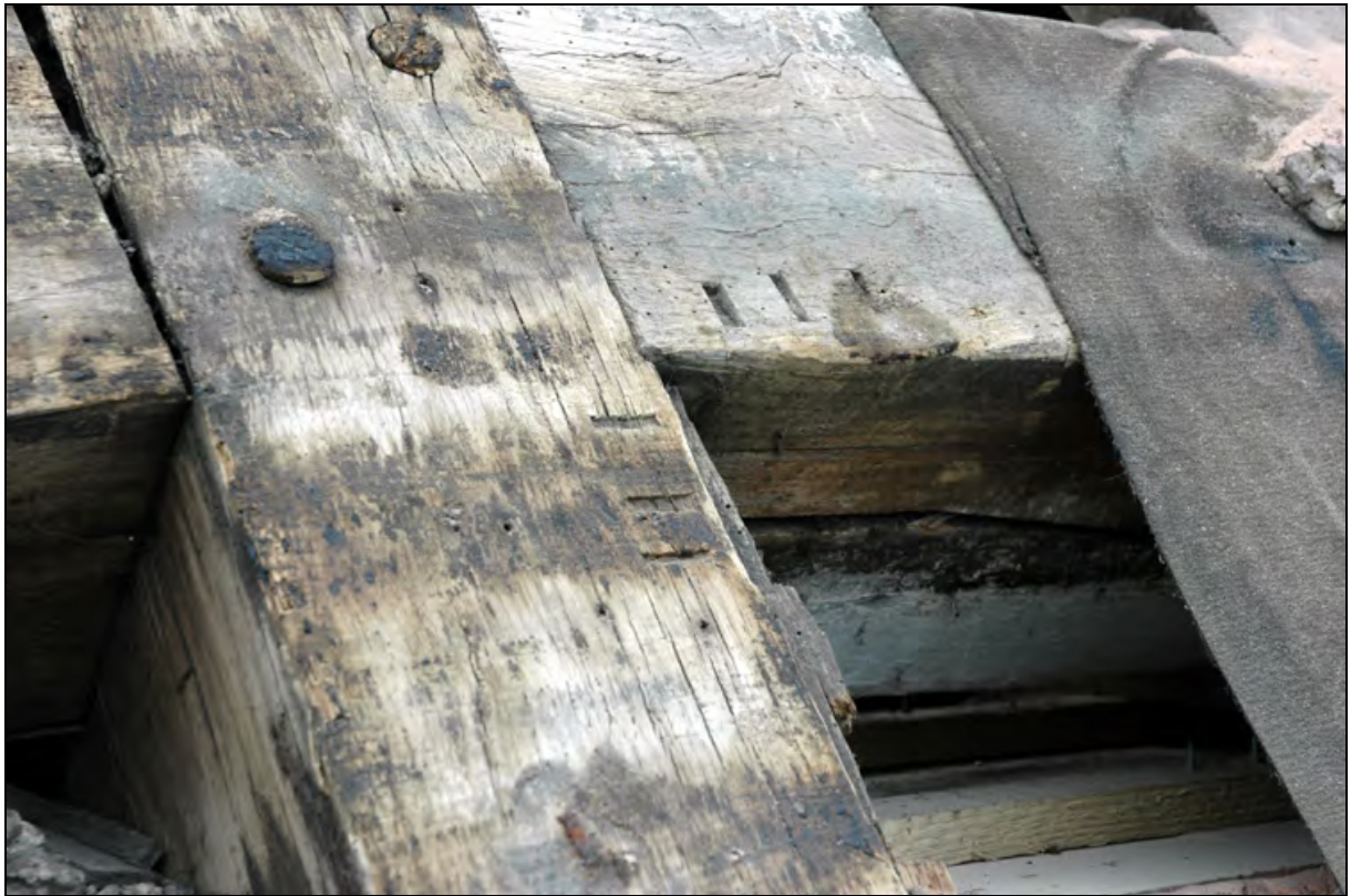
Plate 27: Example of 17 th century carpenters marks on a purlin and principal rafter
