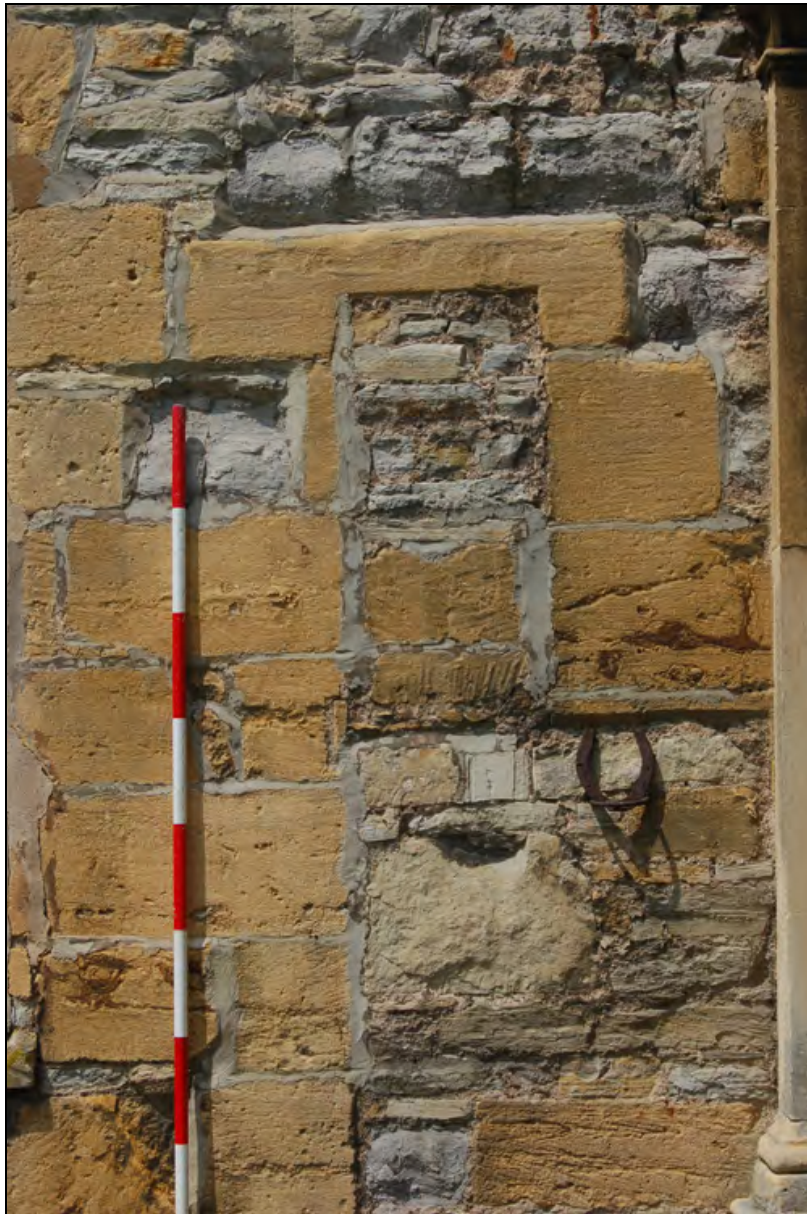
Plate 6: Abbey Gate rear (east) elevation showing possible window opening
