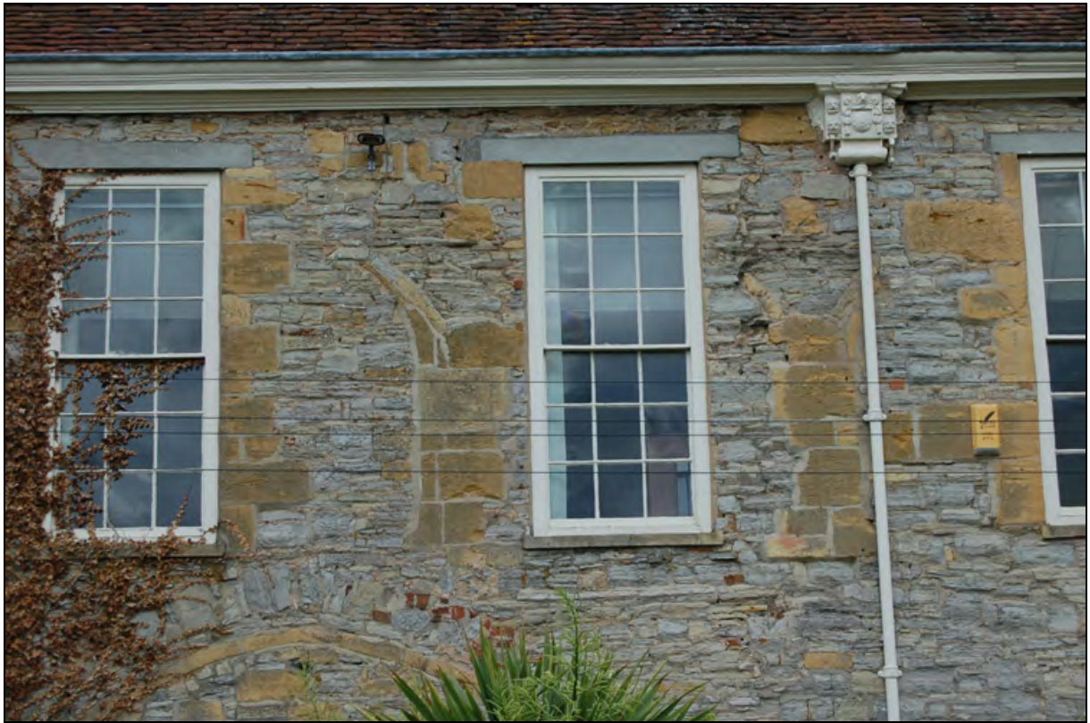
Plate 5: Abbey Gate rear (east) elevation showing probable blind arcading
