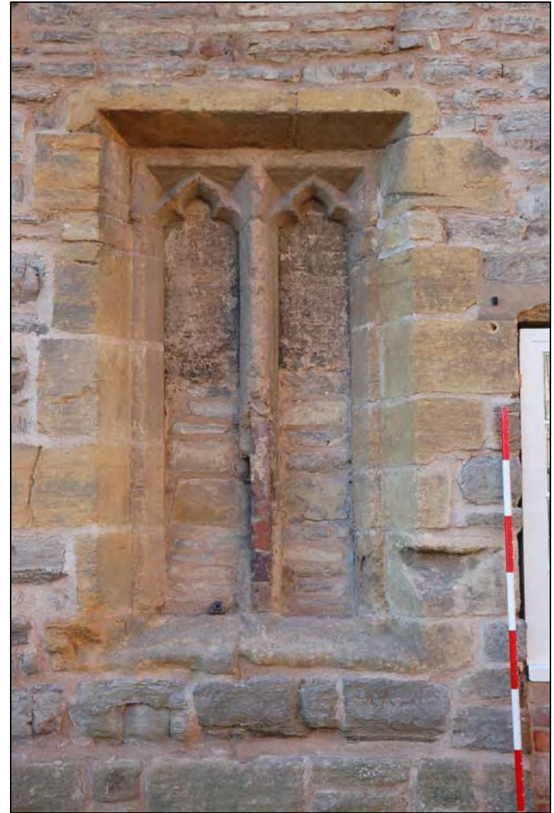
Plate 23: 15 th century inserted window in north wall of 'Abbots Stables'
