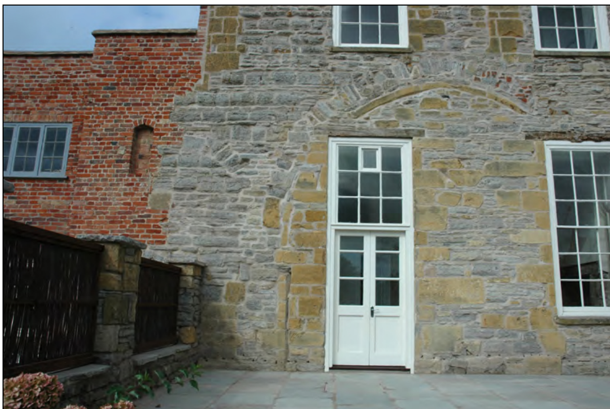
Plate 4: Rear (east) elevation of Abbey Gate showing original gate arch
