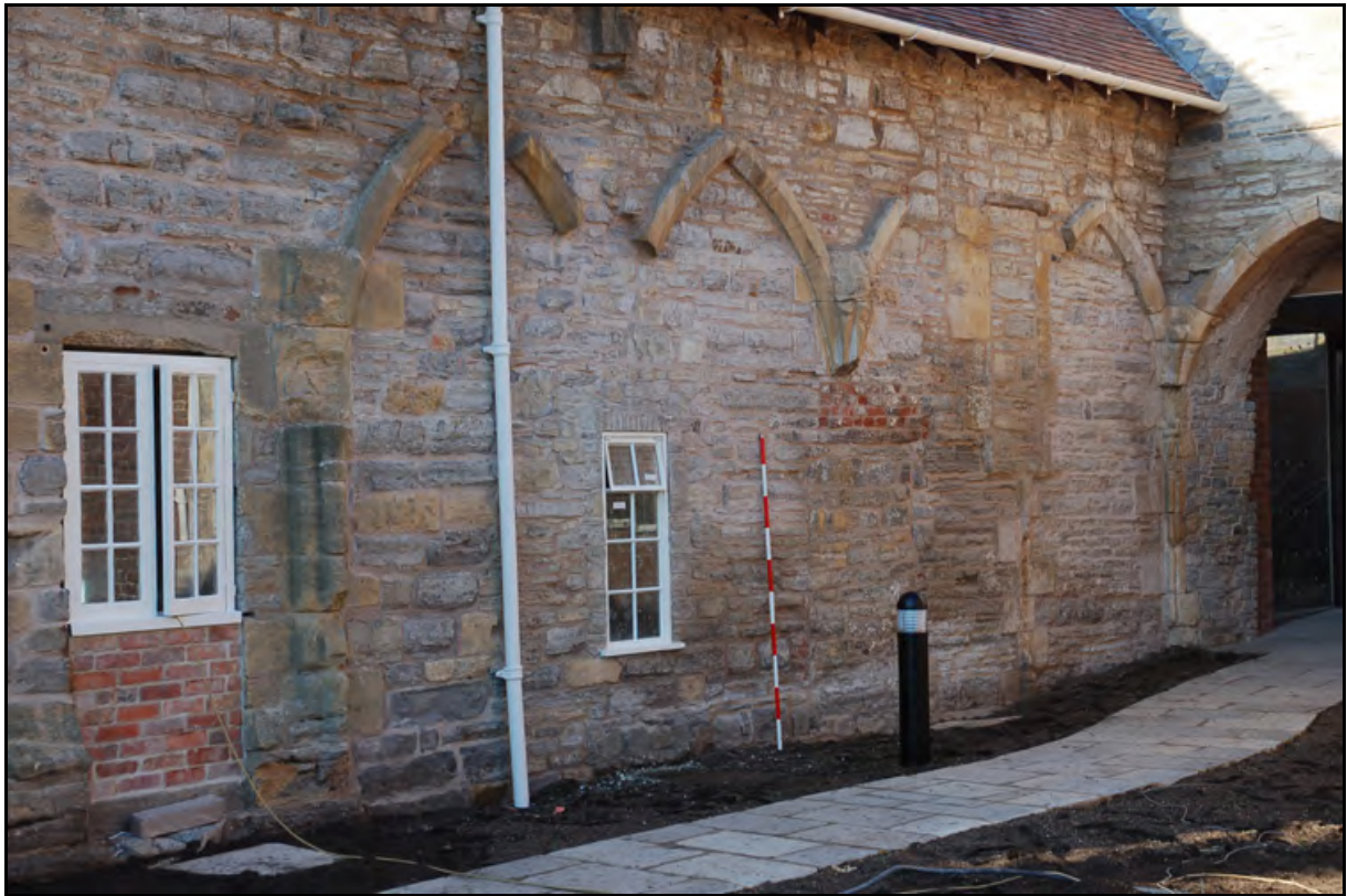
Plate 17: North wall of 'Abbots Stables' showing passageway columns and vault springers
