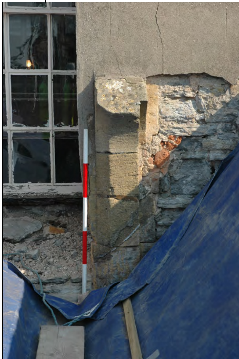
Plate 7: Abbey Gate south elevation showing arch springer
