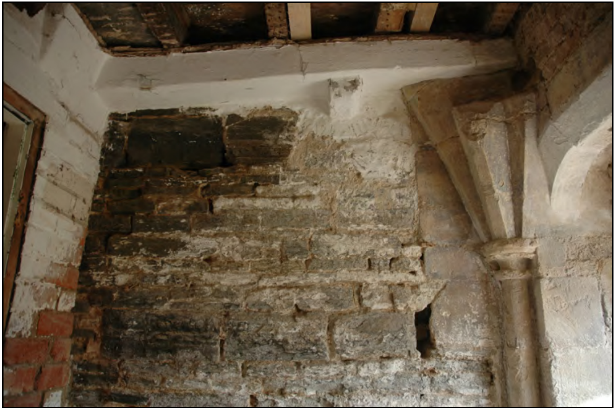
Plate 15: Column and vault springer for south flanking range
