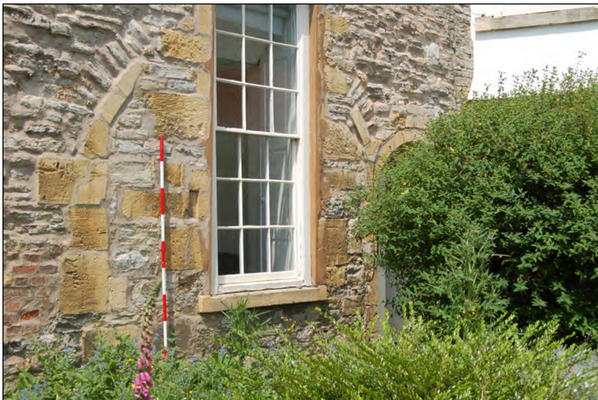
Plate 9: Abbey Gate rear (east) elevation showing blocked opening, possible window
