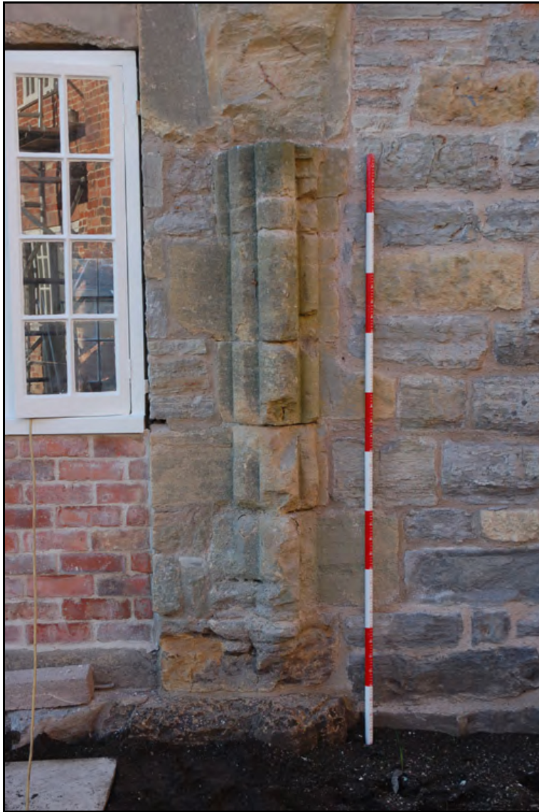
Plate 18: Column of vault springer (right) and gate jamb (left)
