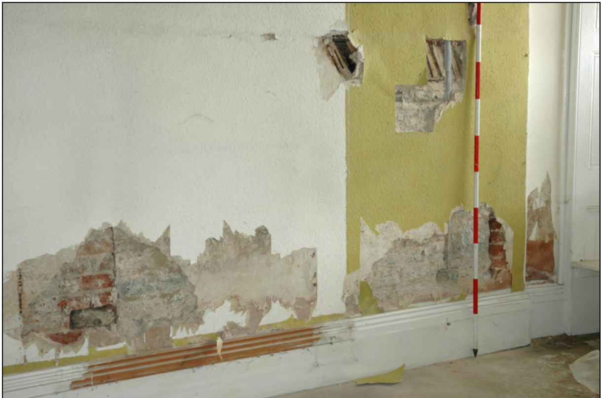
Plate 42: Early 18 th century fireplace (now blocked). The lintel has been covered with laths and the brick sides are visible at each side of the image
