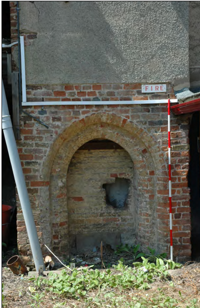
Plate 48: Brick arch copying 14 th century arch on opposite side of building
