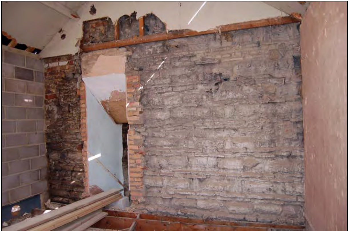
Plate 11: 'Abbots Stables' west elevation showing wide and narrow coursing
