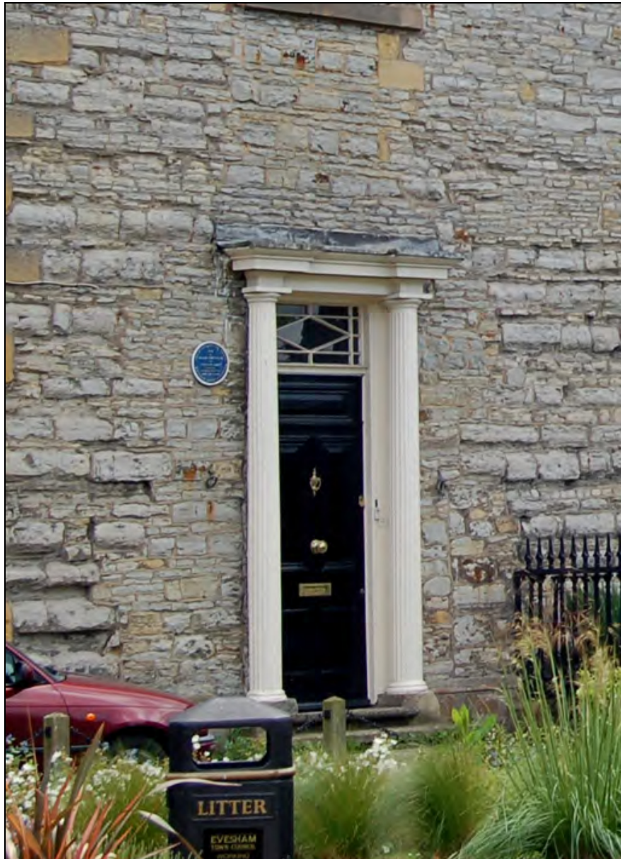
Plate 8: Abbey Gate front elevation showing blocked opening (change of coursing around door)
