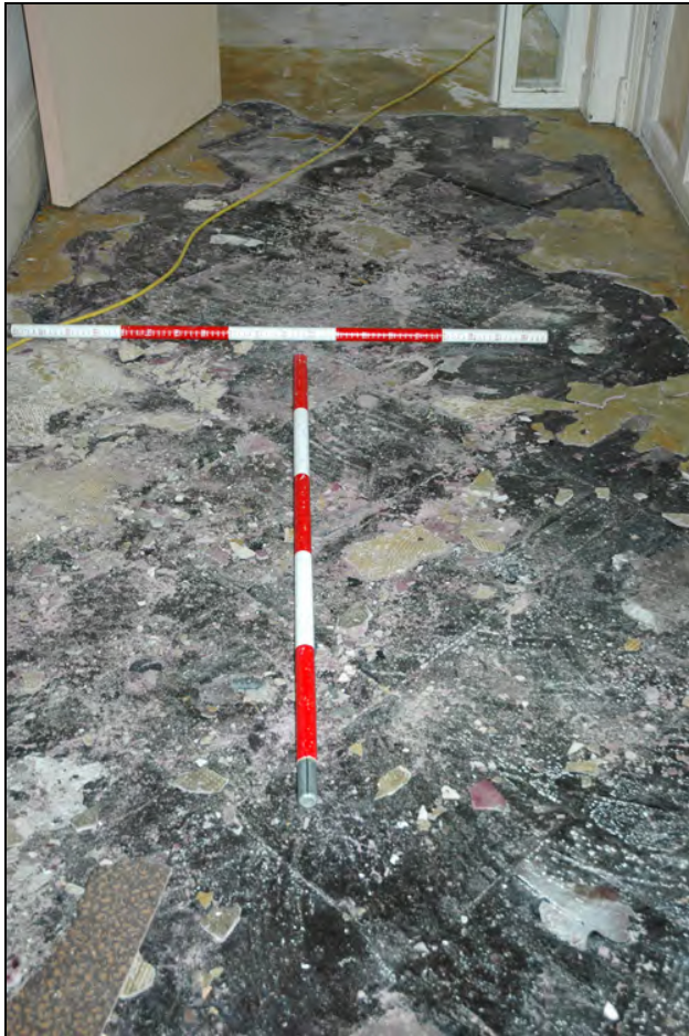
Plate 64: 18 th century lias and limestone floors, covered and varnished in the 20 th century
