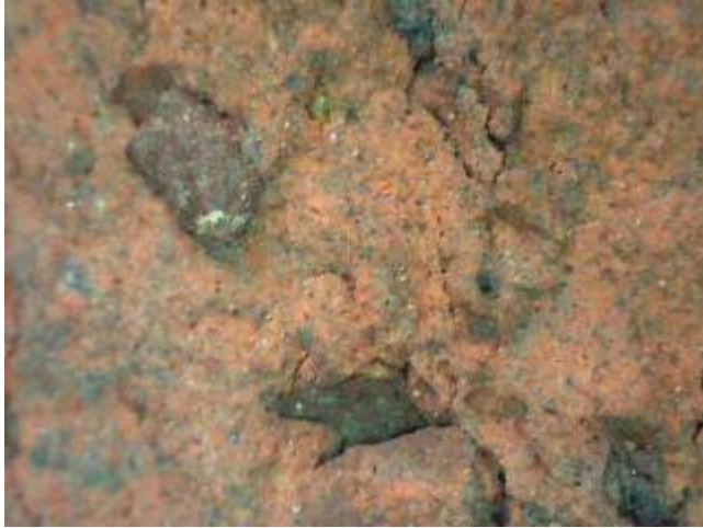
Figure 4 close-up of chimney pot fabric showing ironstone inclusions
