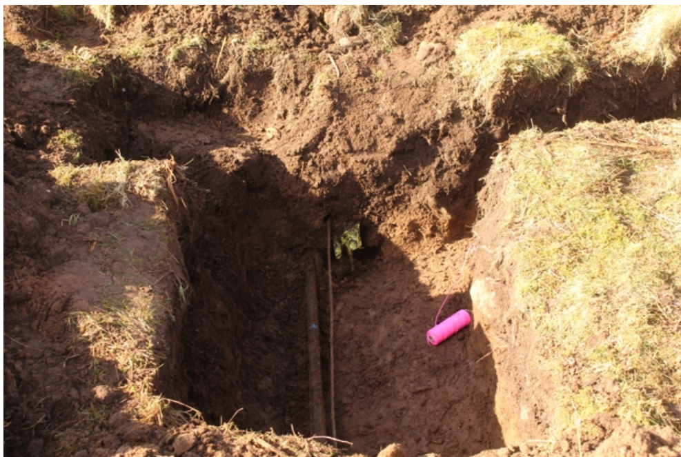
Illustration 8 Milquhanzie Hill, Crieff, Modern Cable Trench [003] showing Cables, (002) and (005)
