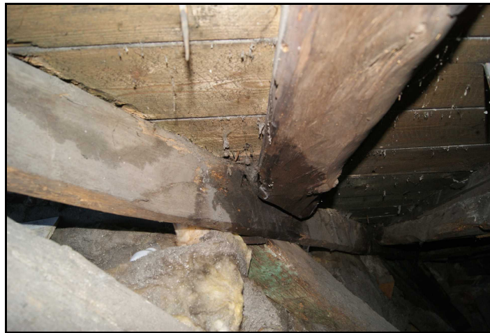
Photo valley timber 23B and rafter 21B
