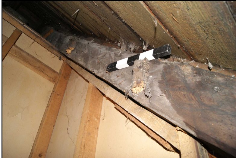
Photo of studs nailed to rafter 17A
