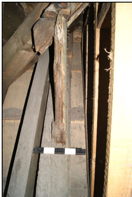
Photo of stud nailed to rafter 4B
