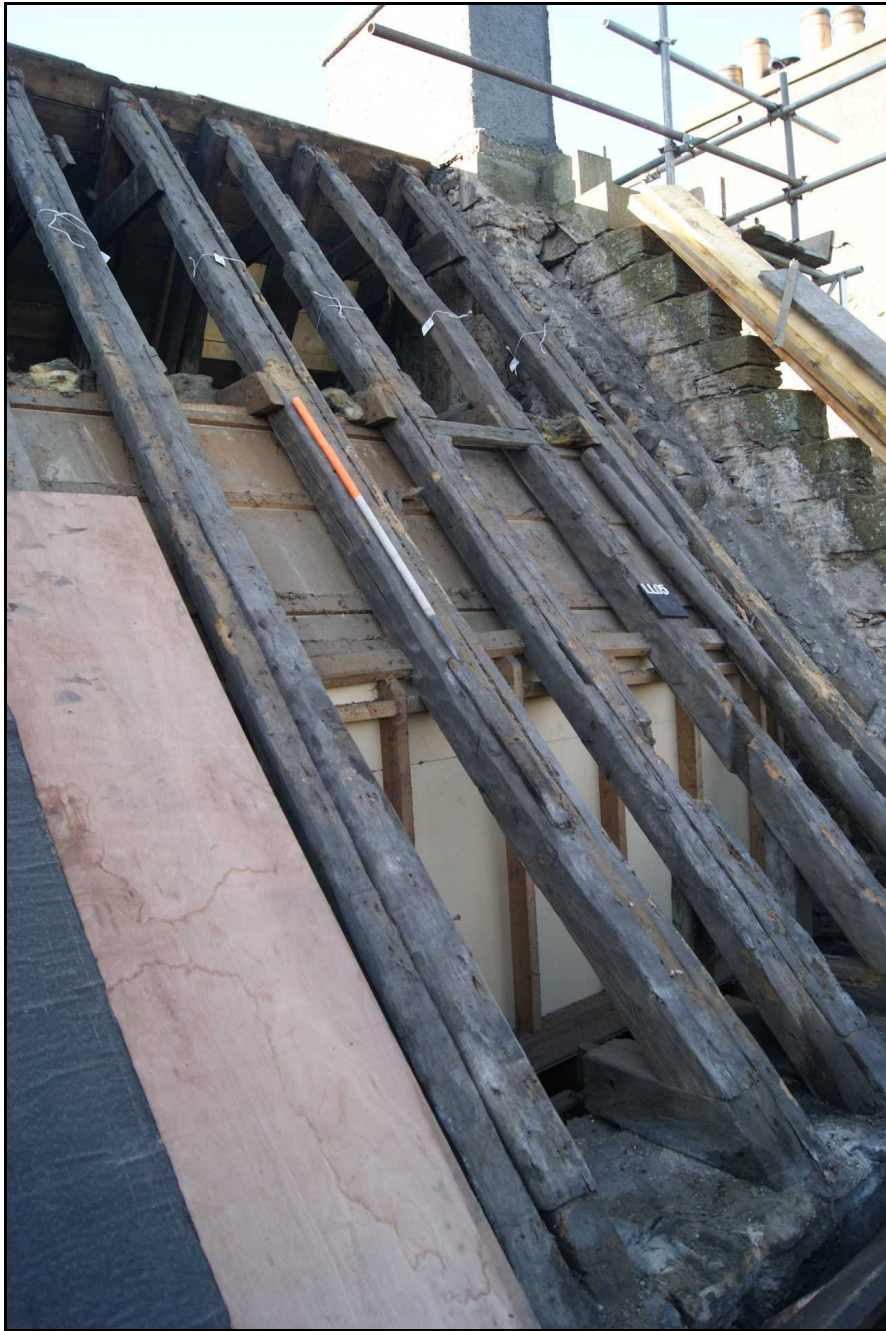
Photo of rafters, N pitch of the N roof
