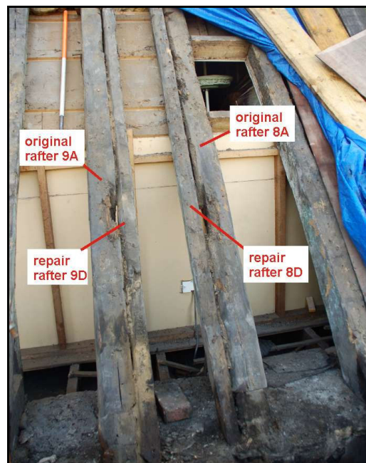
Photo showing some of the repairs to the N roof
