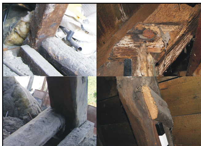
Photos showing the differences between widths of collars between the N and S roofs. The N roof collars (whole) are shown on the left whilst the narrow S roof collar stubs are shown on the right
