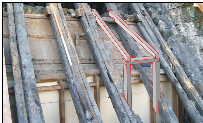
Reconstruction of cat slide (rafters 2A & 3A)
