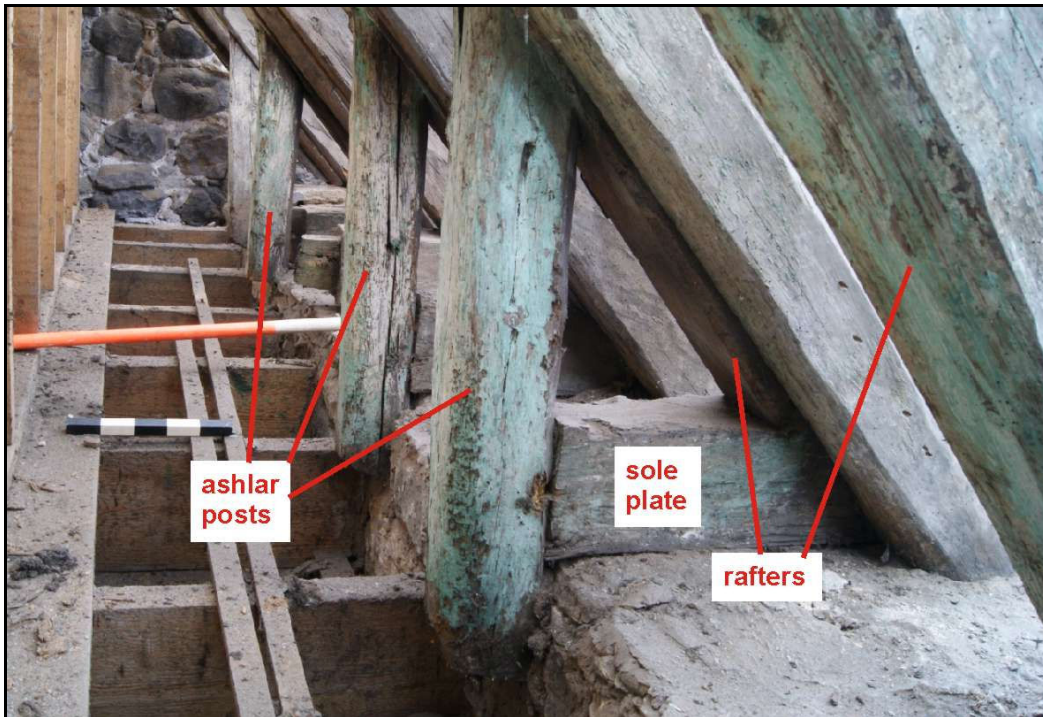
Photo showing ashlar posts and sole plates at the N wall
