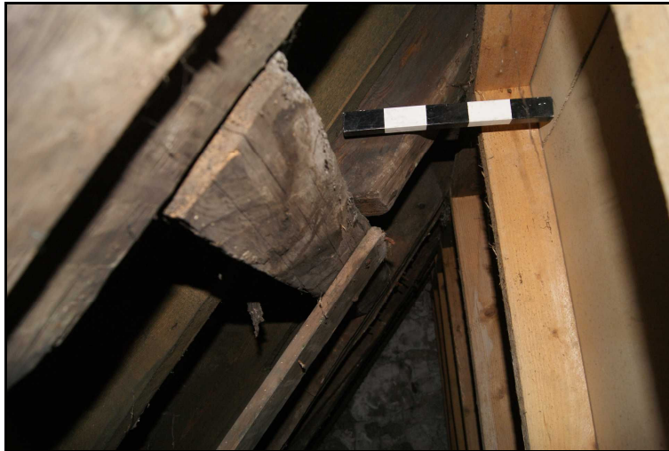
Photo of bridle 28 on the E side of the S roof
