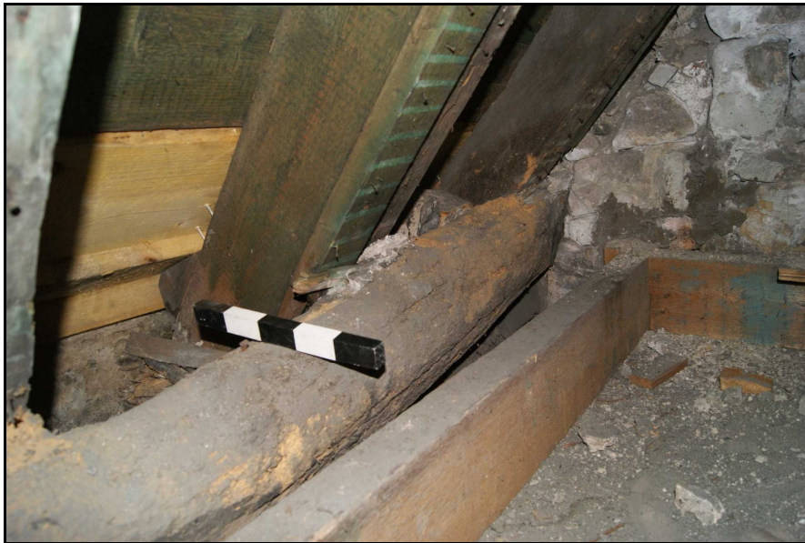
Photo showing beam 26 with 27 below
