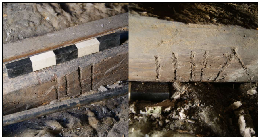
Photos of assembly marks in the N roof
