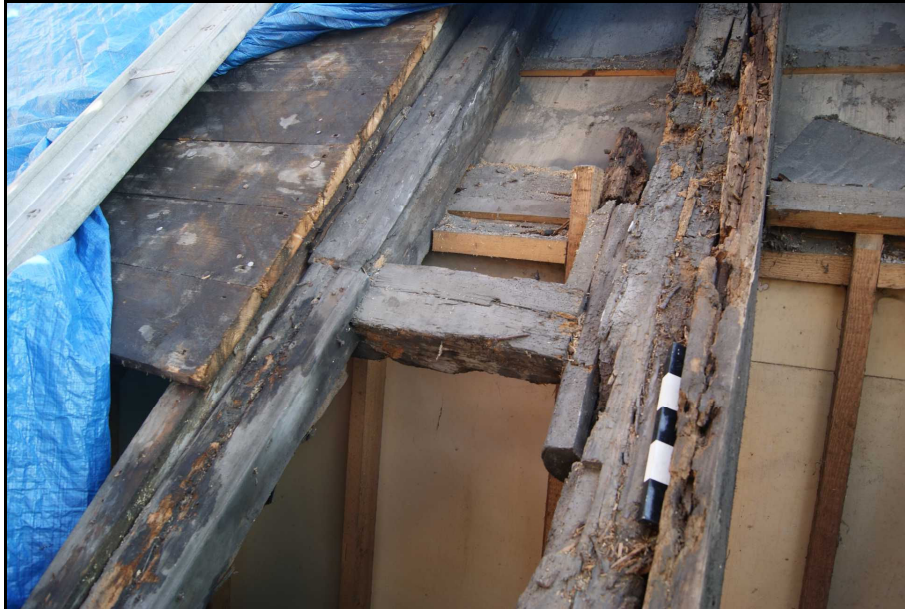
Photo of bridle 36 on the W side of the S roof
