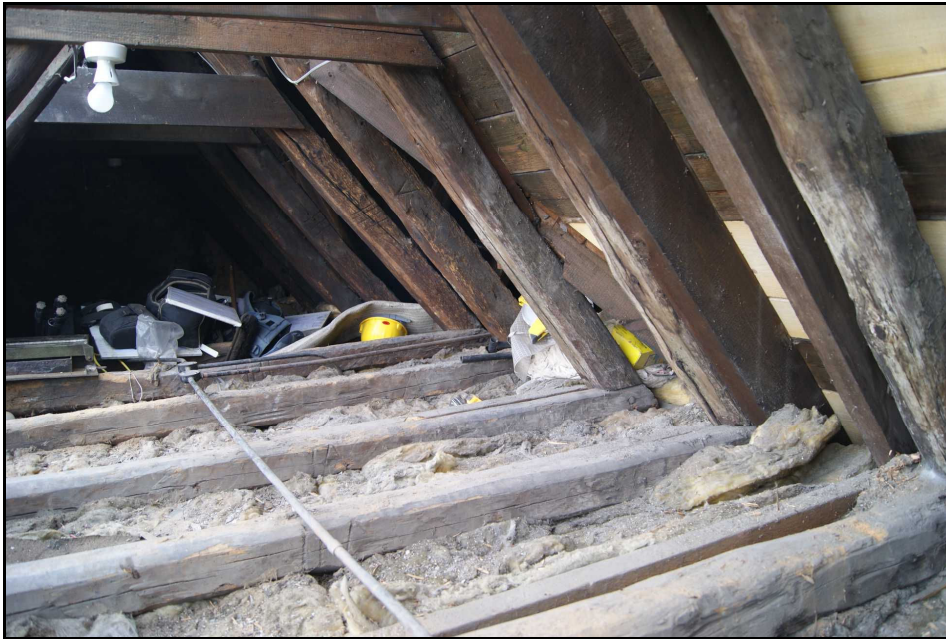
Photo showing collars of the N roof
