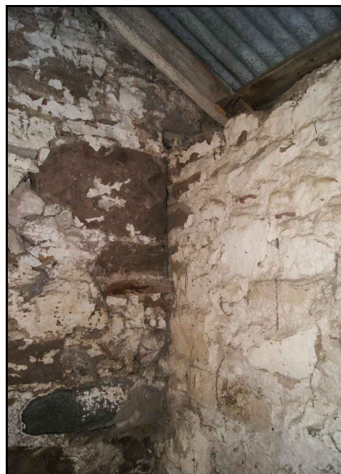
Shot showing where the E wall of the Barn has been built around the N wall of the Cart Shed
