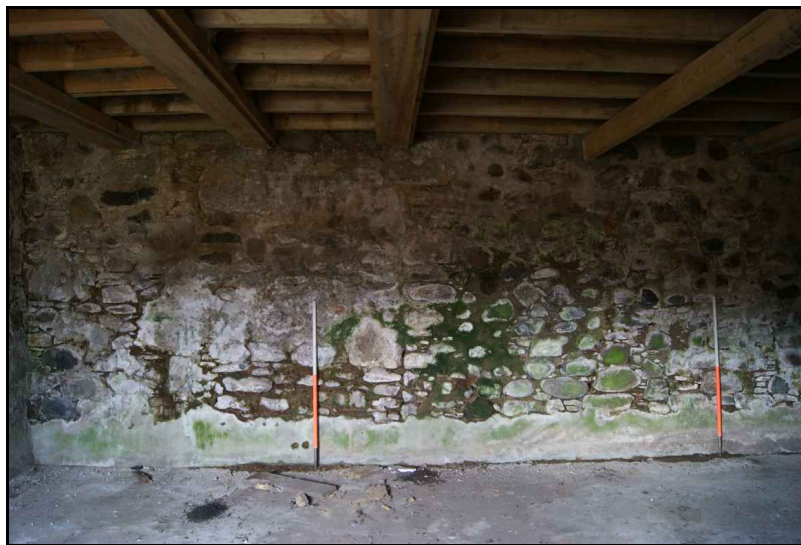
The blocked doorway in the W wall of the Mill, ground floor
