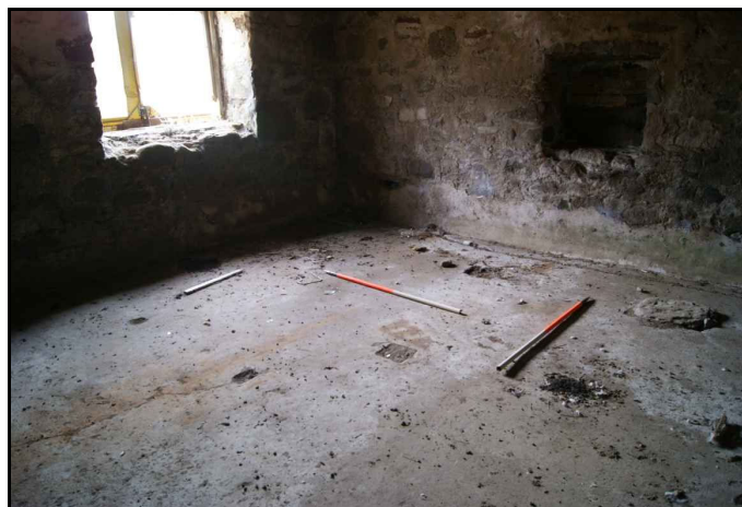
Shot showing holes and plinth in concrete floor for grinding equipment/cogs
