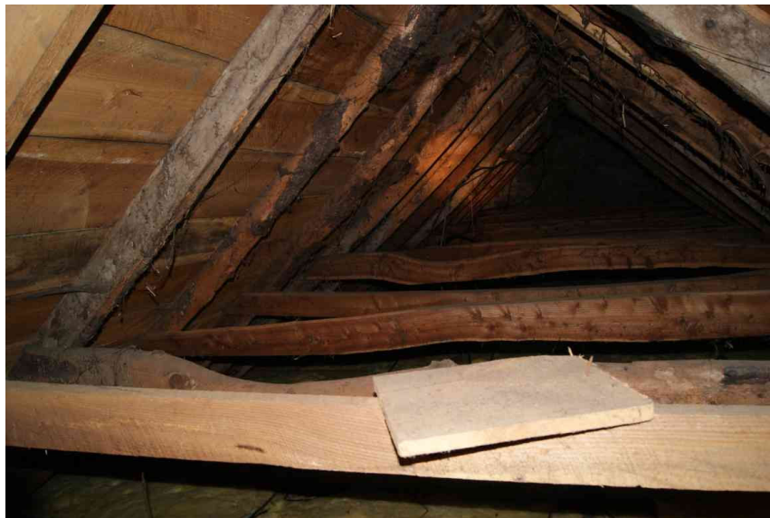
The roof in the E part of the cottage showing irregularly shaped collars
