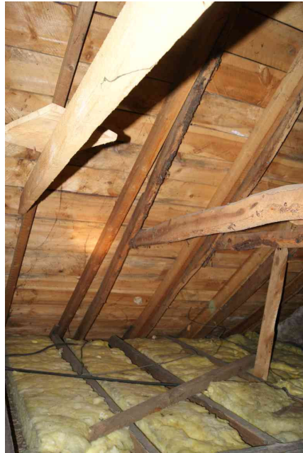
Shot showing floor joists, original rafters and later rafter replacements
