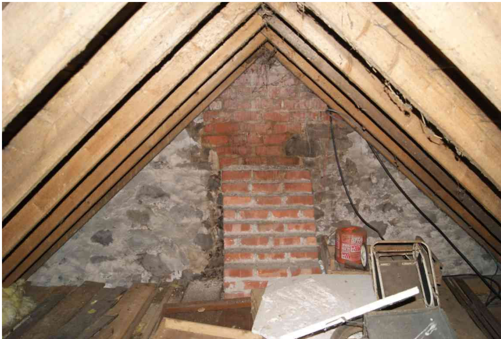
The E gable above Bedroom 1 showing the red brick chimney stack
