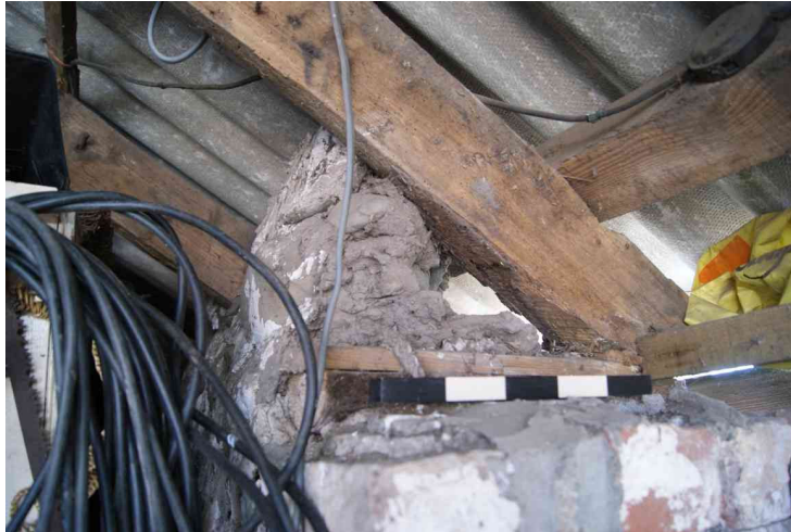
Clay fill on the top of the S wall
