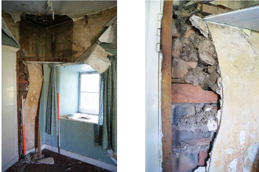
The corner cupboard and bricks with clay bonding next to the extension doorway
