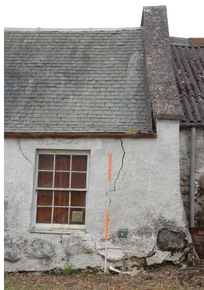
Shot showing foundation stones low down in the N wall
