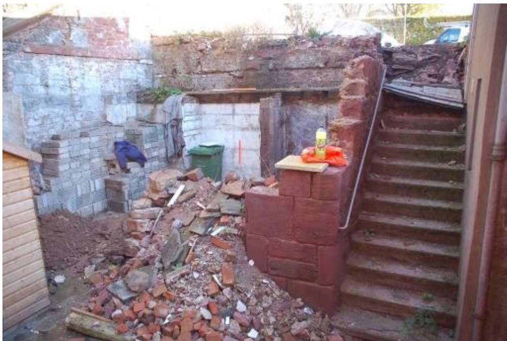
Working on lower area of site
