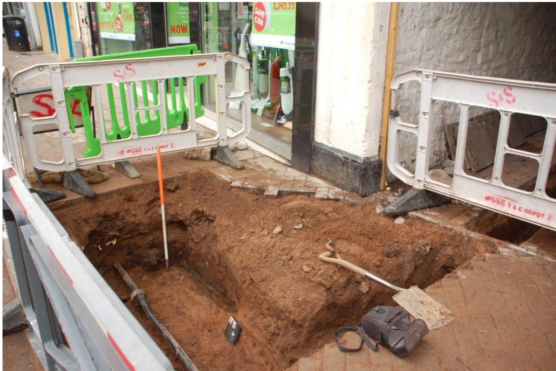
Location of 'T joint' in Castle Street, showing ditch feature
