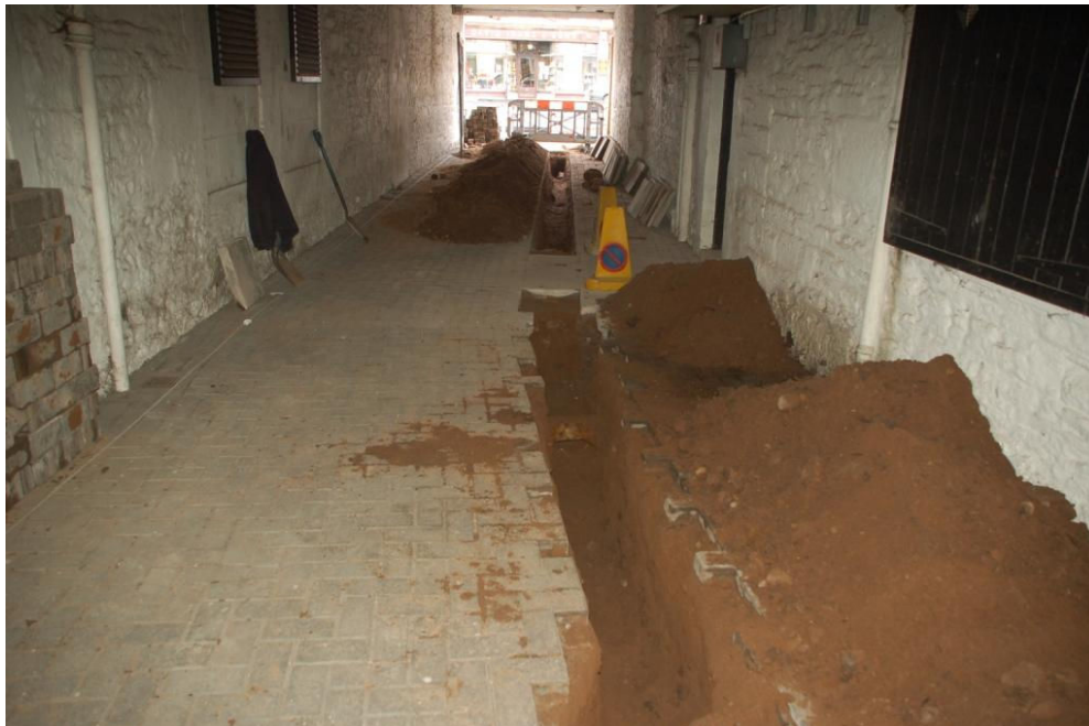
Excavated cable trench in pend
