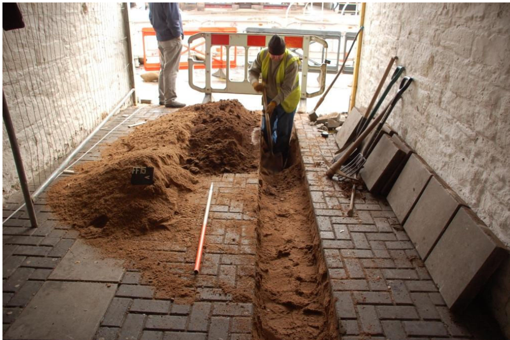
Starting excavation of cable trench in pend
