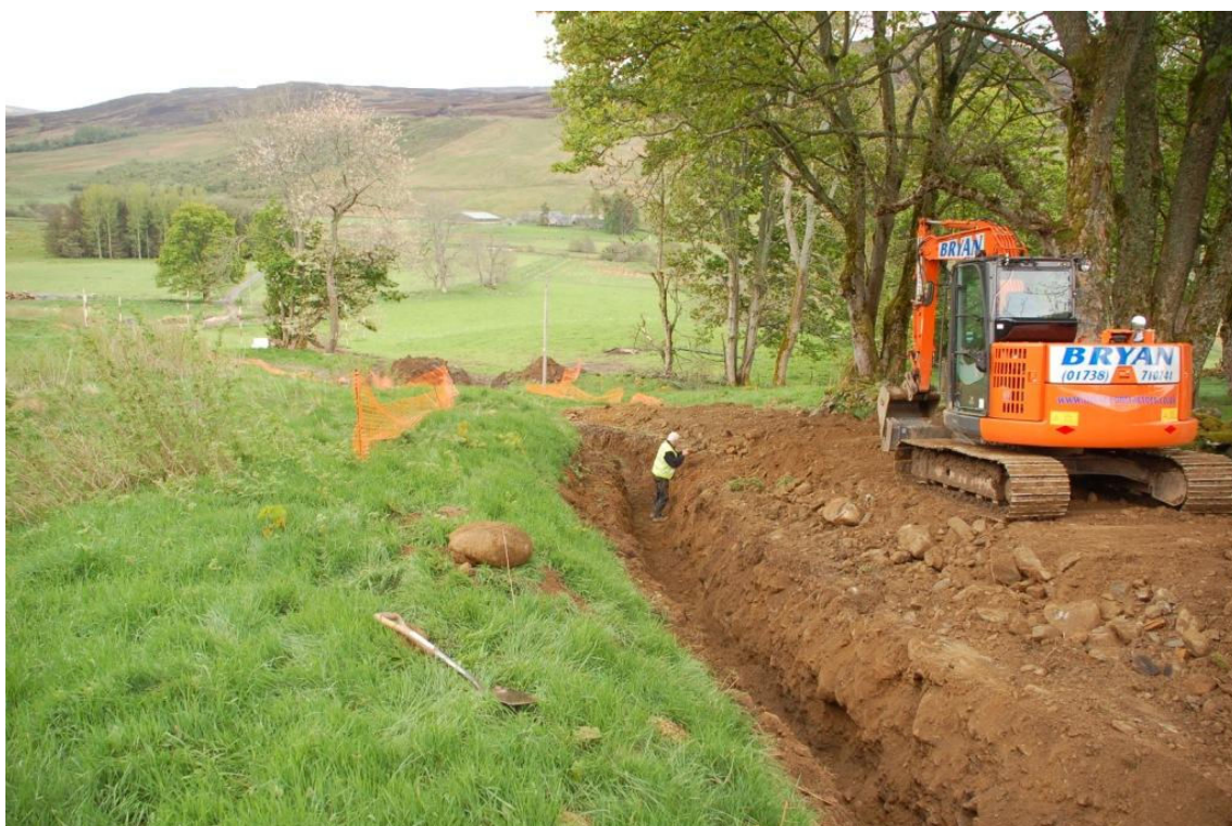
Pipe trench cut into drainage ditch
