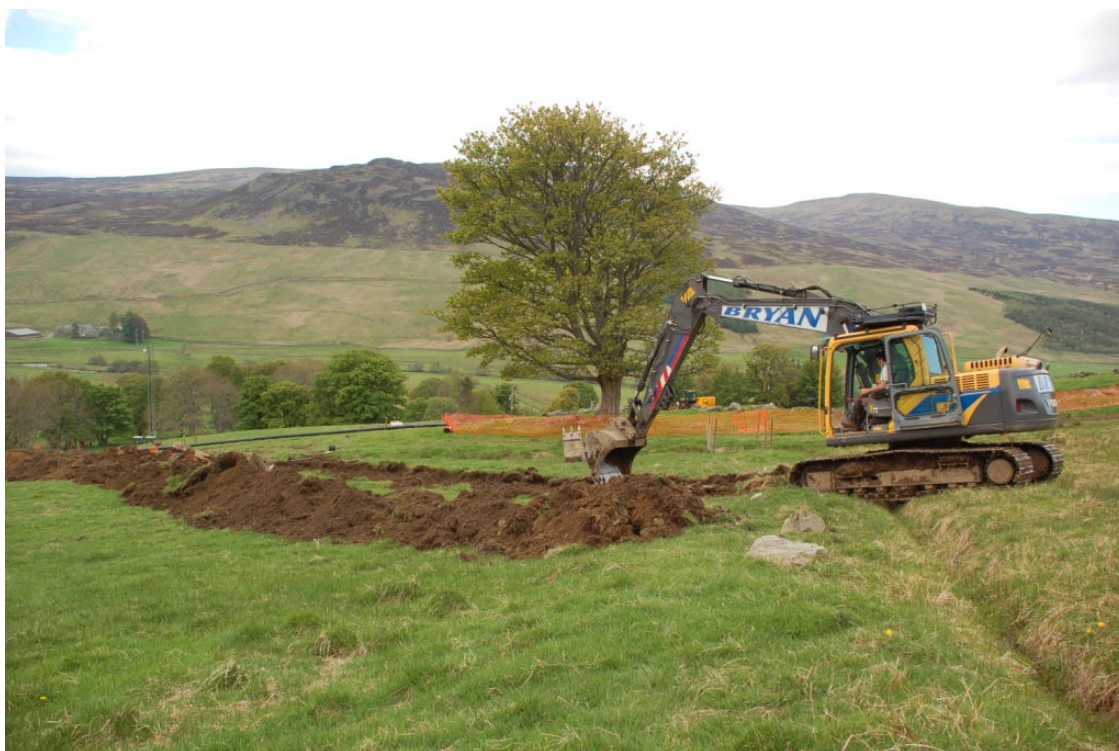
Pipe trench on E side of farmstead site
