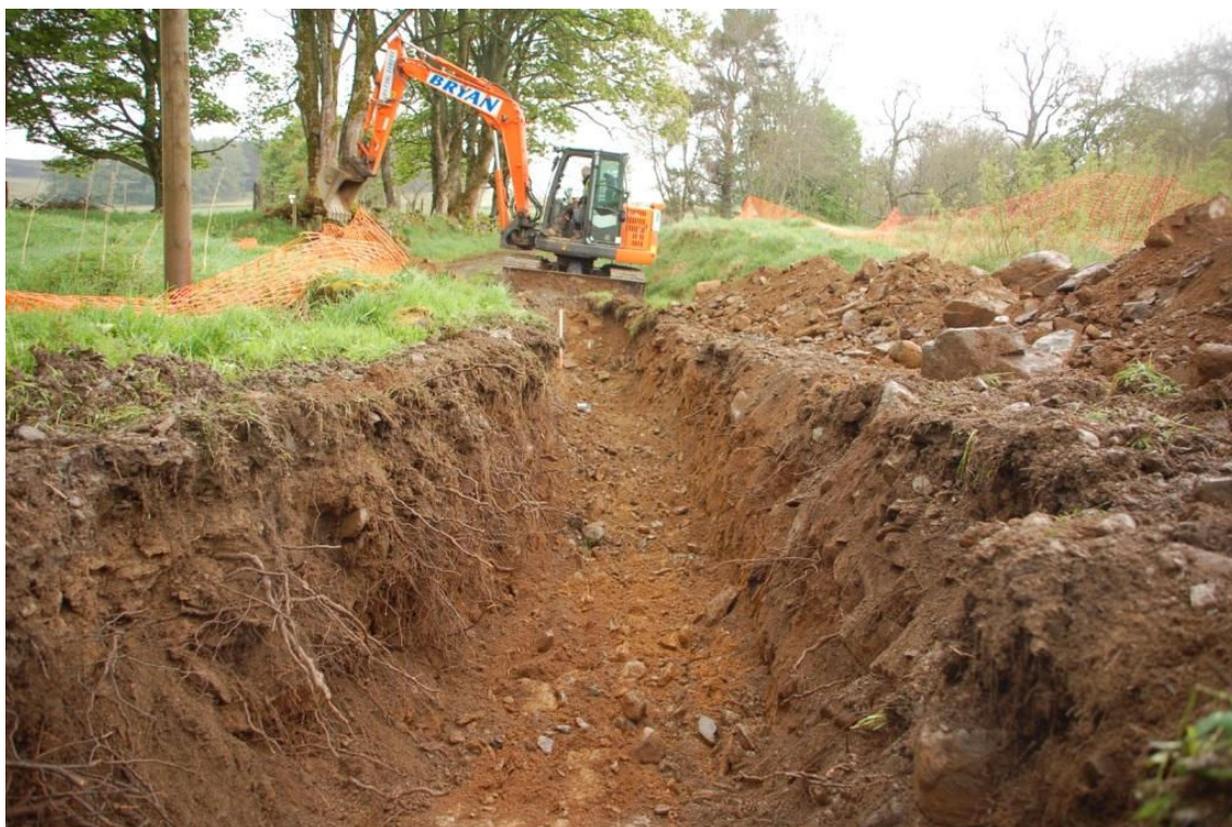
Pipe trench crossing road
