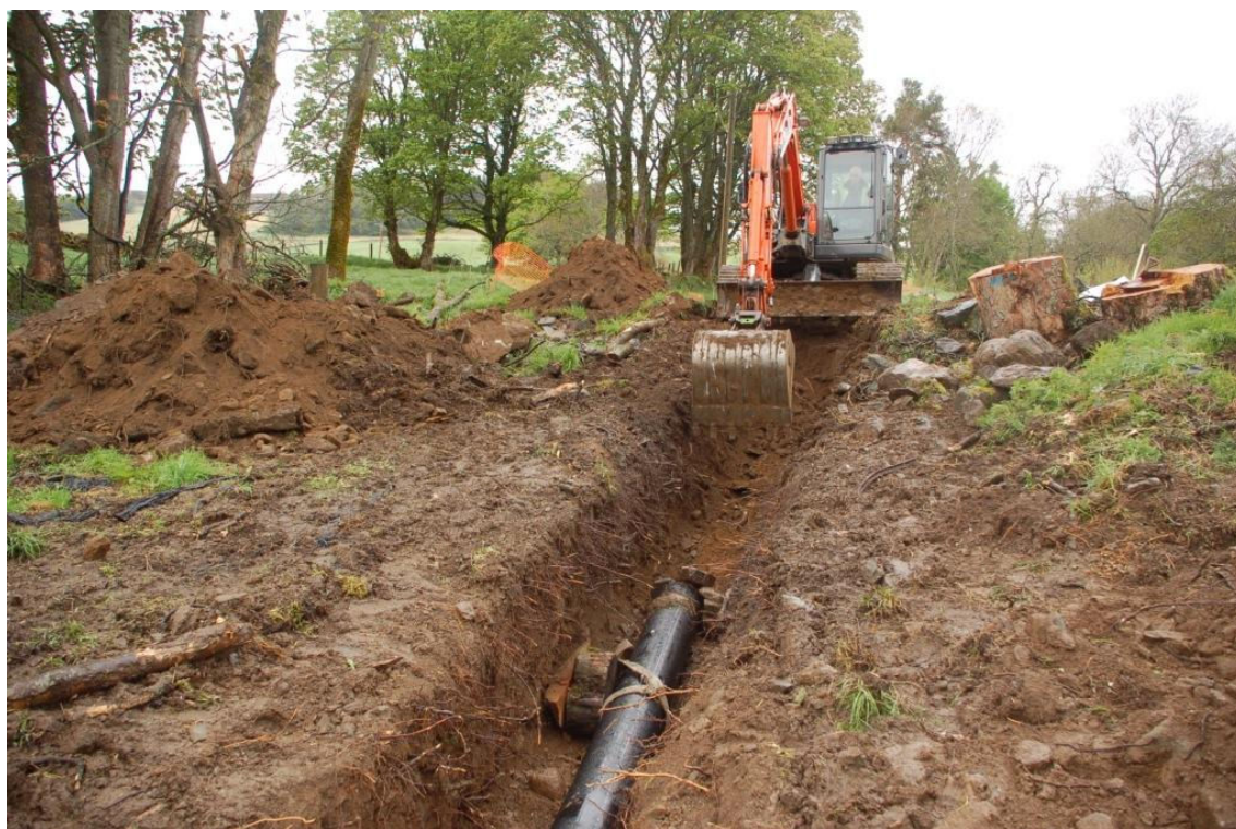
Pipe trench crossing field boundary
