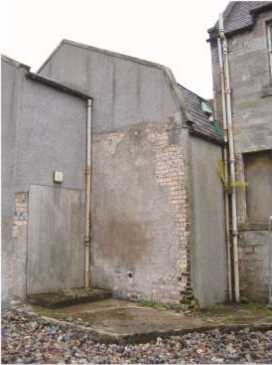
Image 037 SE corner with 'Dutch barn' roof.
