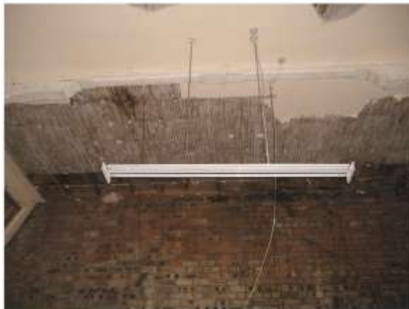
Image 027 North roof truss partly masked by later ceiling
