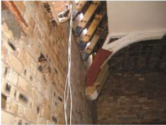
Image 011 South roof truss and corbels
