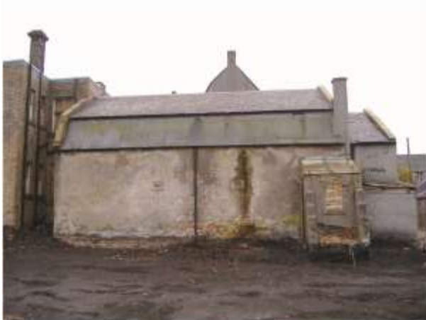
Image 042 West elevation with ventilators and roof truss bolts.
