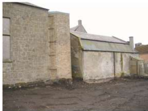
Image 050 NW corner with adjacent buildings.
