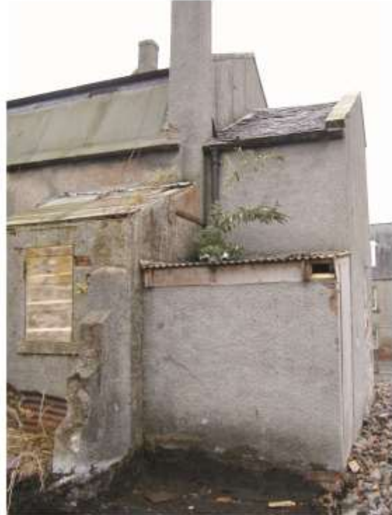
Image 040 SW corner with toilet annexe and chimney.
