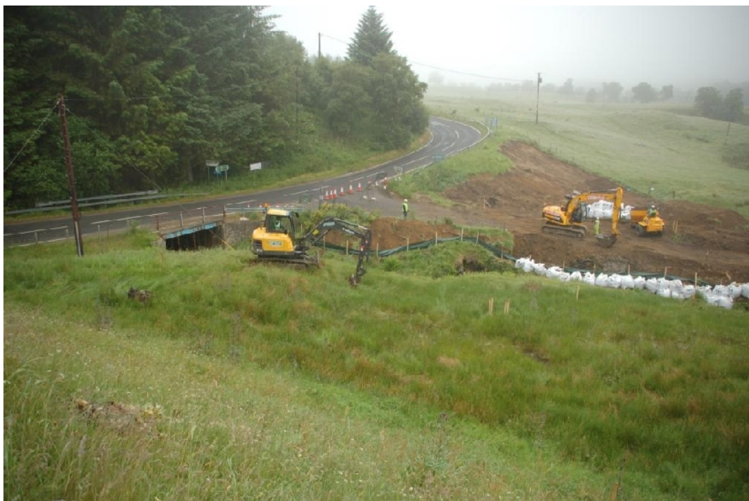
BL02_159: General groundworks over Allt an Lair, view N.
