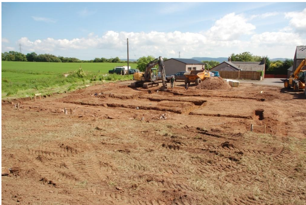
LF05_058 House foundation trenches view SE
