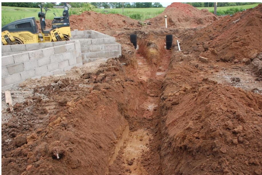
LF05_226 Drainage trenches and inspection chambers on house plot, view NE
