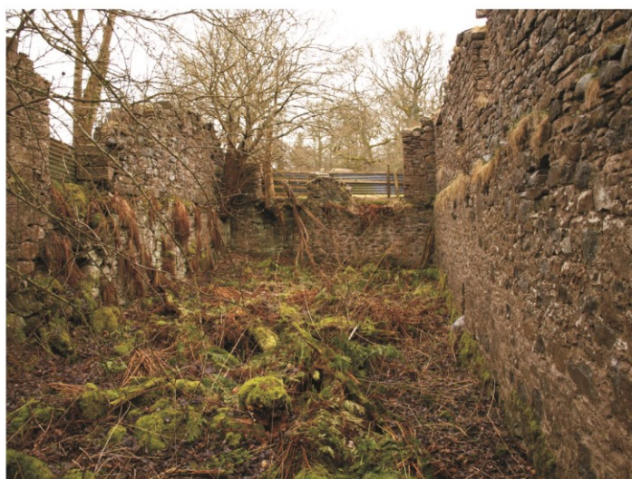
Illus 8 Mill House 02 interior. W Wall 03 ahead. Pit 23 and Wall 11 under vegetation in foreground. Wall 04 to R with Scarcement 10 and Putlogs 15 - 20 below.
