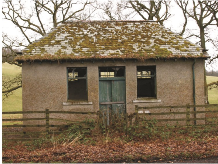
Illus 12 Water Treatment House 34 from road.
