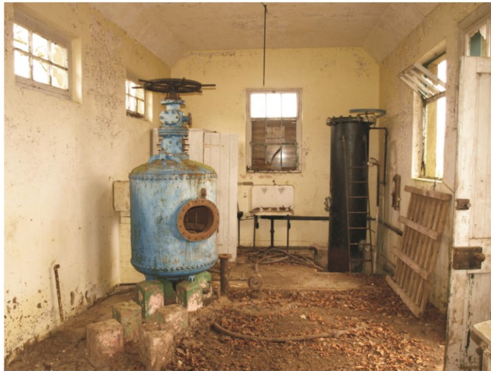
Illus 13 Water Treatment House 34 interior. Machine 38.
