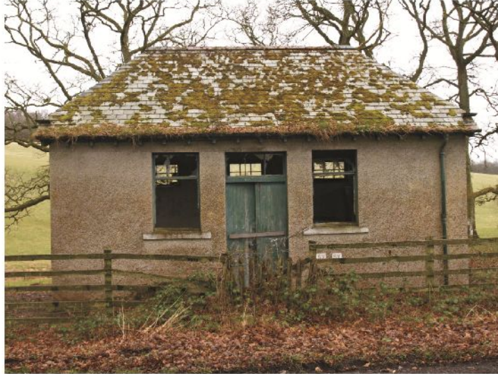
Illus 12 Water Treatment House 34 from road.
