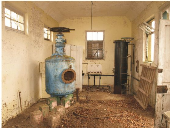
Illus 13 Water Treatment House 34 interior. Machine 38.
